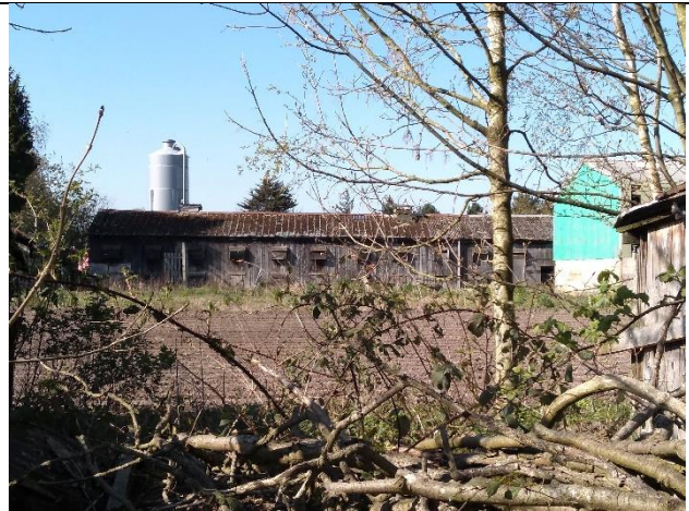
TN14 – Farm building associated with Rose Farm (April 2019)
