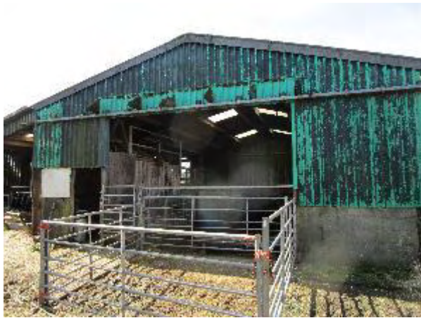
Eastern elevation of Building 9
