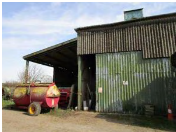
North western elevation of Building 11
