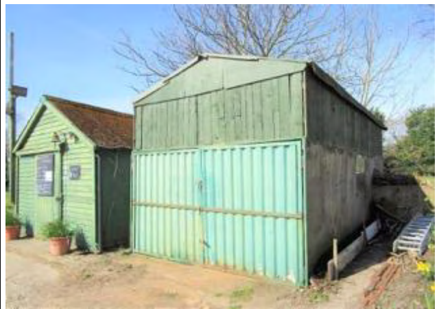
South eastern elevation of Building 4
