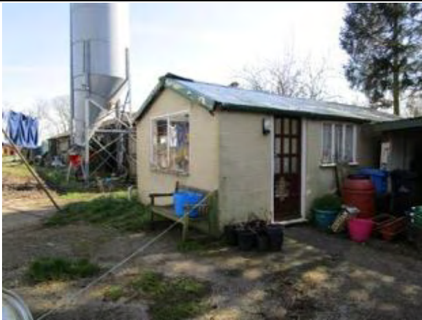
The northern and western elevations of Building 7
