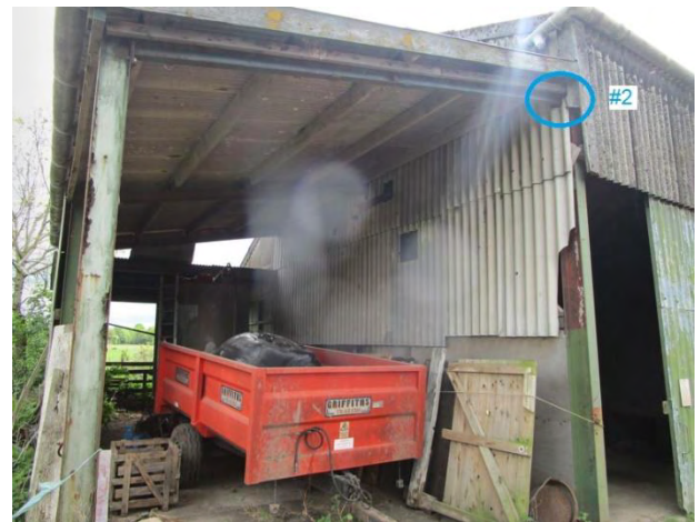
North western elevation of Building 11 noting roost #2
