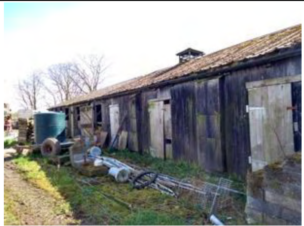
Northern elevation of Building 8
