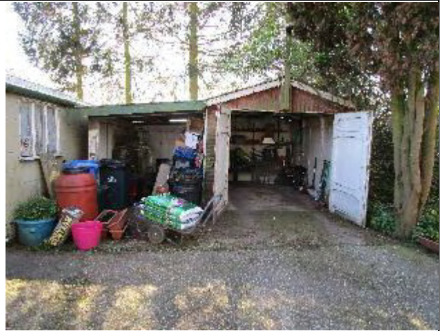
Northern elevation of Building 6
