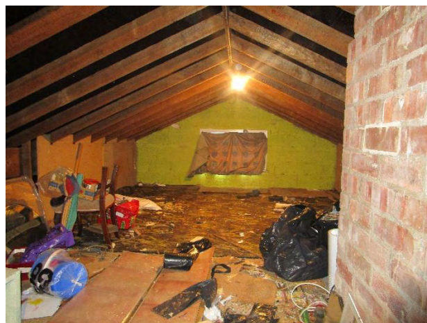
Internal loft area of Building 1
