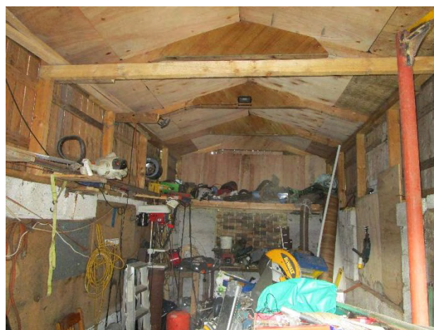
Internal area of Building 4
