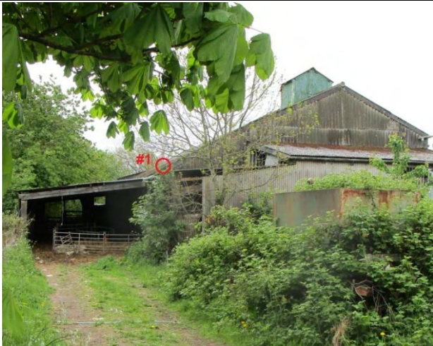
North eastern elevation of Building 11 noting roost #1
