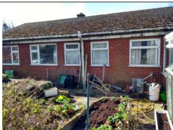
Eastern elevation of Building 1
