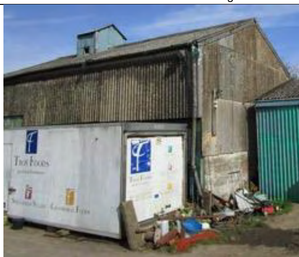
South western elevation of Building 11
