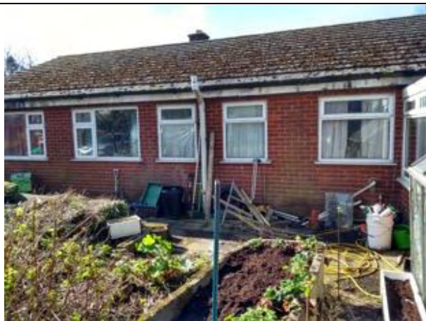
Eastern elevation of Building 1
