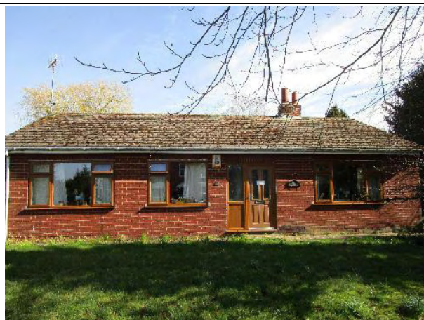
Western elevation of Building 2
