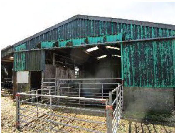
Eastern elevation of Building 9
