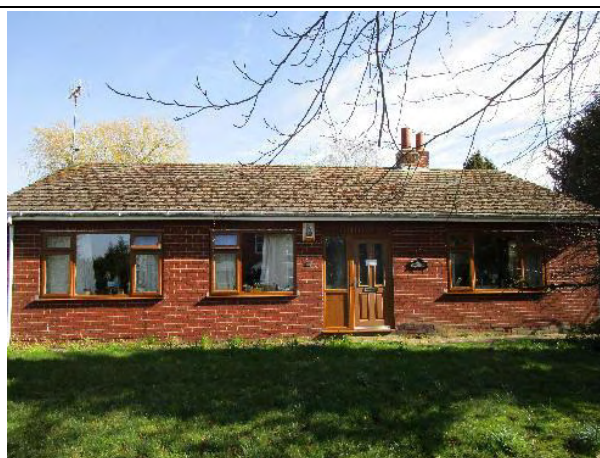
Western elevation of Building 2
