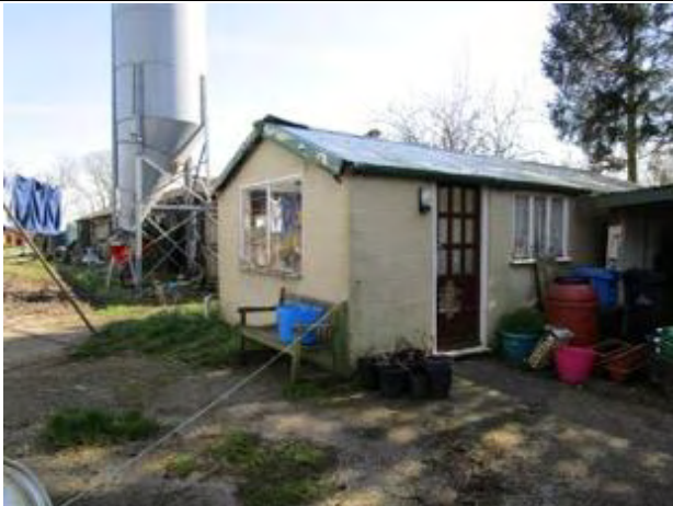
The northern and western elevations of Building 7
