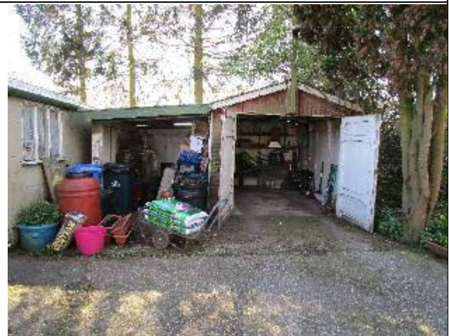
Northern elevation of Building 6
