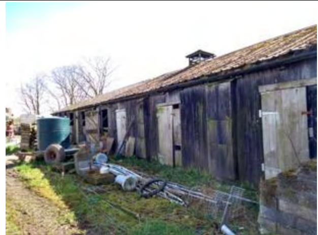
Northern elevation of Building 8
