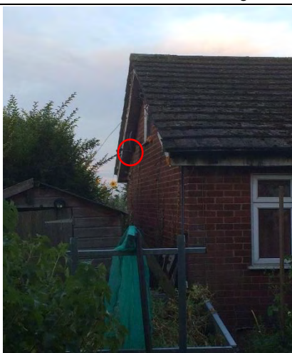
Roost location on the south eastern elevation of Building 1.
