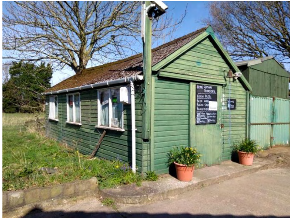
South western elevation of Building 3
