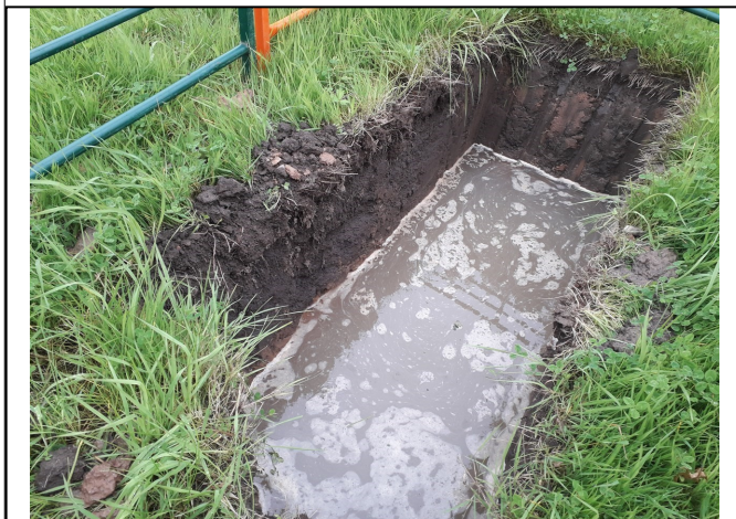
Trial Pit 106/ Soakaway 104
