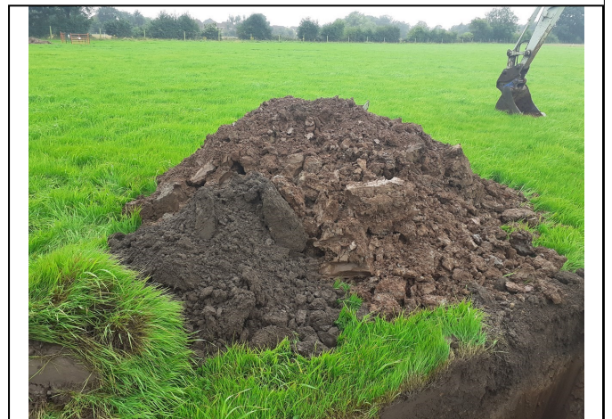
Trial Pit 126 Spoil
