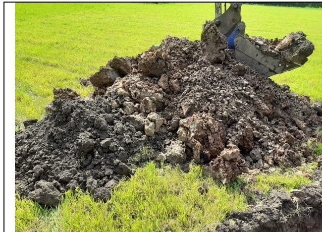
Trial Pit 113 Spoil
