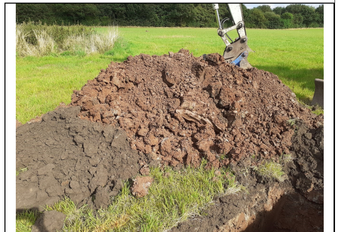
Trial Pit 118 Spoil
