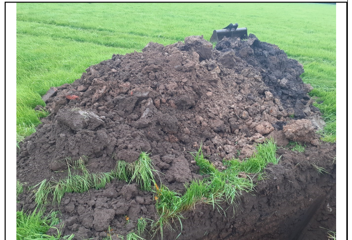
Trial Pit 121 Spoil
