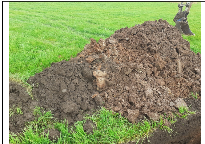
Trial Pit 124 Spoil
