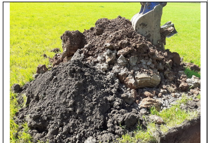
Trial Pit 114 Spoil
