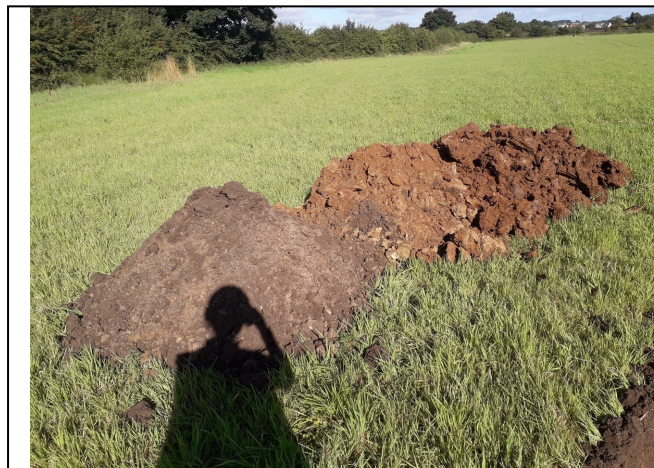
Trial Pit 102 Spoil
