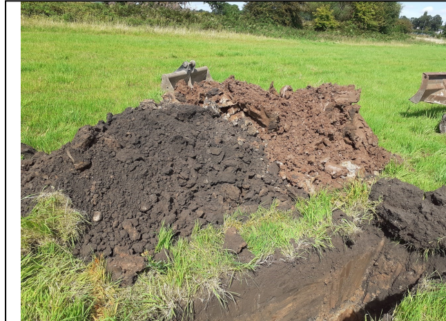
Trial Pit 112 Spoil
