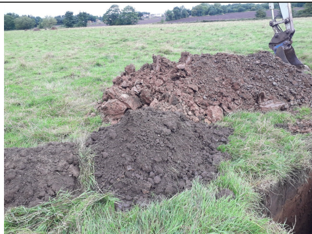
Trial Pit 129 Spoil
