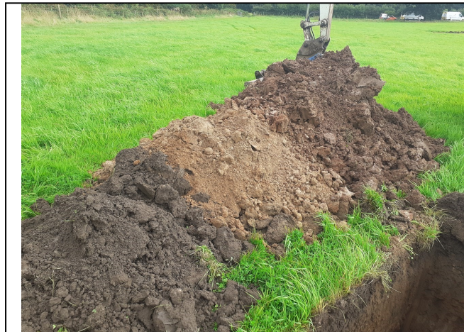
Trial Pit 123 Spoil
