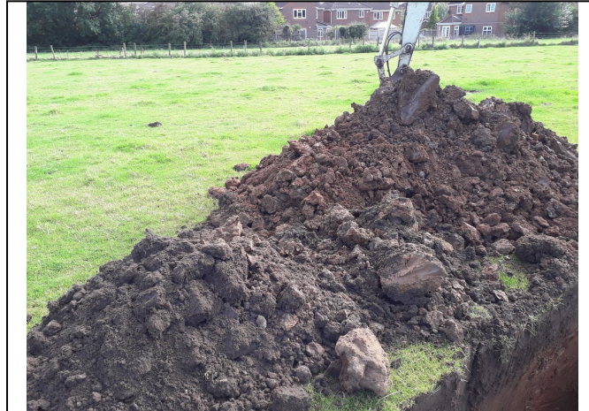
Trial Pit 142 Spoil
