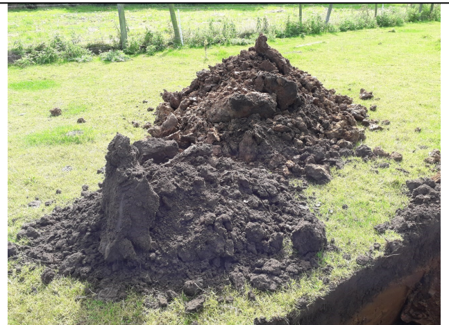
Trial Pit 141 Spoil
