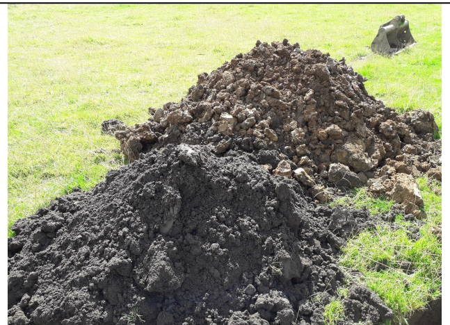
Trial Pit 139 Spoil
