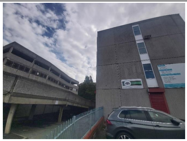
Western and northern aspect of building and adjacent multi-storey car park.
