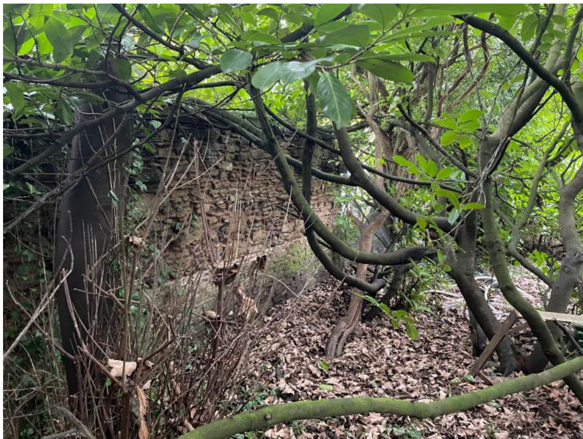
Photo 9: South Side of High Wall in Garden
