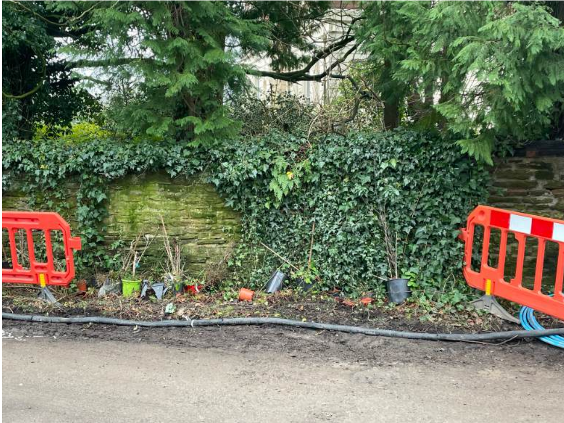
Photo 3: North Side of Wall
