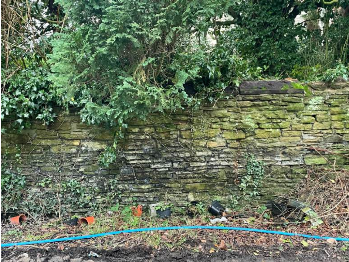
Photo 5: North Side of Wall
