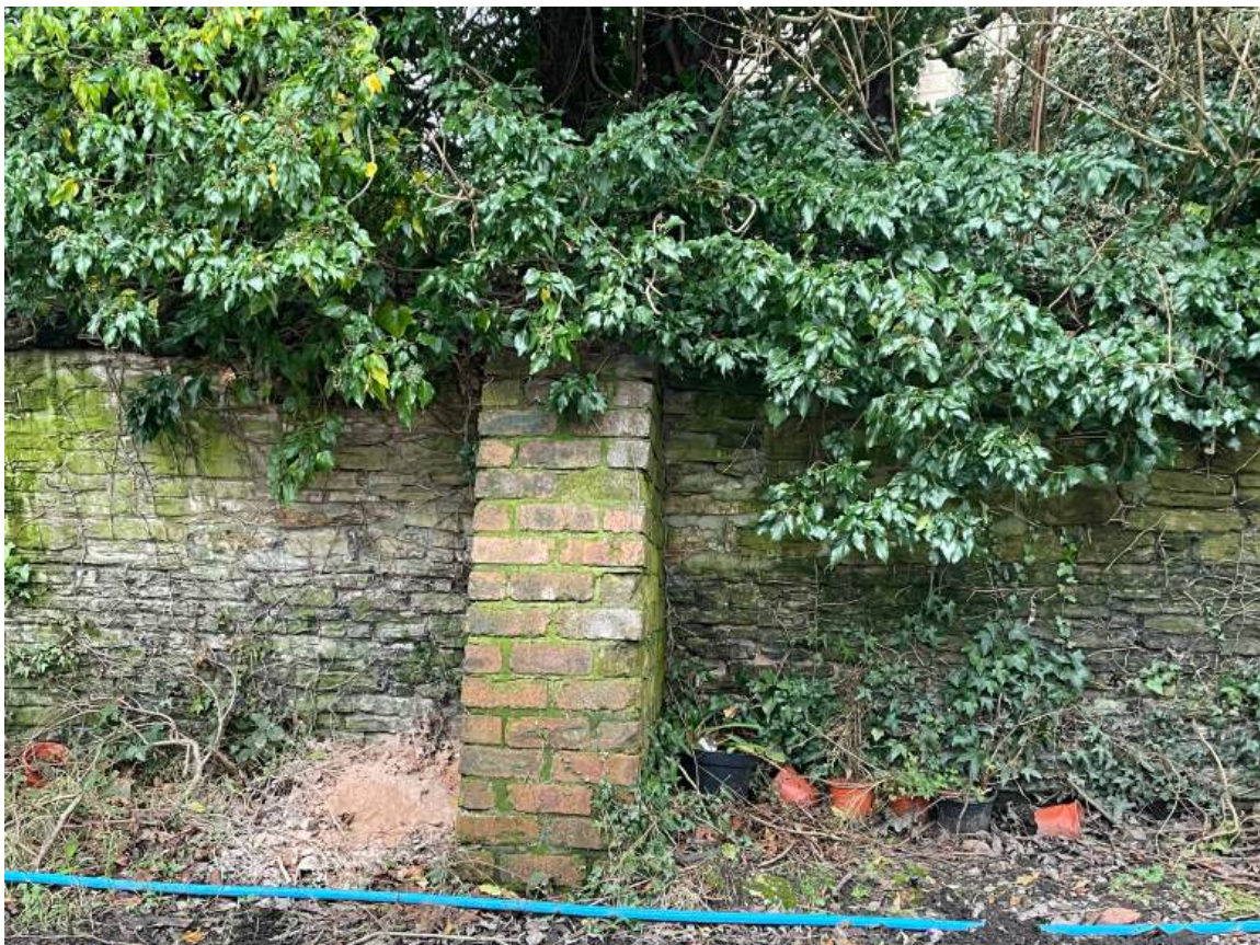
Photo 6: North Side of Wall
