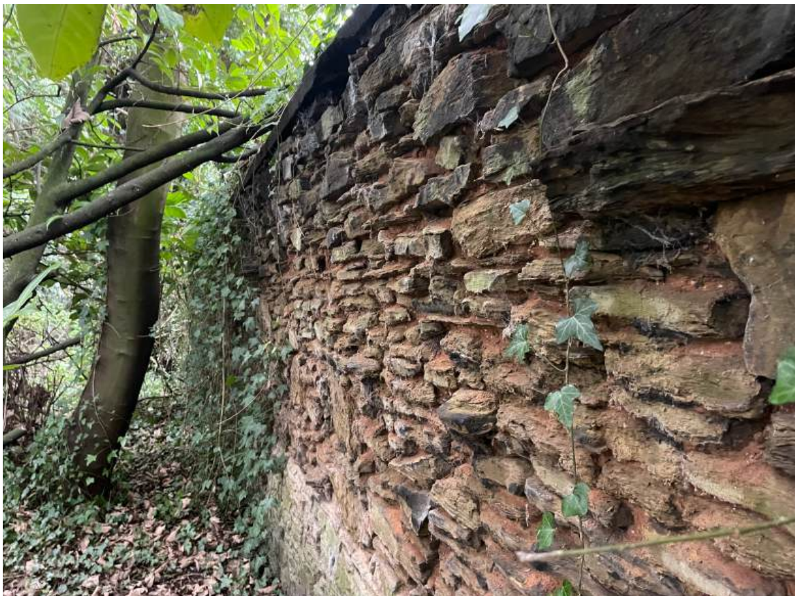
Photo 8: South Side of High Wall in Garden
