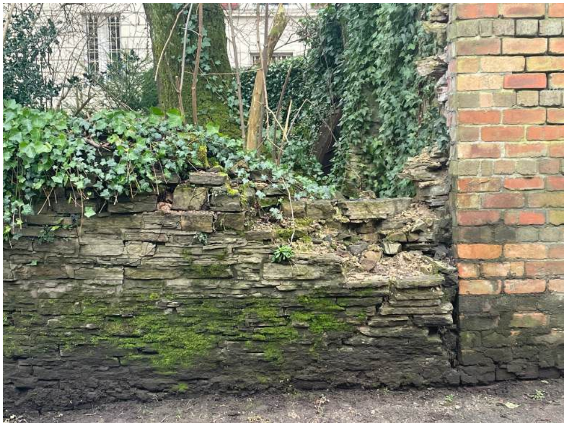
Photo 1: West End of Wall
