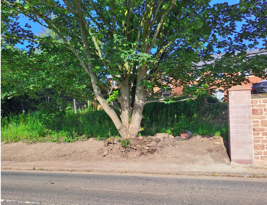
Photo 3: View west following removal of old boundary wall (new wall right of frame)
