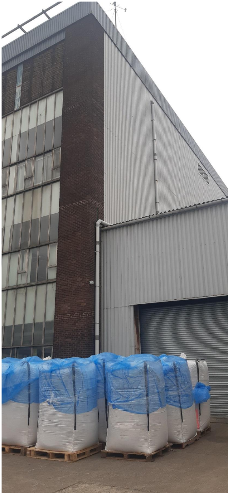
Photo 2: Building to the left to be demolished; building to the right to be retained.
