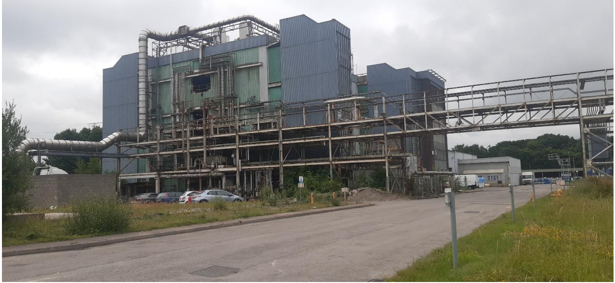
Photo 3: Building in the foreground to be demolished; building to the right to be retained.
