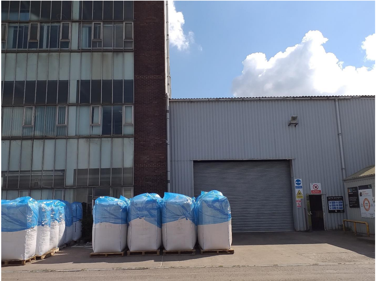
Photo 1: Building to the left to be demolished; building to the right to be retained.
