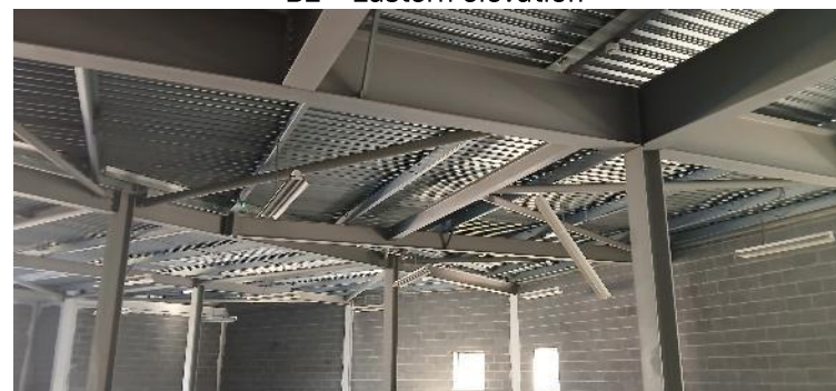
Interior of B2
