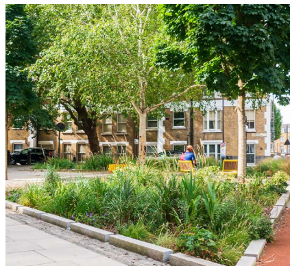
Figure 1.11: Rain garden (Image credit: GreenBlue Urban)
