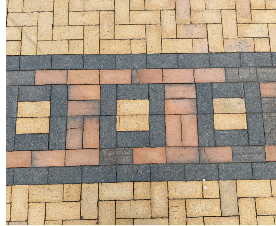
Figure 2.41: Surface treatment to Derby Road
