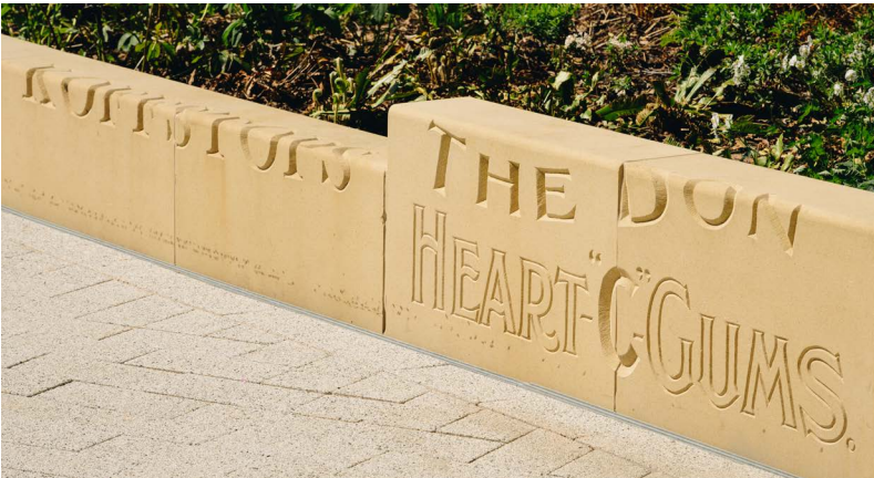
Engraved & Cast-in Lettering: Examples of lettering details
