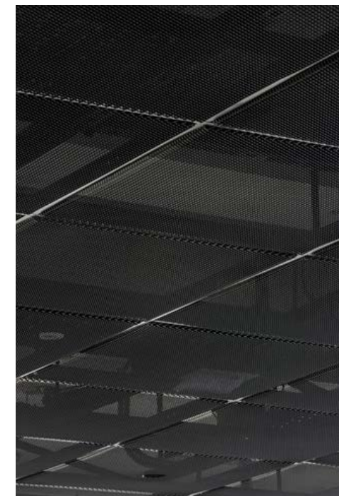
Metal mesh ceiling and exposed services
