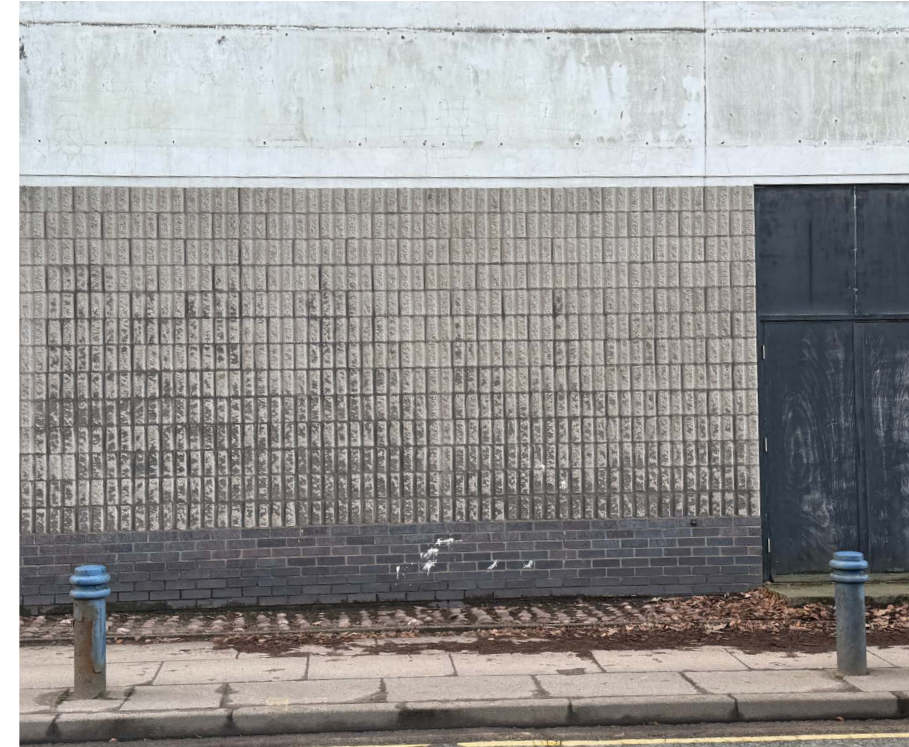
Figure 2.21: Lathom Road Multi-storey as seen from Lathom Road
