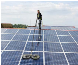
PV Cleaning - Water fed pole
