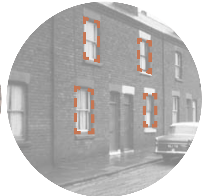
Staggered window arrangement
