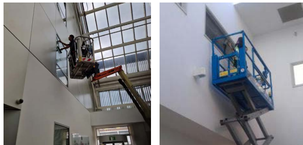
Temporary MEWP cleaning and access internally
