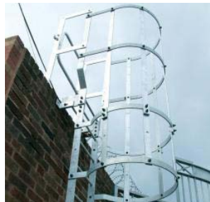
CAT ladder roof access with PPC finish to match light bronze cladding (Level 05 to 06)
