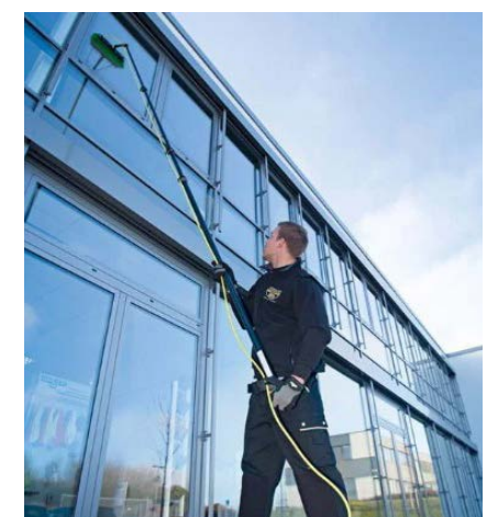
Facade Cleaning via reach & wash / water fed pole
