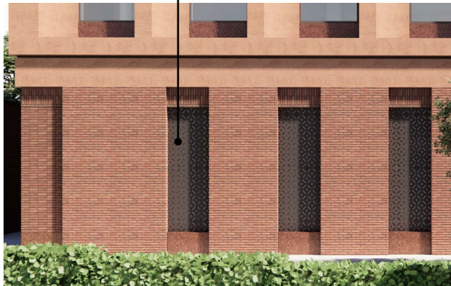
Cladding visualisation: Perforated metal feature patterning
