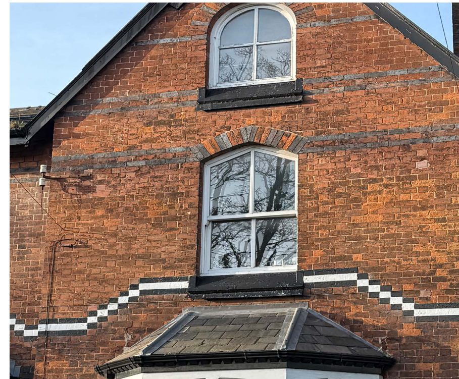
Figure 2.23: Brickwork banding and lintels to houses in the area
