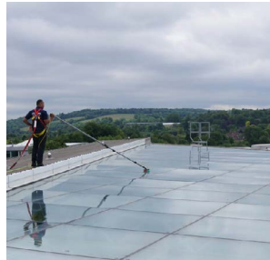
Water fed pole rooflights cleaning
