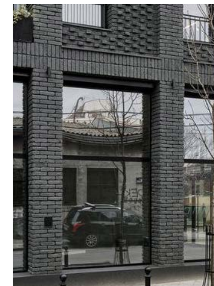
Large street level openings with piers
