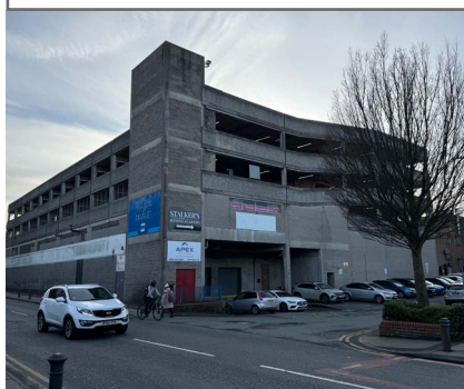
Multi-Storey Car Park
