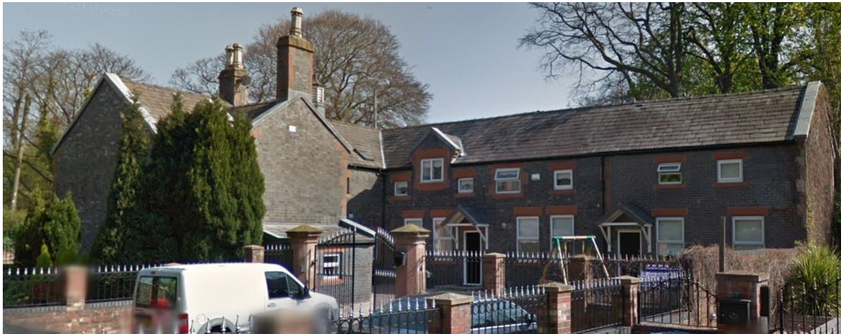
Courtyard view of existing building
