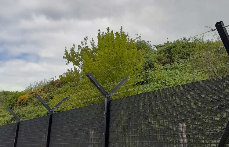
Proposed example paladin fencing [PPC Black] with 'Y' cranked angle bracket and barbed wires above (orange line)
