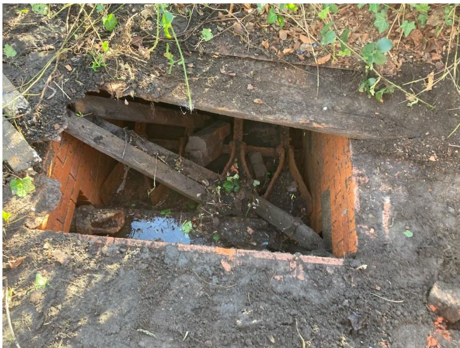
Photograph 4: View of septic tank.
