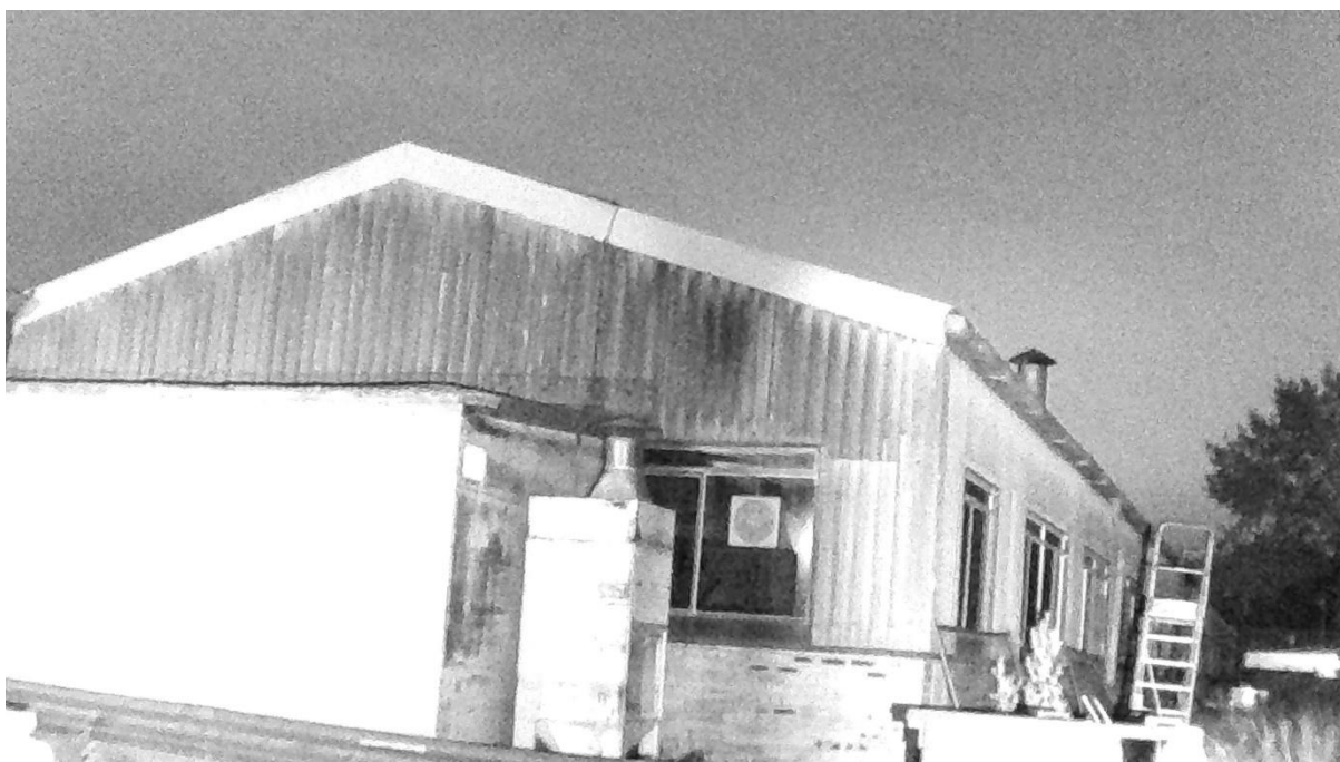
Photograph 1 – Infrared image taken of the western aspect of Building 3 at the darkest point of the survey at 21:51 on 23 rd August 2025.
