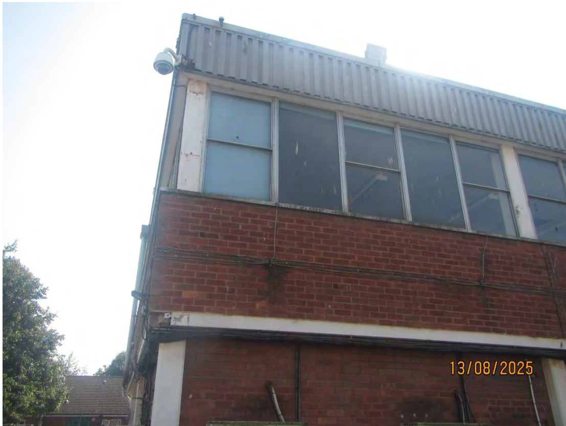
Photograph 11 – Showing the external structure of Building 2, including the cladding, redbrick walls and windows.
