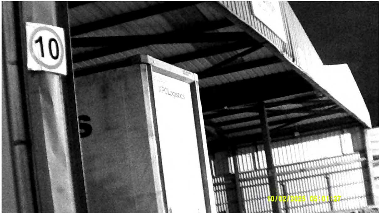
Photograph 25 – Infrared image taken of the northeastern aspect of Building 1 at the darkest point of the survey at 05:01 on 2 nd October 2025.
