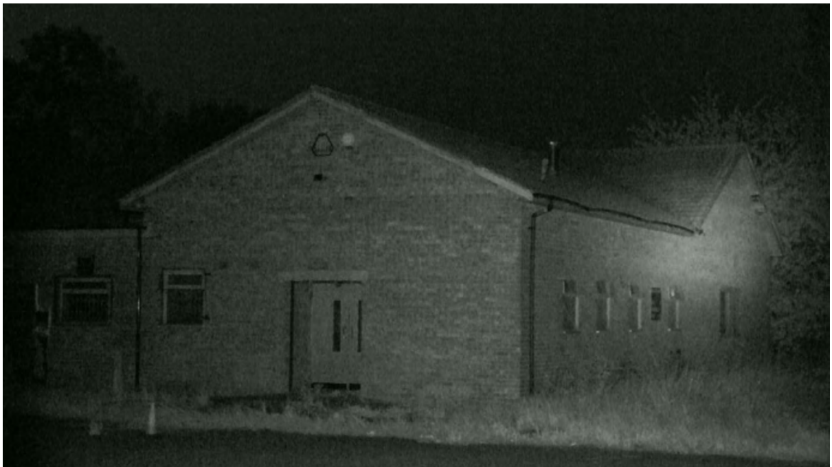
Photograph 4— Infrared image taken of the northwestern aspect of Building 7 at the darkest point of the survey at on.
