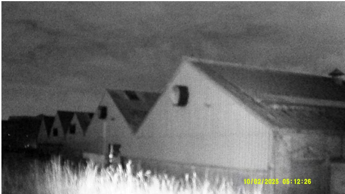
Photograph 21 – Infrared image taken of the northeastern aspect of Building 1 at the darkest point of the survey at 05:12 on 2 nd October 2025.
