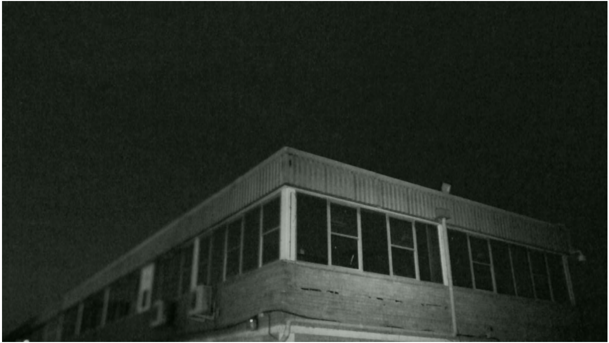
Photograph 3— Infrared image taken of the northwestern aspect of Building 2 at the darkest point of the survey at 21:30 on 23 rd August 2025.
