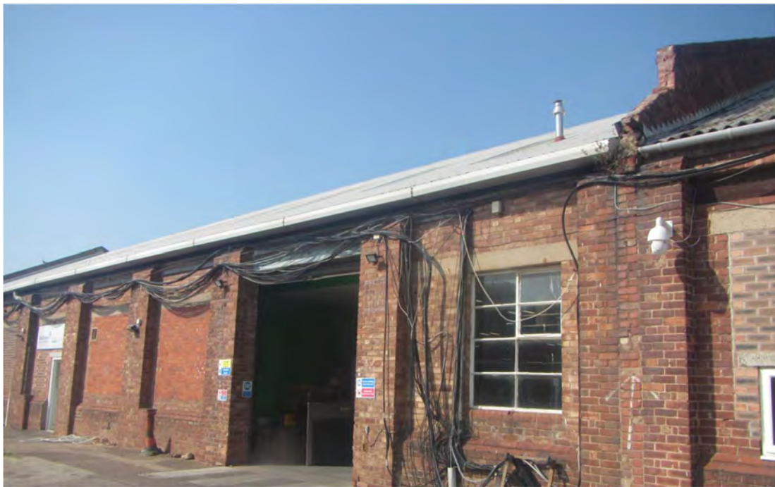
Photograph 4 – Sheet metal roof on Building 1.
