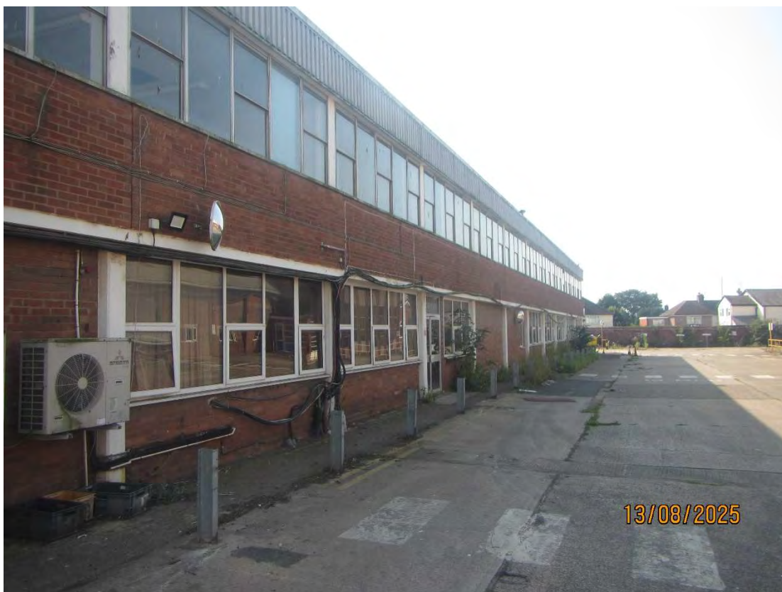
Photograph 10 – The northern aspect of Building 2.
