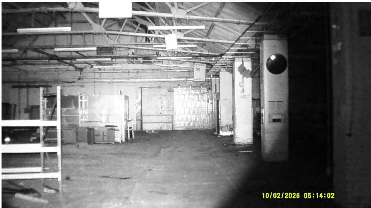
Photograph 20 – Infrared image taken of the western interior of Building 1 at the darkest point of the survey at 05:14 on 2 nd October 2025.
