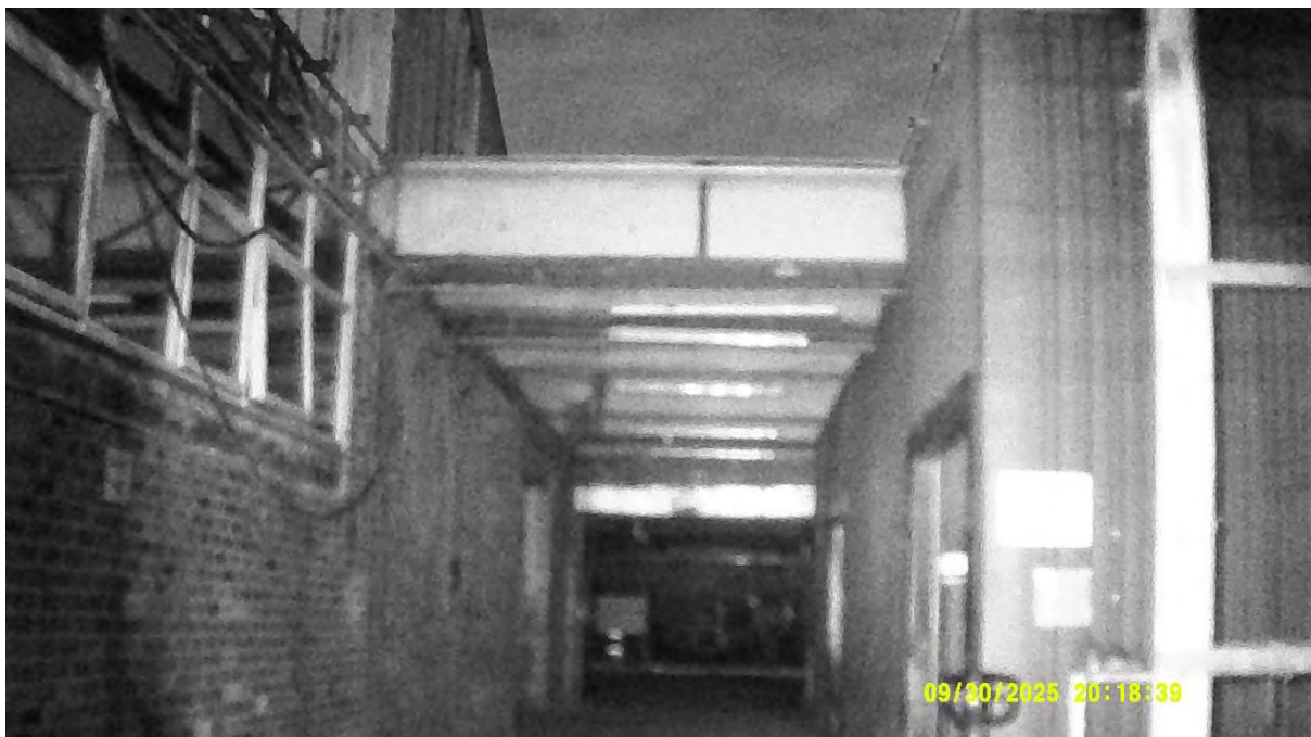
Photograph 18 – Infrared image taken of the northern aspect of Building 1 at the darkest point of the survey at 20:18 on 30 th September 2025.
