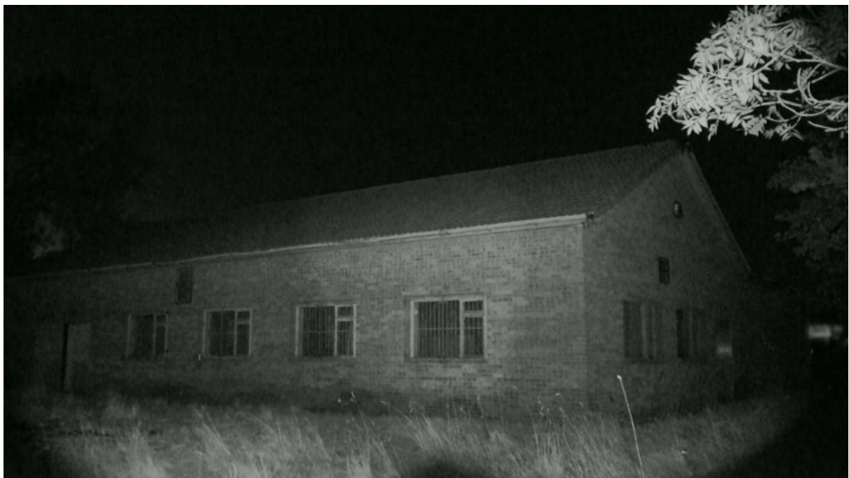
Photograph 14 – Infrared image taken of the southern aspect of Building 7 at the darkest point of the survey at 20:32 on 25 th September 2025.
