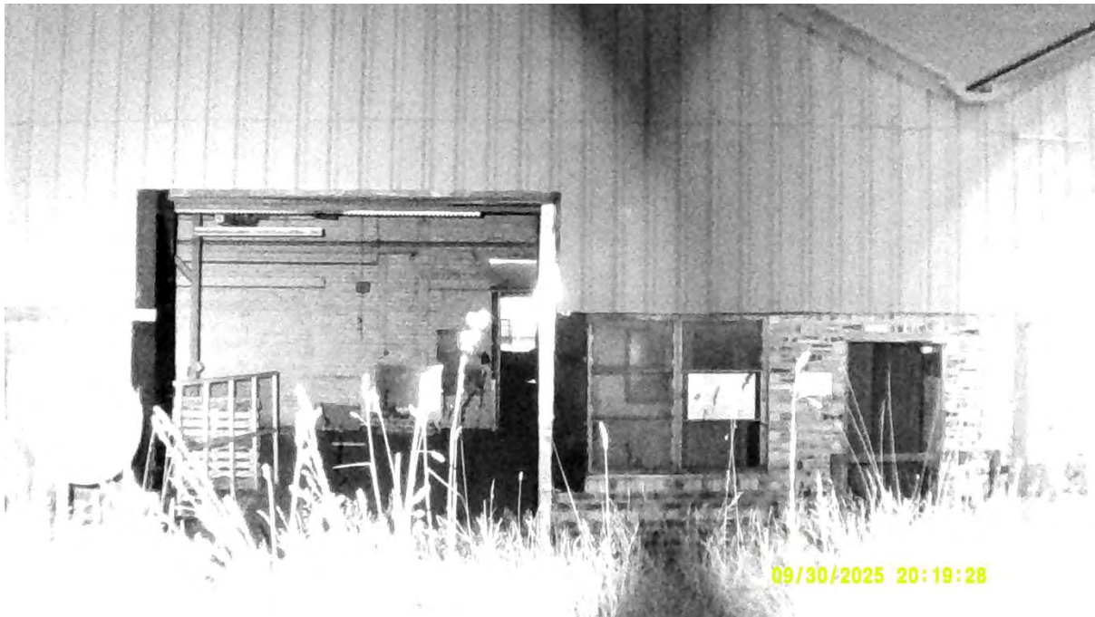
Photograph 17 – Infrared image taken of the northeastern aspect of Building 1 at the darkest point of the survey at 20:19 on 30 th September 2025.
