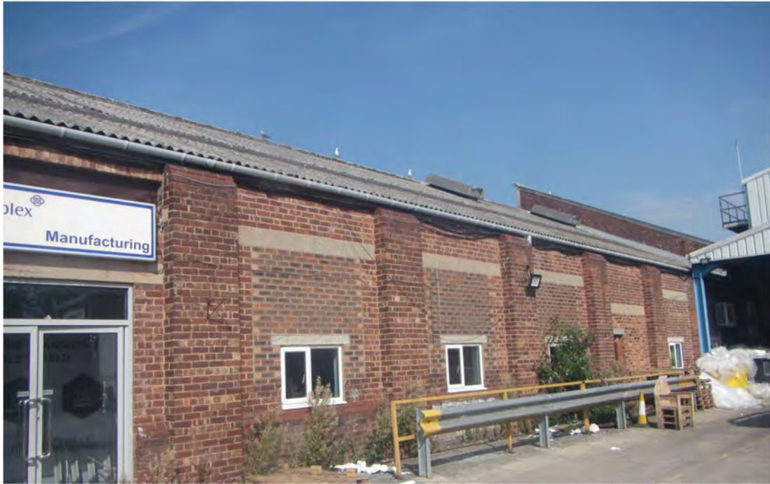
Photograph 3 – Corrugated asbestos roof on Building 1.
