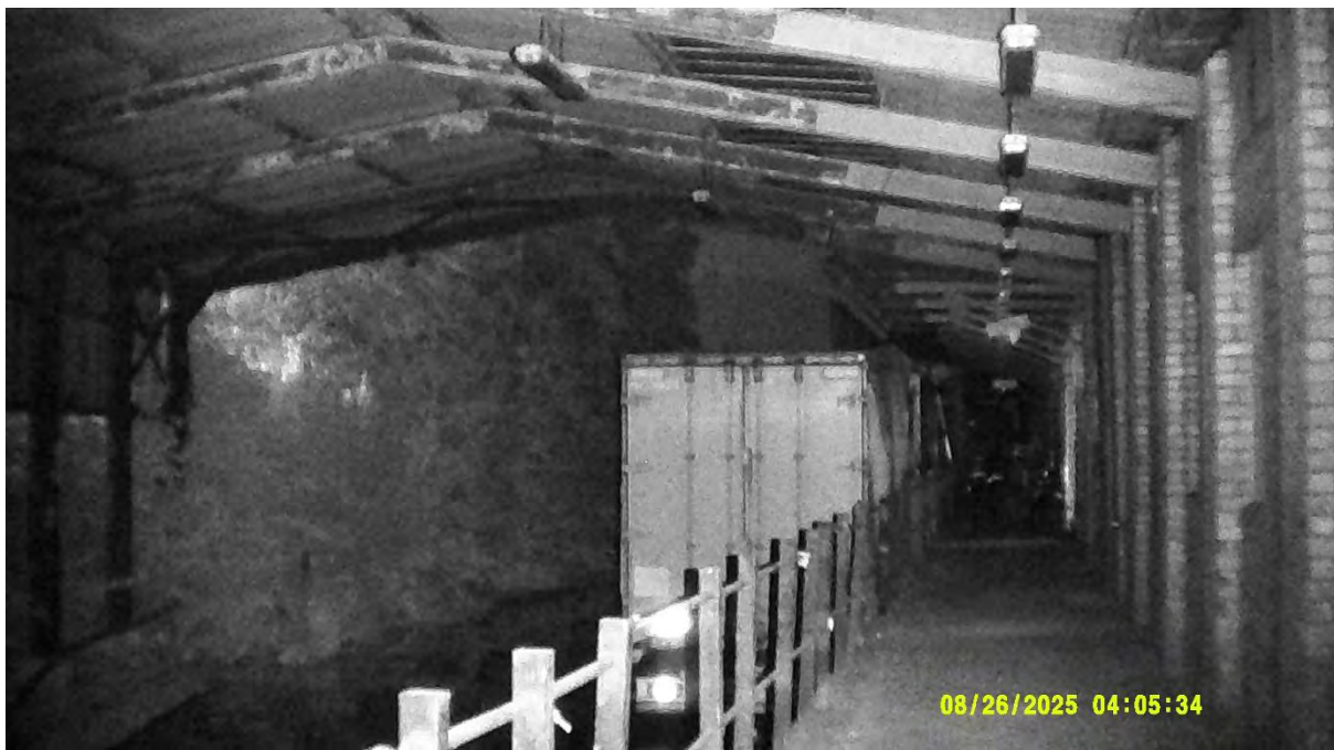
Photograph 8 – Infrared image taken of the northern aspect of Building 1 at the darkest point of the survey at 04:05 on 26 th August 2025.
