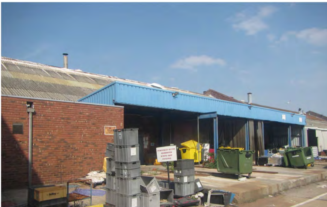
Photograph 2 – A flat roof located along the southern aspect of Building 1.
