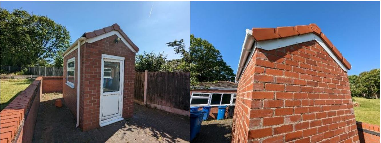
Plate 5 – B3 outbuilding front and rear
