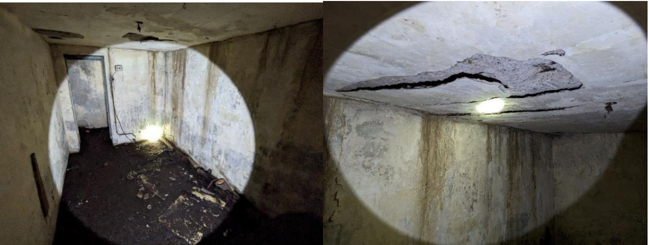
Plate 11 – Target Note 1 air raid shelter – interior and low but potential value crevice in ceiling
