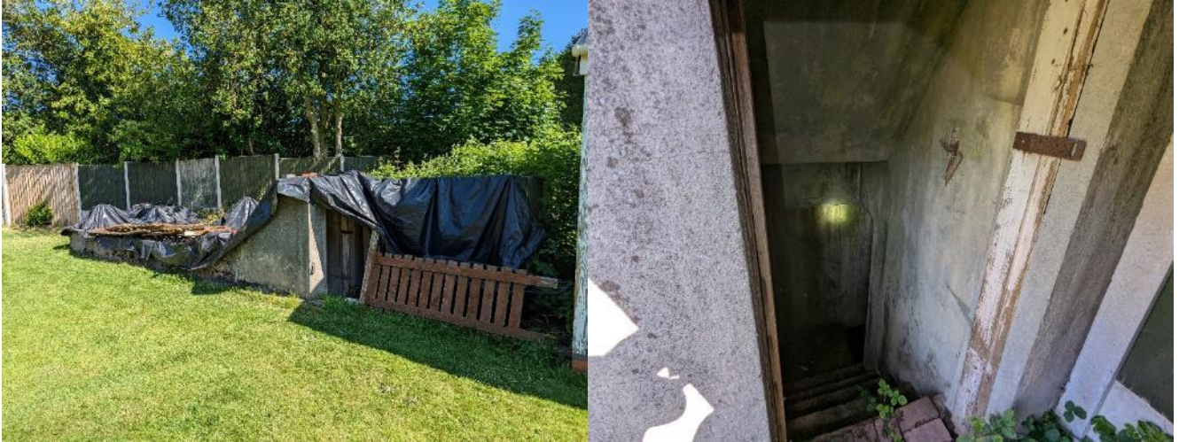
Plate 10 – Target Note 1 air raid shelter with open entrance
