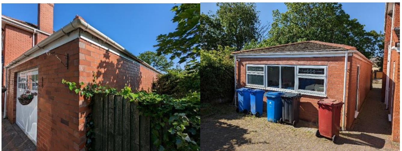
Plate 3 – B2 side garage front and rear
