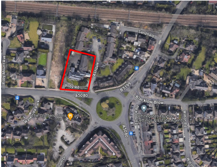
Aerial photograph of site
