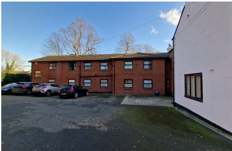
View from Site Car Park
