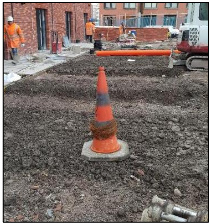
Figure 4: The sub-soil is overlain by 150mm topsoil to FFL:
