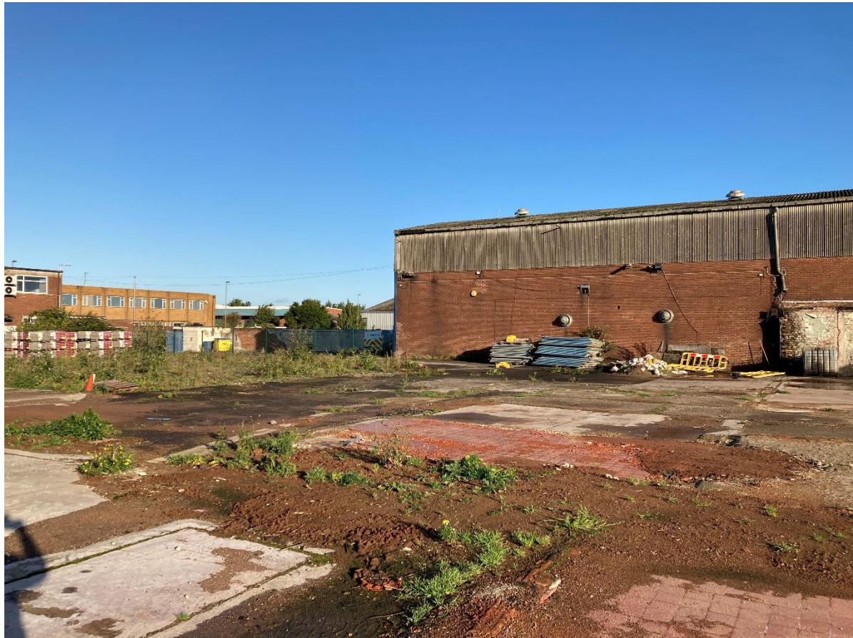
PLATE 5 VIEW NORTHWEST - ACM ON UPPER GARAGE, DEMOLITION RELATED MADE GROUND MIDDLE LEFT OF PHOTO (GRASSY AREA)
