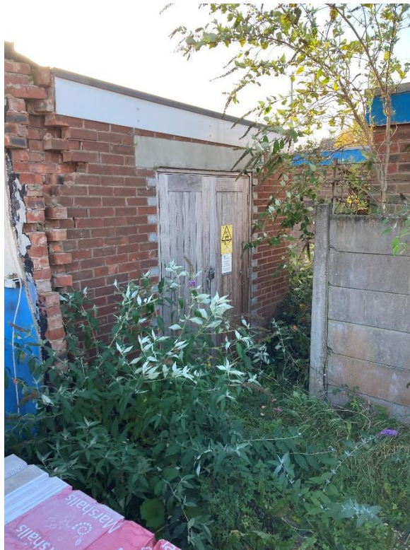
PLATE 1 ELECTRICITY SUBSTATION - BUILDING ON SOUTHERN BOUNDARY LOOKING SE
