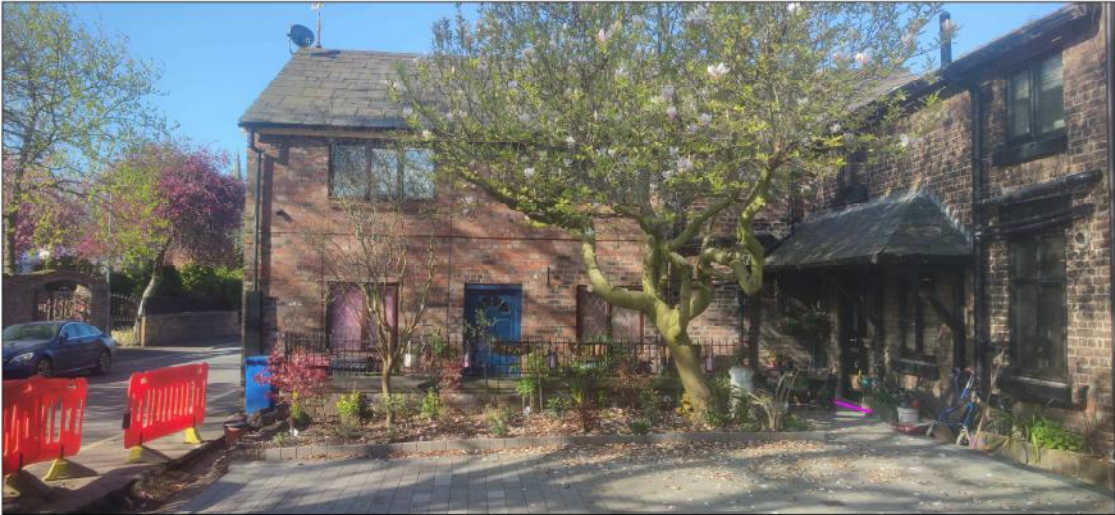
GRIFFIN BARN SIDE ELEVATION & ALREADY DEMOLISHED FRONT WALL
