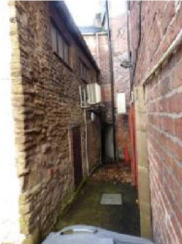
RH rear return stone wall of rear outrigger.
