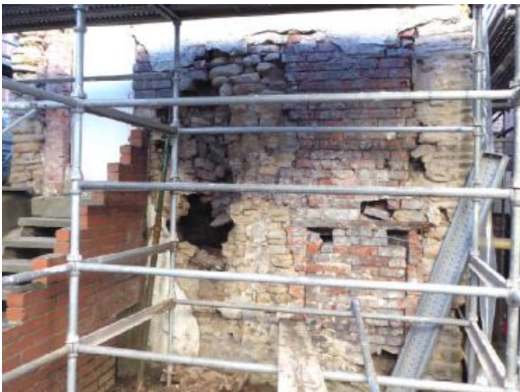
Exposed rear elevation December 2021.
