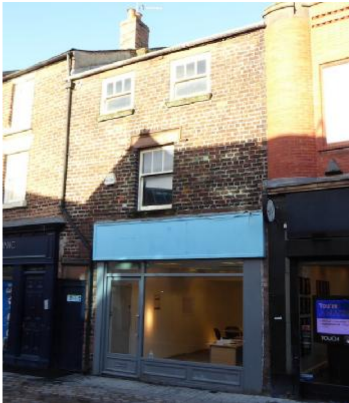
Front Elevation. (Existing shop front currently being replaced under planning application ref: 20/00724/FUL).
