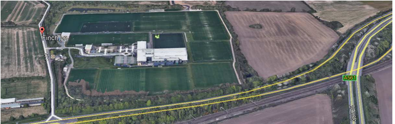
Birds eye view of USM Finch Farm Training Facility from South (A562 Higher Road)
