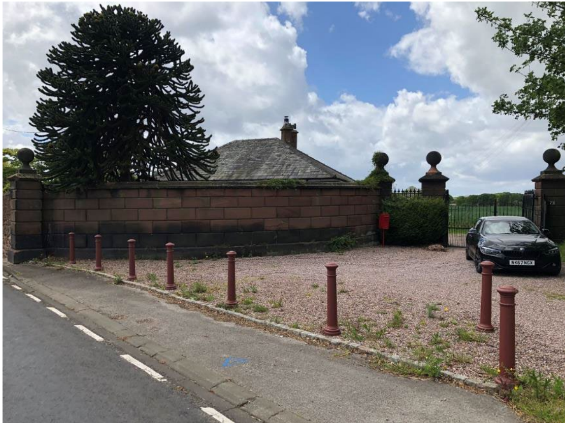
Plate 13. View facing south-west of the eastern entrance to Halsnead Park, with the Grade II listed Lodge behind the curved boundary wall and the adjacent Gate Piers
