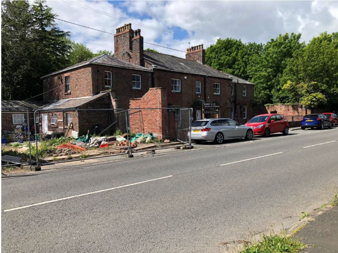
Plate 19. View facing south-west to the northern elevation of Sandfield House. Note the extensive vegetation present to the south of the house
