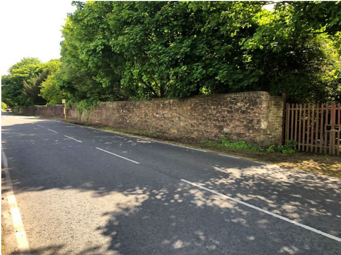
Plate 1. View facing east along Licker's Lane of the boundary wall and gated entrance into the study site
