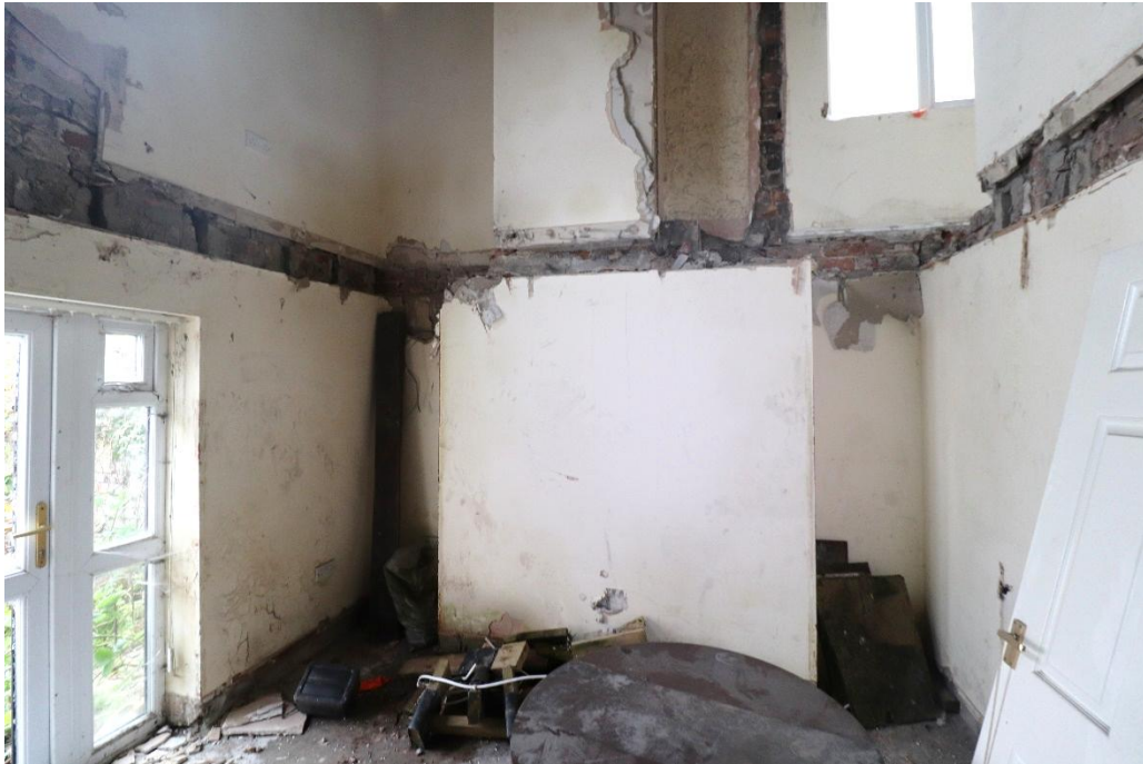
Figure 5-4 - 75 Baileys Lane Interior
