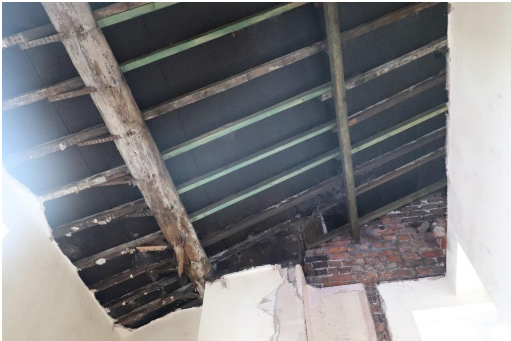
Figure 5-5 - 75 Baileys Lane Underside of Roof
