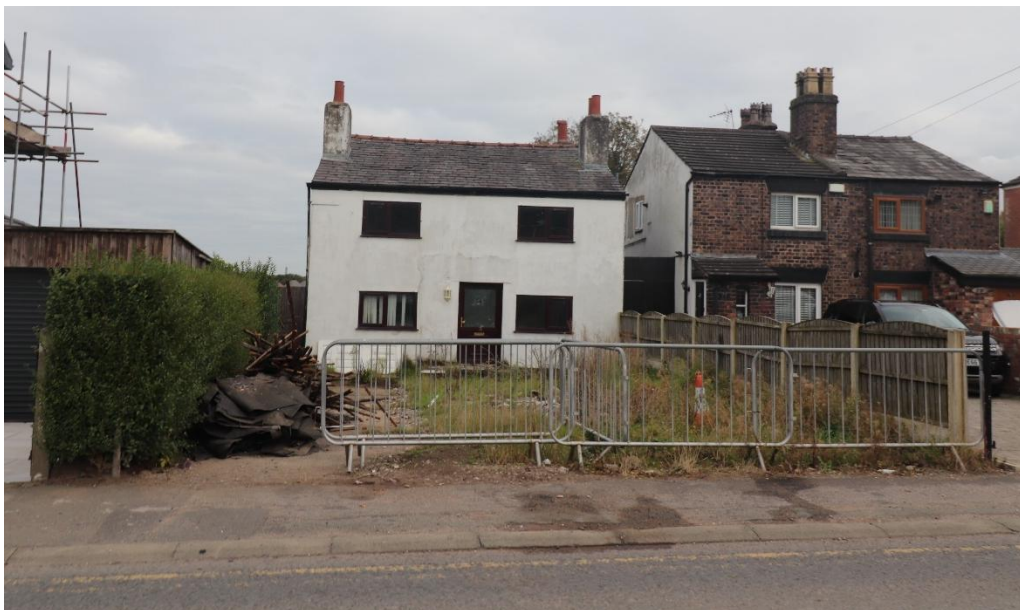
Figure 4-2: Photograph of 75 Baileys Lane (white dwelling in centre of image)
