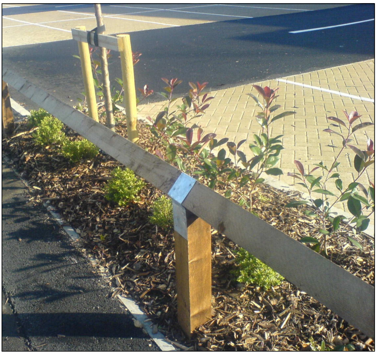
Fence Type 1 - Knee Rail Fencing Diamond knee height barrier.
