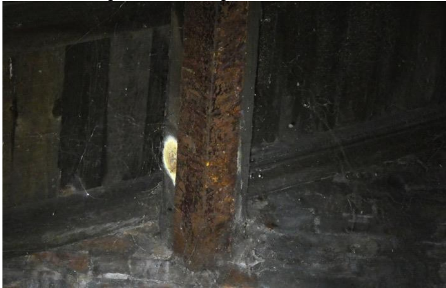
Figure 6. Fungal fruiting body on purlin
