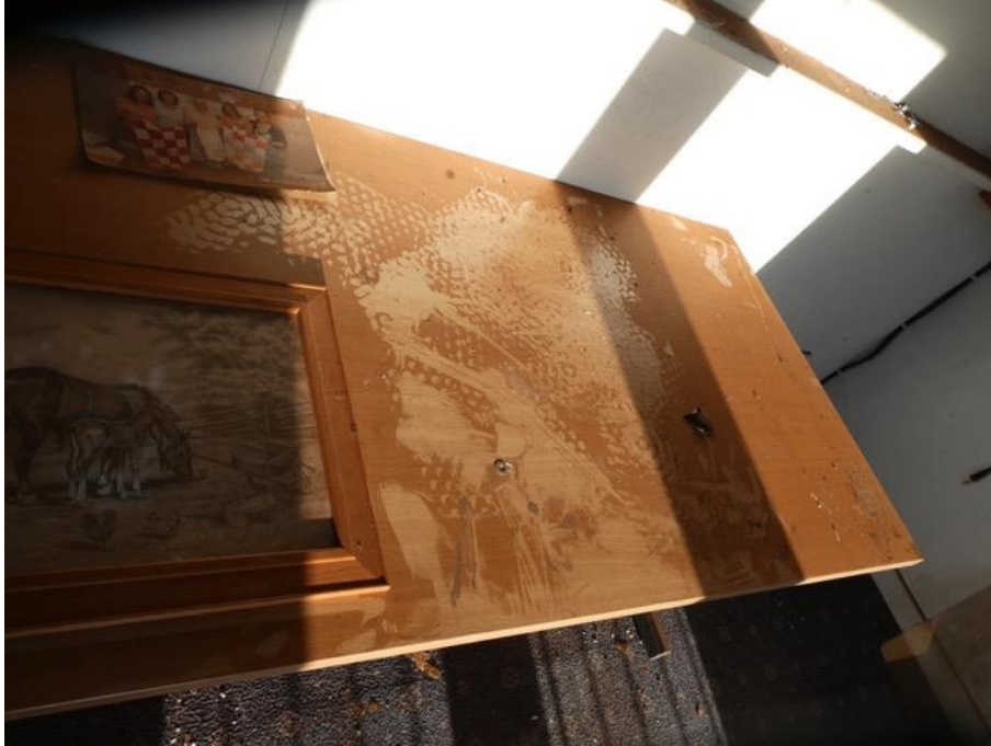
Figure 8. Spores of 'Dry rot' Serpula lacrymans covering all horizontal surfaces.
