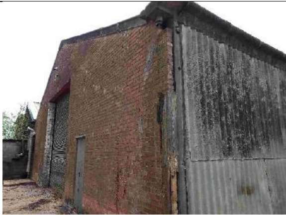
Photograph 13: Eastern and northern elevation of building B2
