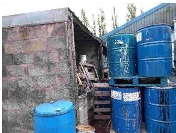
Photograph 18: Single storey storage shed of western elevation of B3
