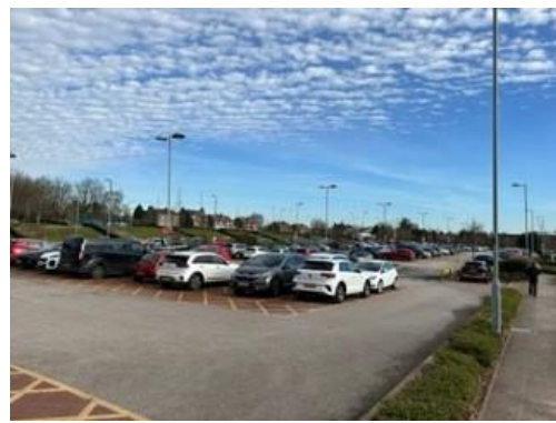
Figure 2.9: Visitor car parking adjacent to the proposed extension.
