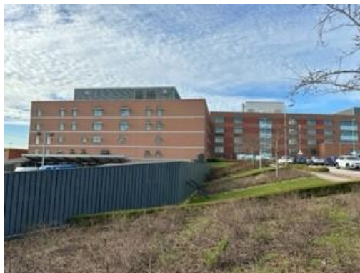
Figure 2.4: West wing of main hospital building where the new extension is proposed to adjoin.
