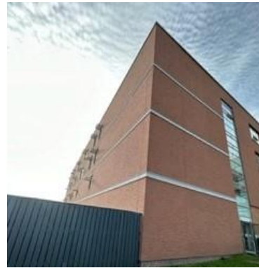
Figure 2.7: Close up of west wing displaying redbrick which will fit in with the proposed materials of the new extension.
