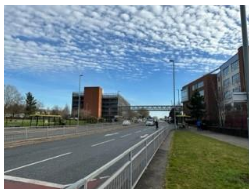
Figure 2.11: Warrington Road where access can be sought to Whiston Hospital.
