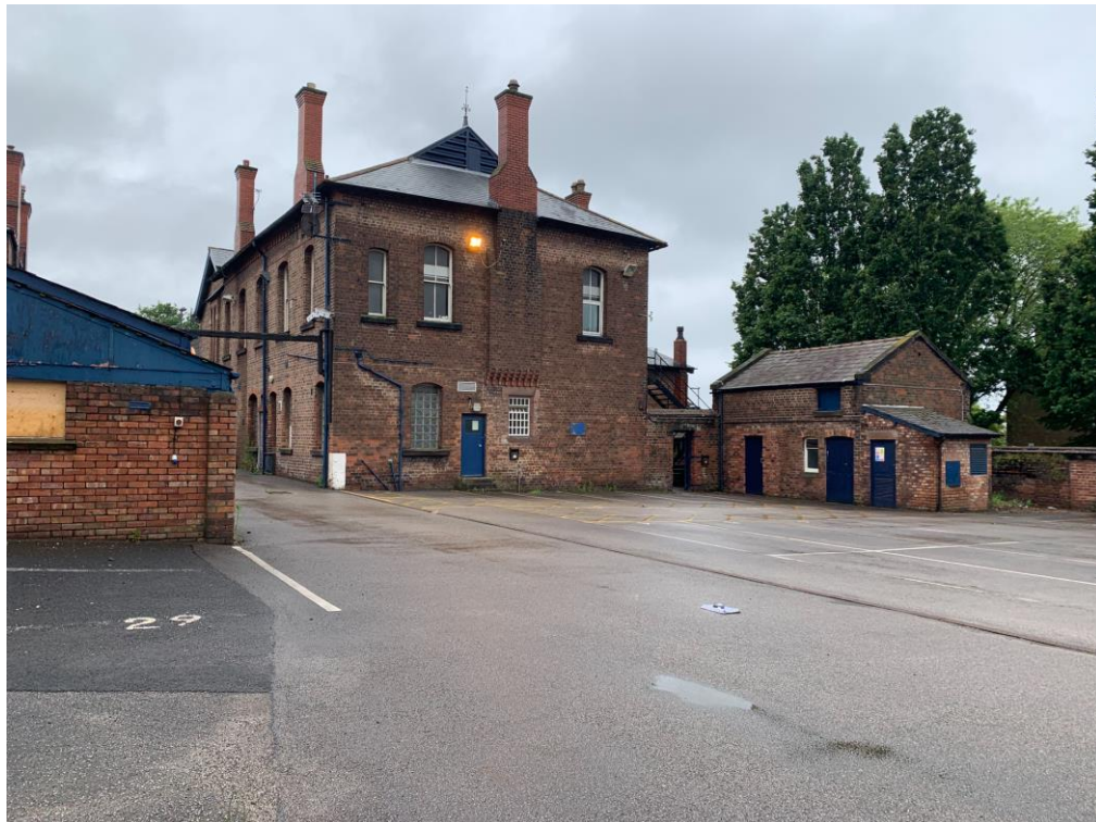
Figure 2 – Former Police Station – view from courtyard of police station and ancillary buildings
