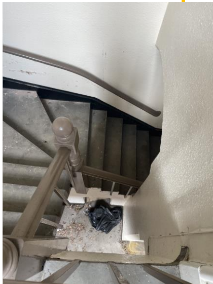
Figure 44 - Original court access stairs
