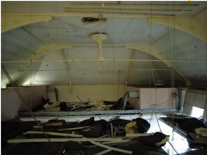
Figure 43 - Original Court roof structure exposed
