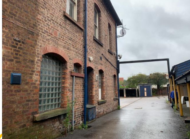
Figure 16 – Principal East Elevation
