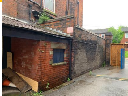
Figure 30 – Existing Store near entrance to site
