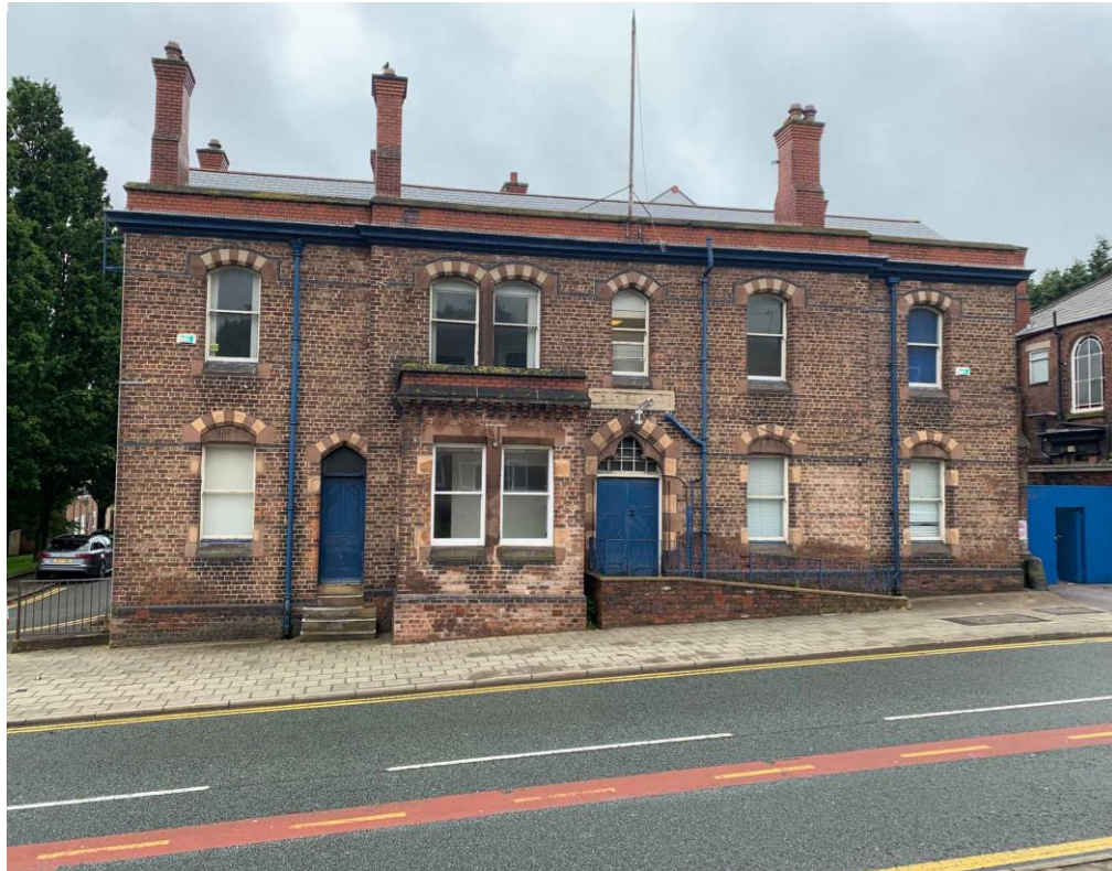
Figure 1 – Former Police Station – view of front elevation from street
