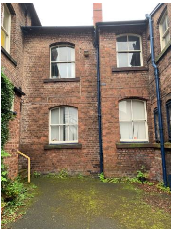
Figure 13– rear inner courtyard
