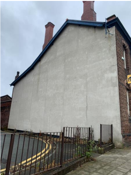
Figure 11 – Principal West Elevation
