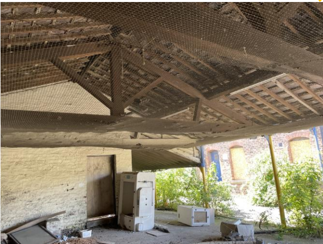
Figure 29 – View of existing canopy in outbuilding 2
