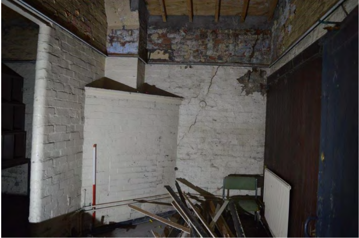
Plate 131. Blocked fireplace in eastern section of Building E, view NNW, scale 1m
