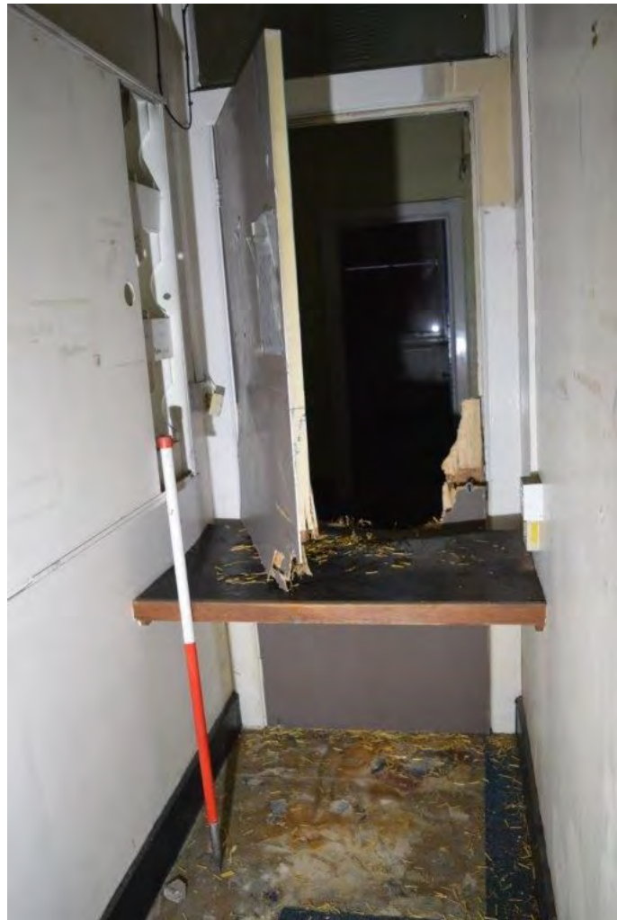
Plate 33. Inserted former counter in lobby north of narrow doorway in RG02, view north, scale 1m
