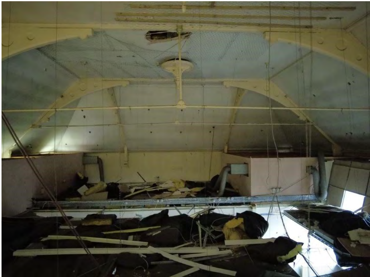
Plate 111. Roof structure of former courtroom above RF14, view north
