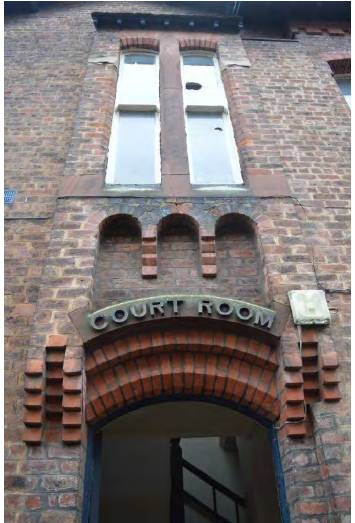
Plate 13. Windows and blind arches above courtroom entrance, view west
