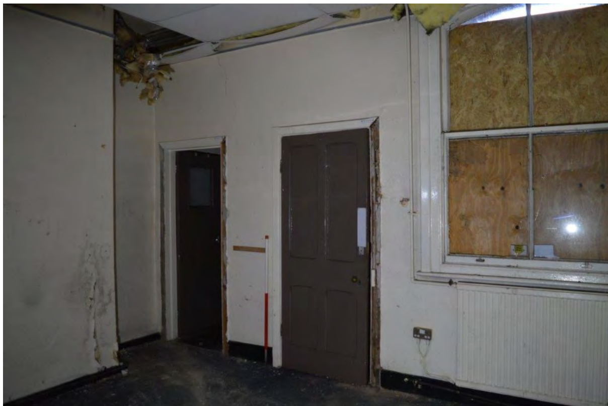
Plate 47. View north-west in RG08, scale 1m
