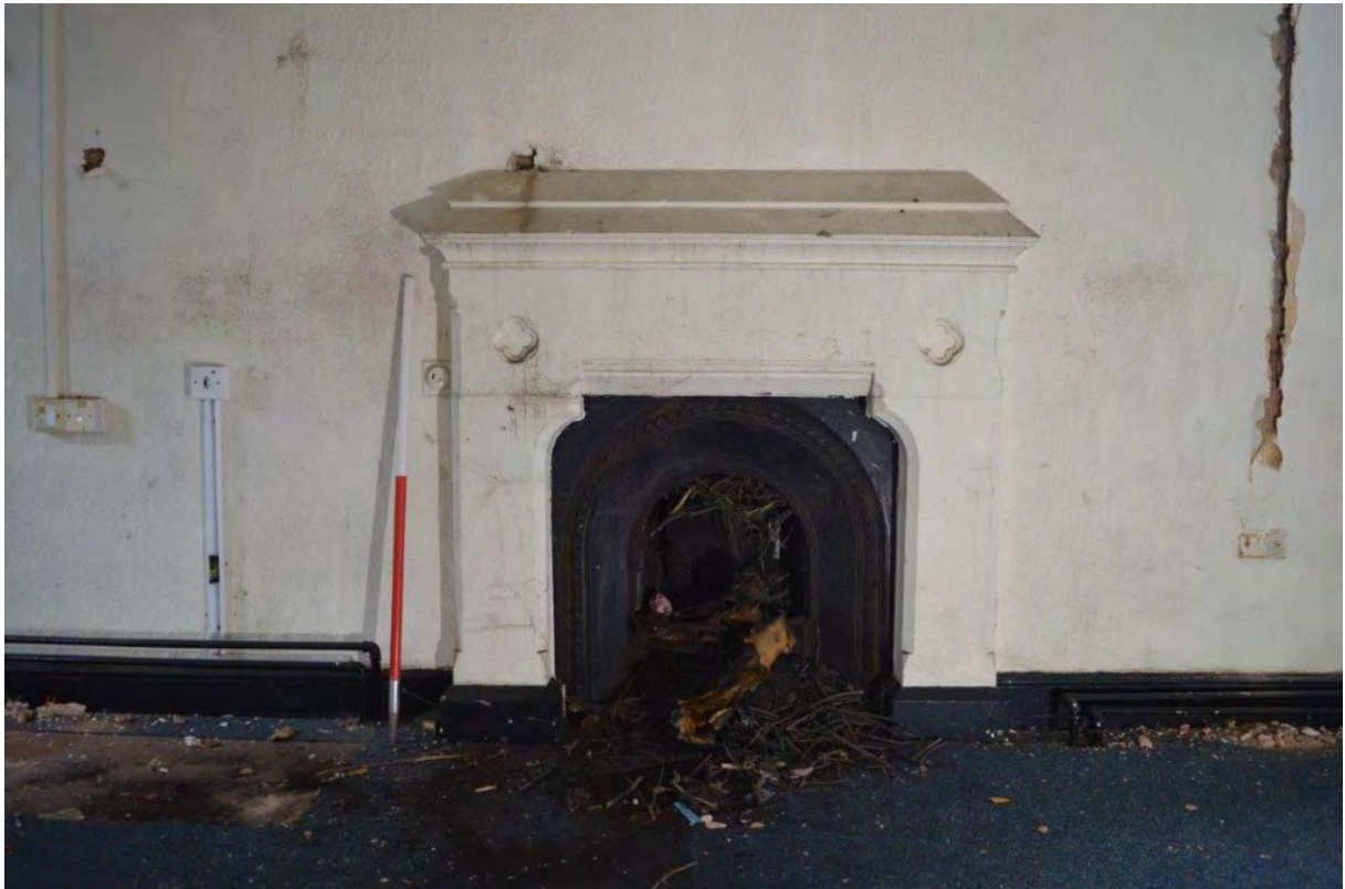
Plate 119. Fireplace in north wall of RF19, scale 1m
