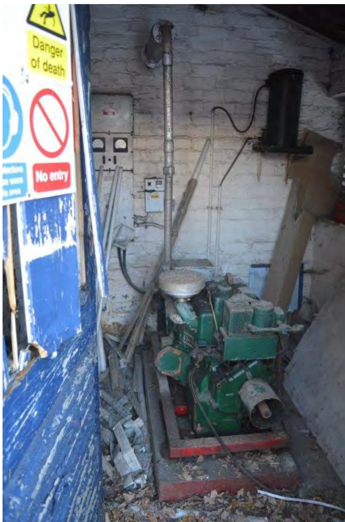
Plate 146. Interior of Building K, view WSW
