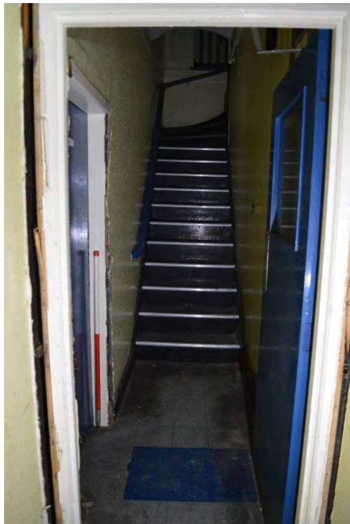
Plate 63. Staircase RG17 facing south, scale 1m
