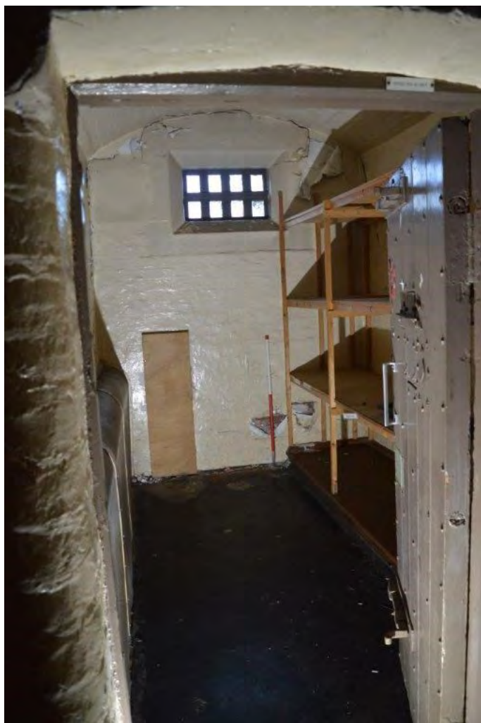
Plate 83. View west into former cell RG27, scale 1m
