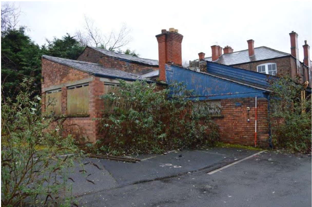
Plate 128. Buildings D and G, view south-west, scale 2m
