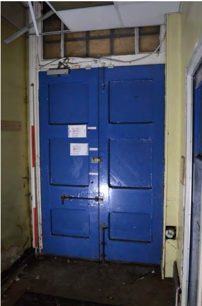
Plate 23. Rear of front doors from lobby RG01 view SSE, scale 2m
