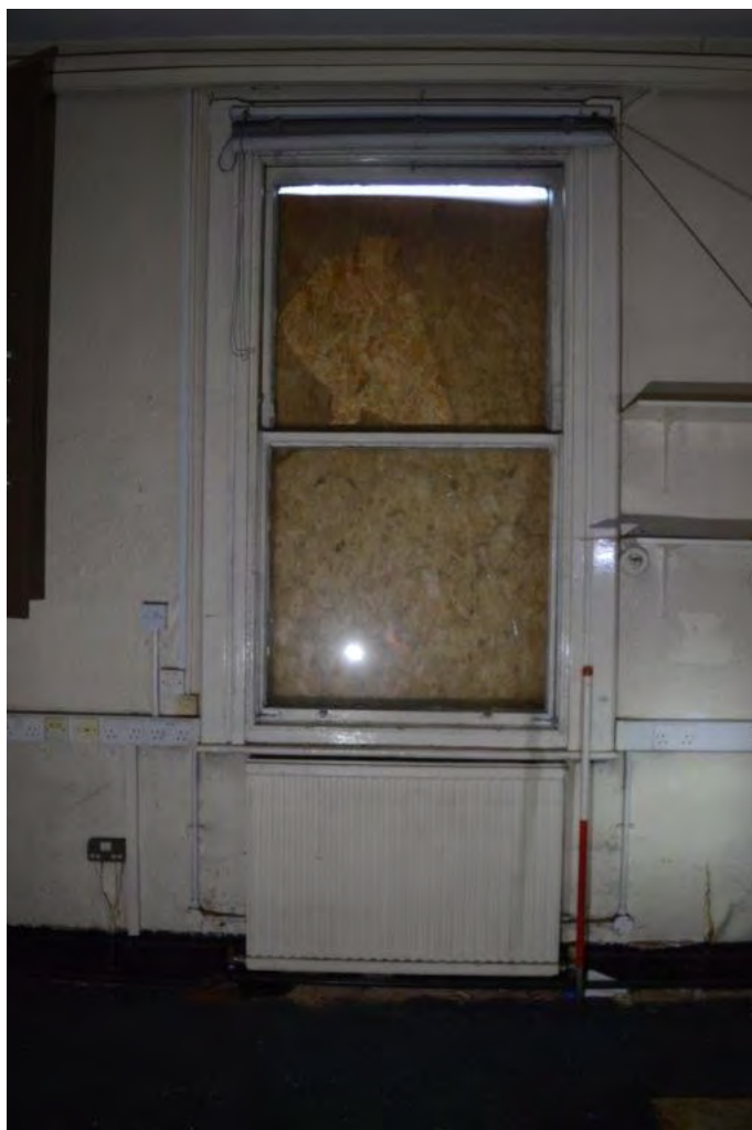
Plate 37. Single hung sash window in south wall of RG03 facing Derby Street, view south, scale 1m
