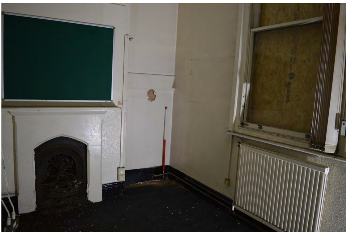
Plate 92. View south-east in RF04, scale 1m
