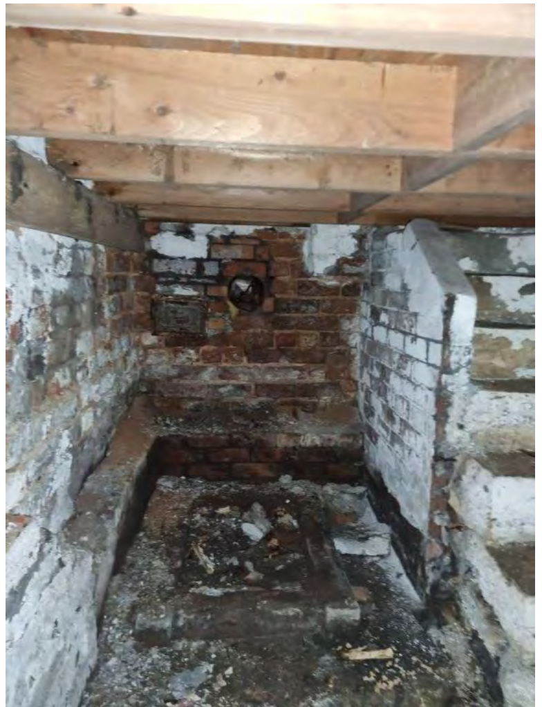
Plate 59. Bonded timbers in south wall of former stone staircase to dock, view north-east
