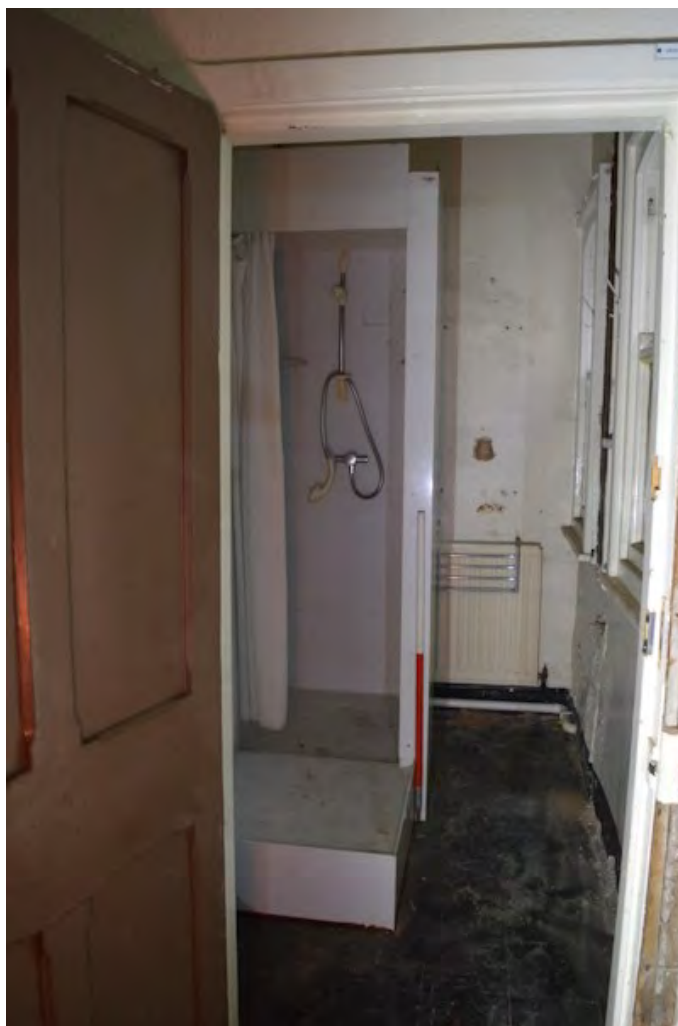
Plate 50. View north into shower area RG09, scale 1m
