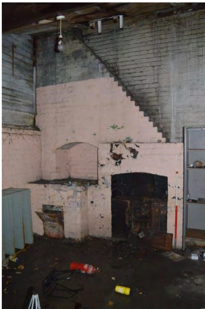
Plate 129. Interior of Building D, view north-east, scale 1m
