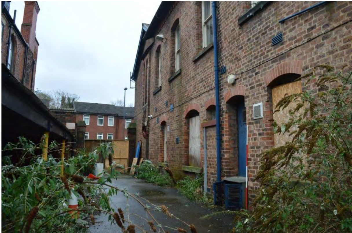
Plate 4. Accessway at east of building, view south, scale 2m
