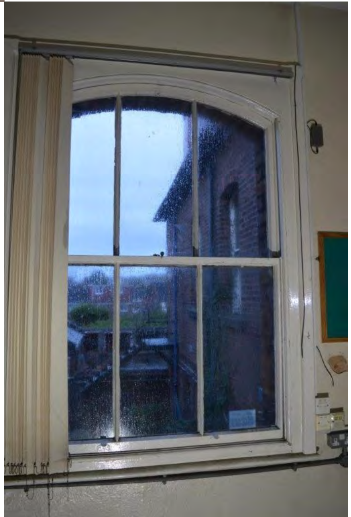
Plate 104. Window in north wall of RF12, scale 1m
