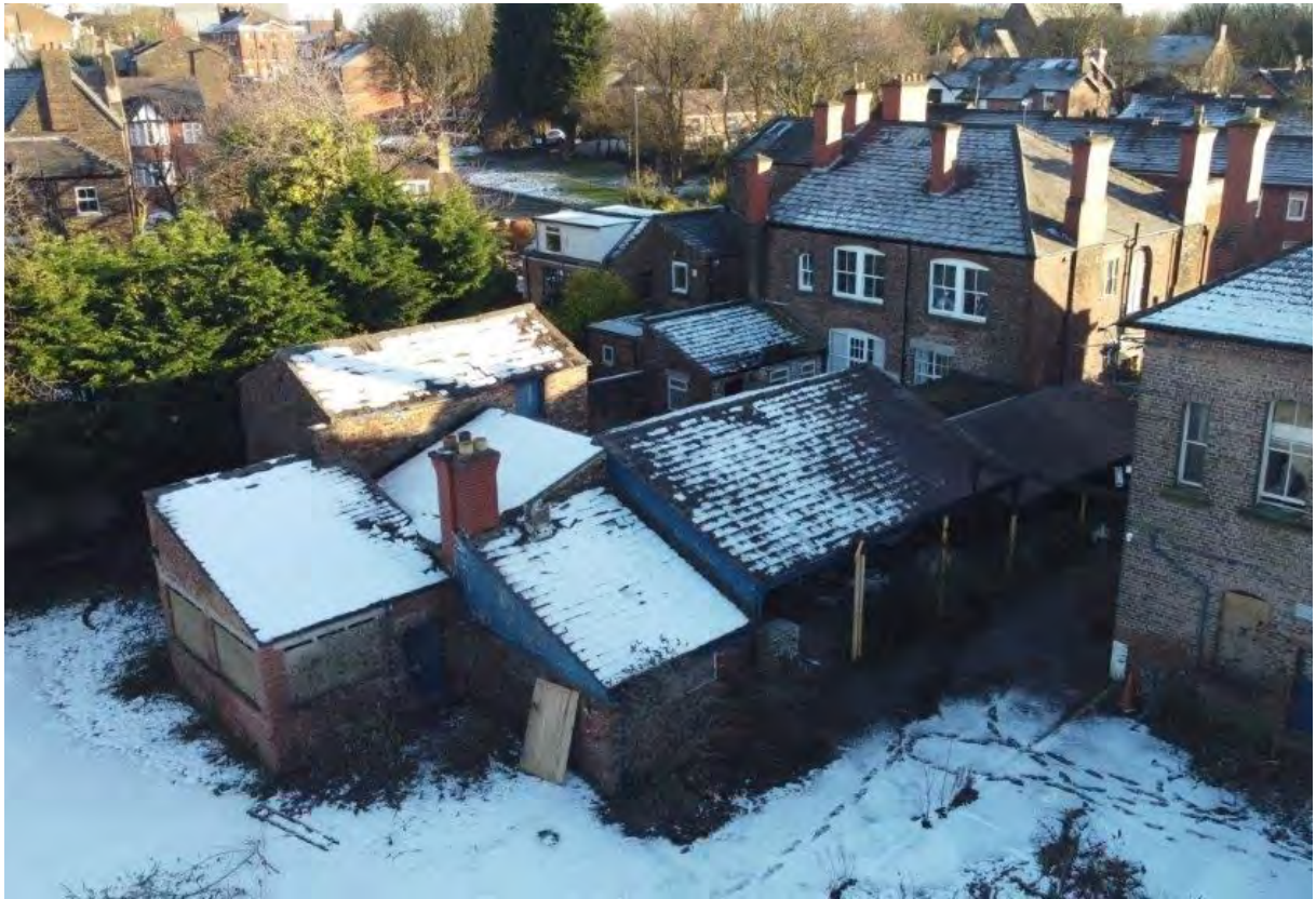
Plate 125. low level aerial view of buildings B-G, view south-east
