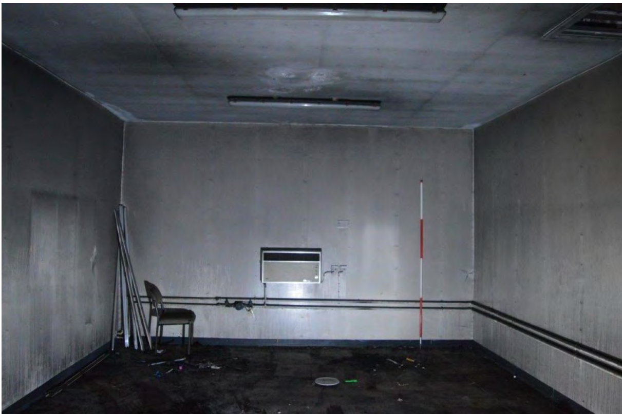
Plate 134. Interior of Building F, view NNW, scale 2m
