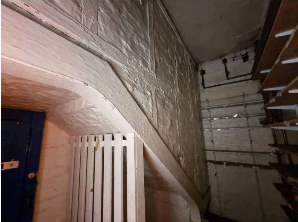
Plate 59. Bonded timbers in south wall of former stone staircase to dock, view north-east
