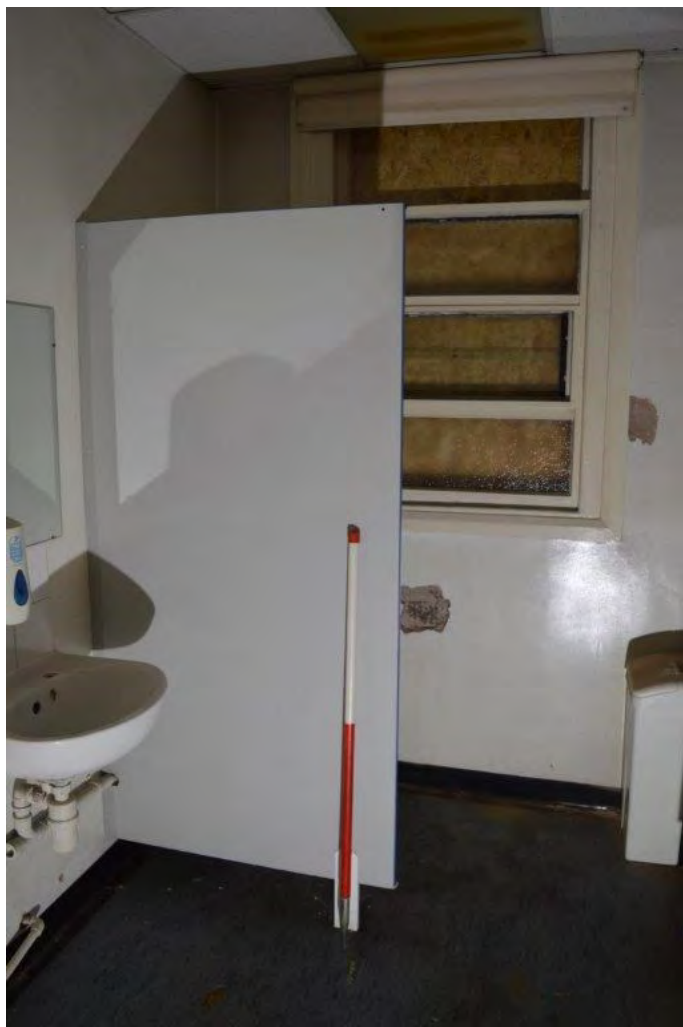
Plate 93. View SSE into toilet RF05/RF05A, scale 1m
