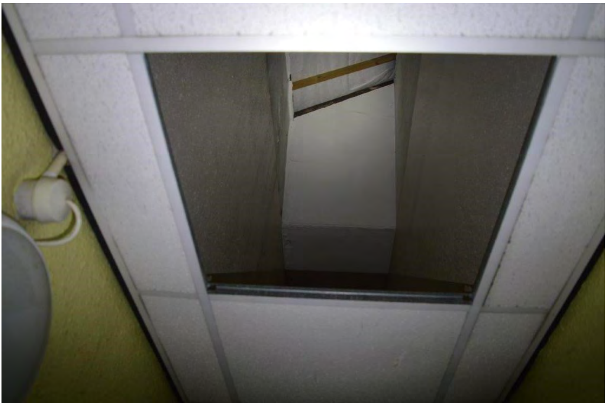
Plate 108. Roofline visible through suspended ceiling above RF13
