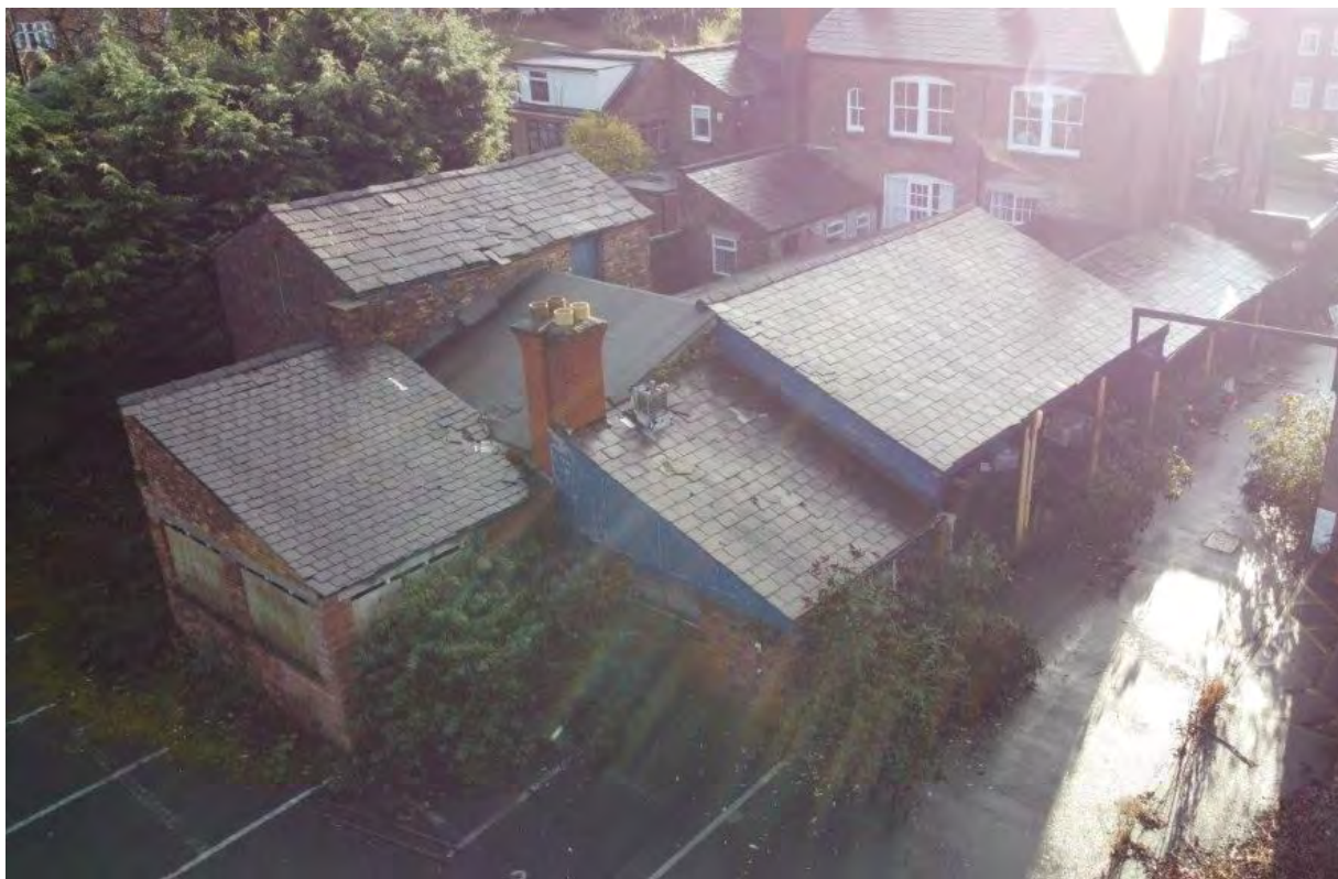
Plate 6. Low level aerial view of Buildings A-G, view south-east
