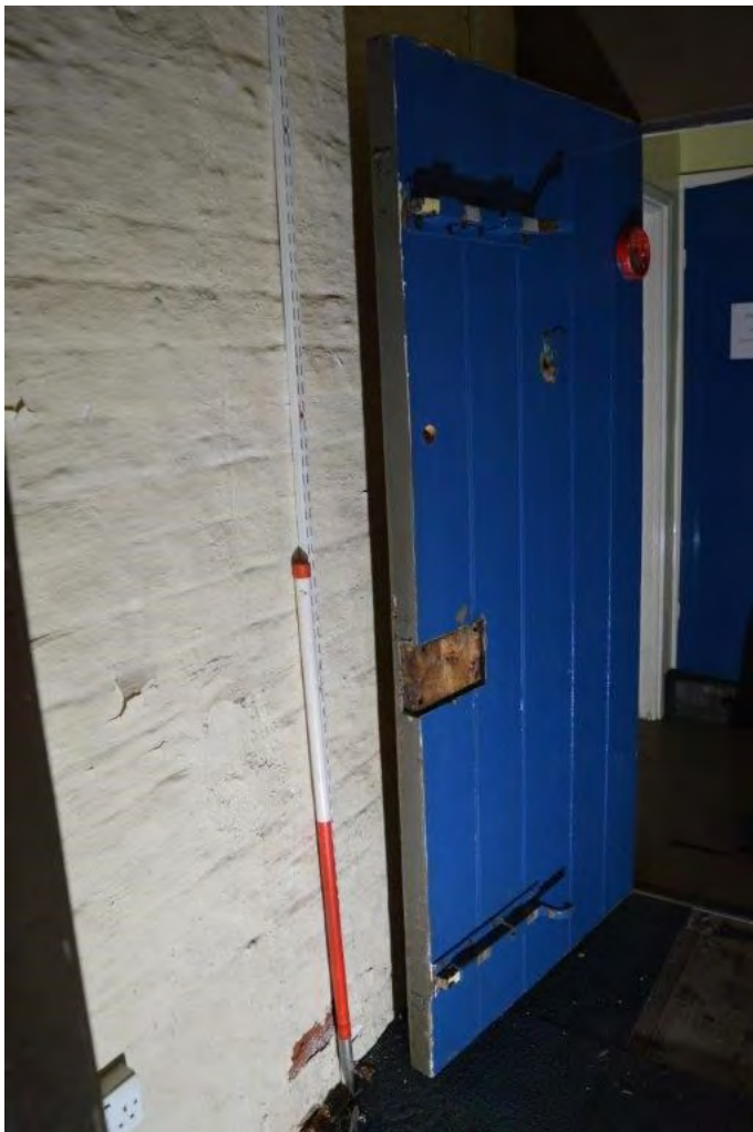
Plate 78. Heavy duty security door to south of RG25, scale 1m
