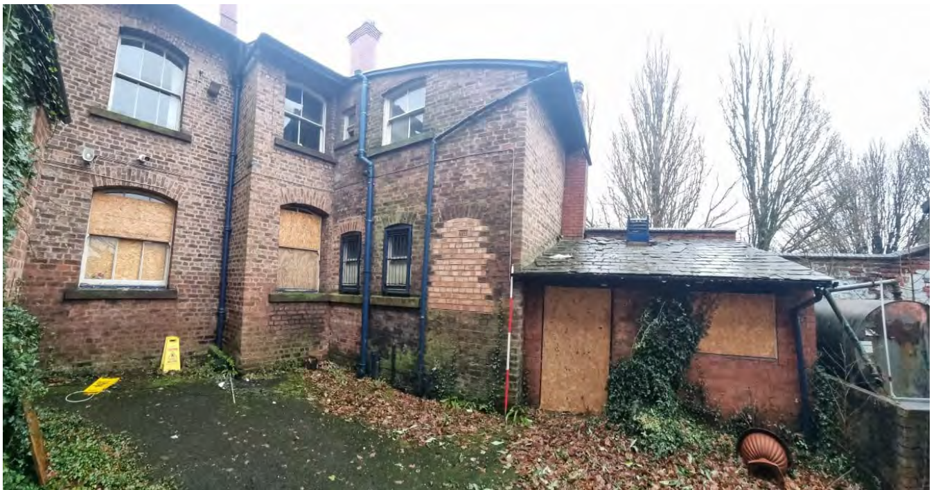
Plate 20. Northward projection section of police station west of courtyard and boiler house, view south-west
