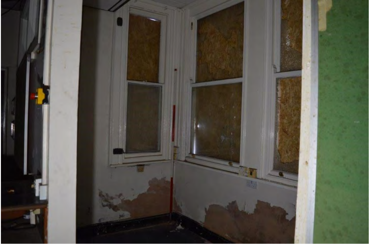
Plate 31. Interior of bay window at front of RG02, view south-east
