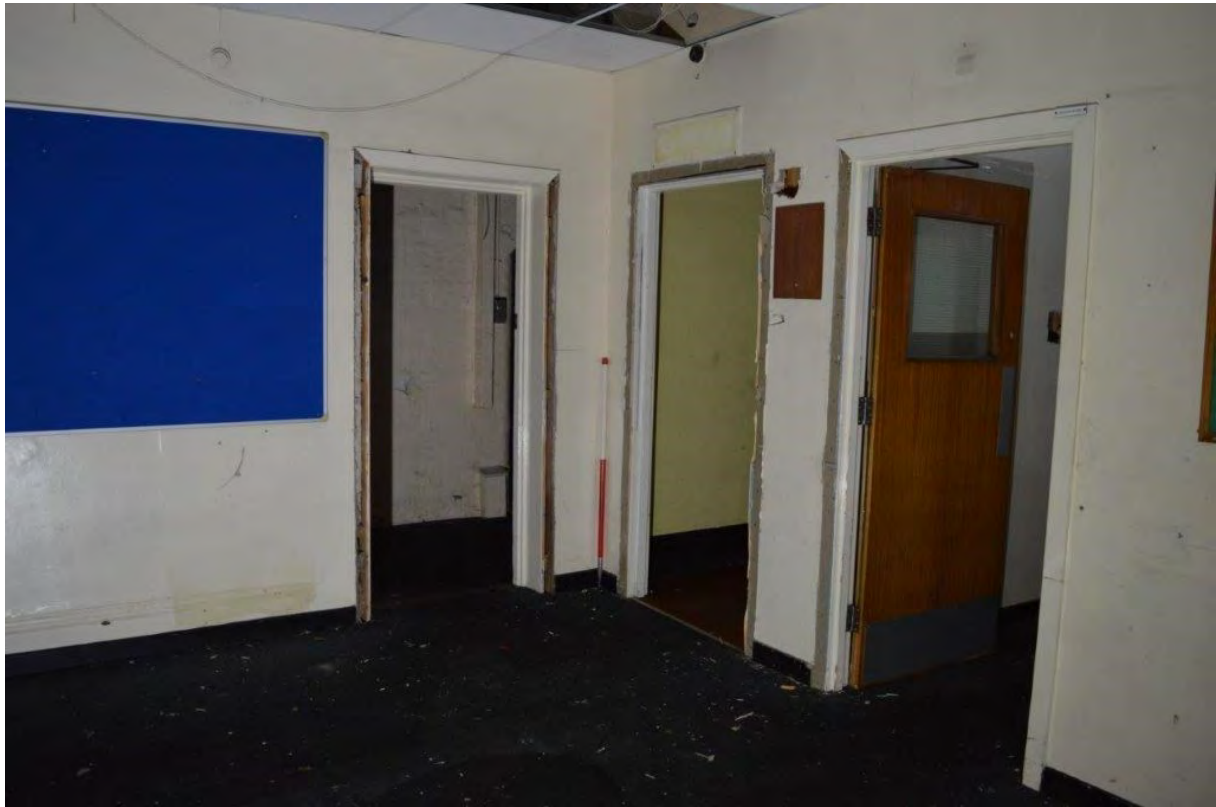
Plate 71. View north-east in RG21, door to cell corridor RG24 on left, scale 1m
