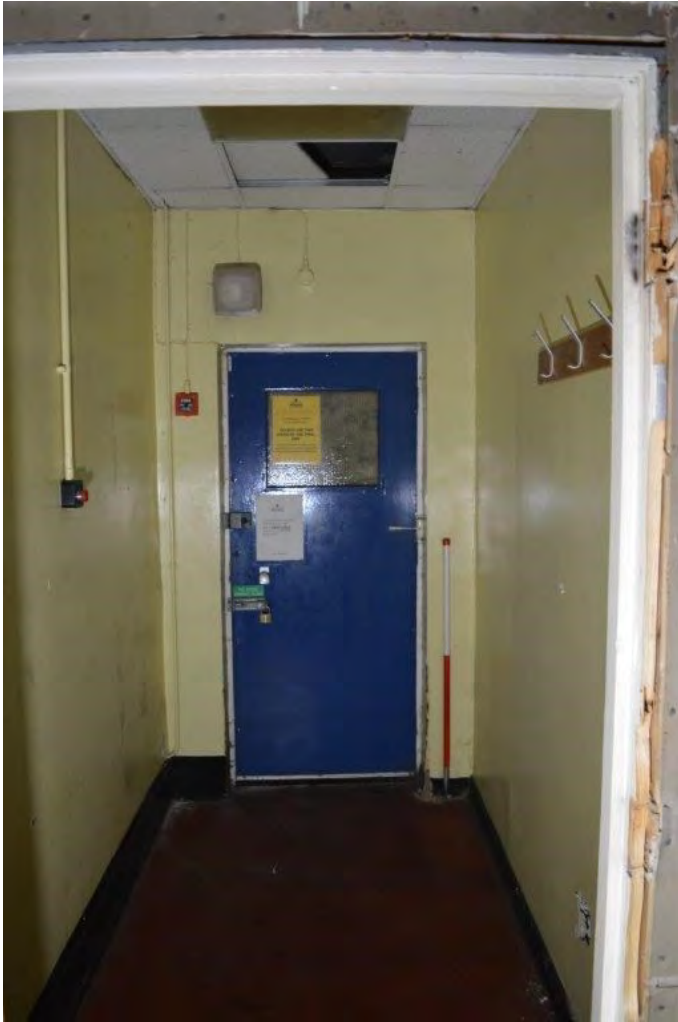
Plate 73. View north in corridor RG23 to inserted doorway in north wall of courtroom wing, scale 1m
