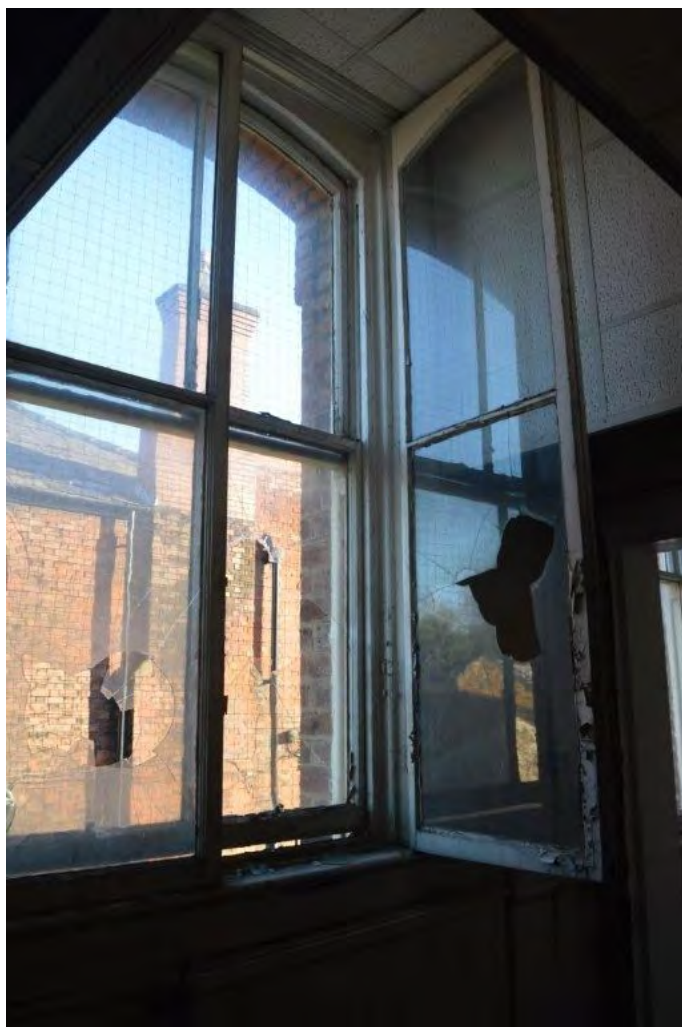
Plate 113. Window in east wall of RF14 with internal casement, view south-east
