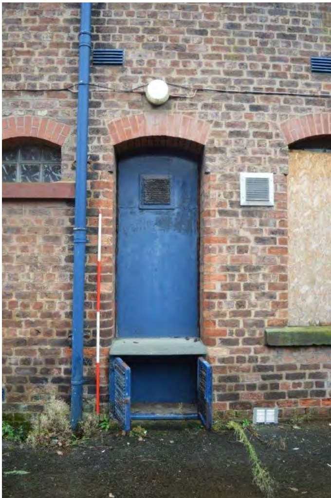
Plate 14. Doorway to RG21 (blocked from inside), view west, scale 2m
