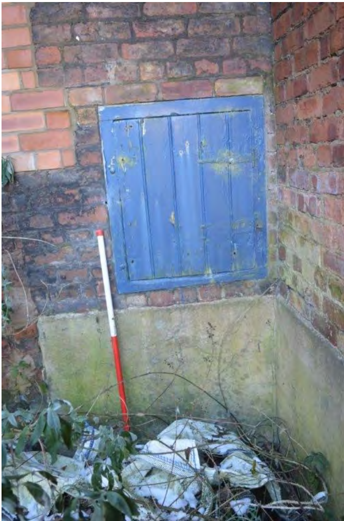
Plate 133. hatch in northern wall of Building F, view SSE
