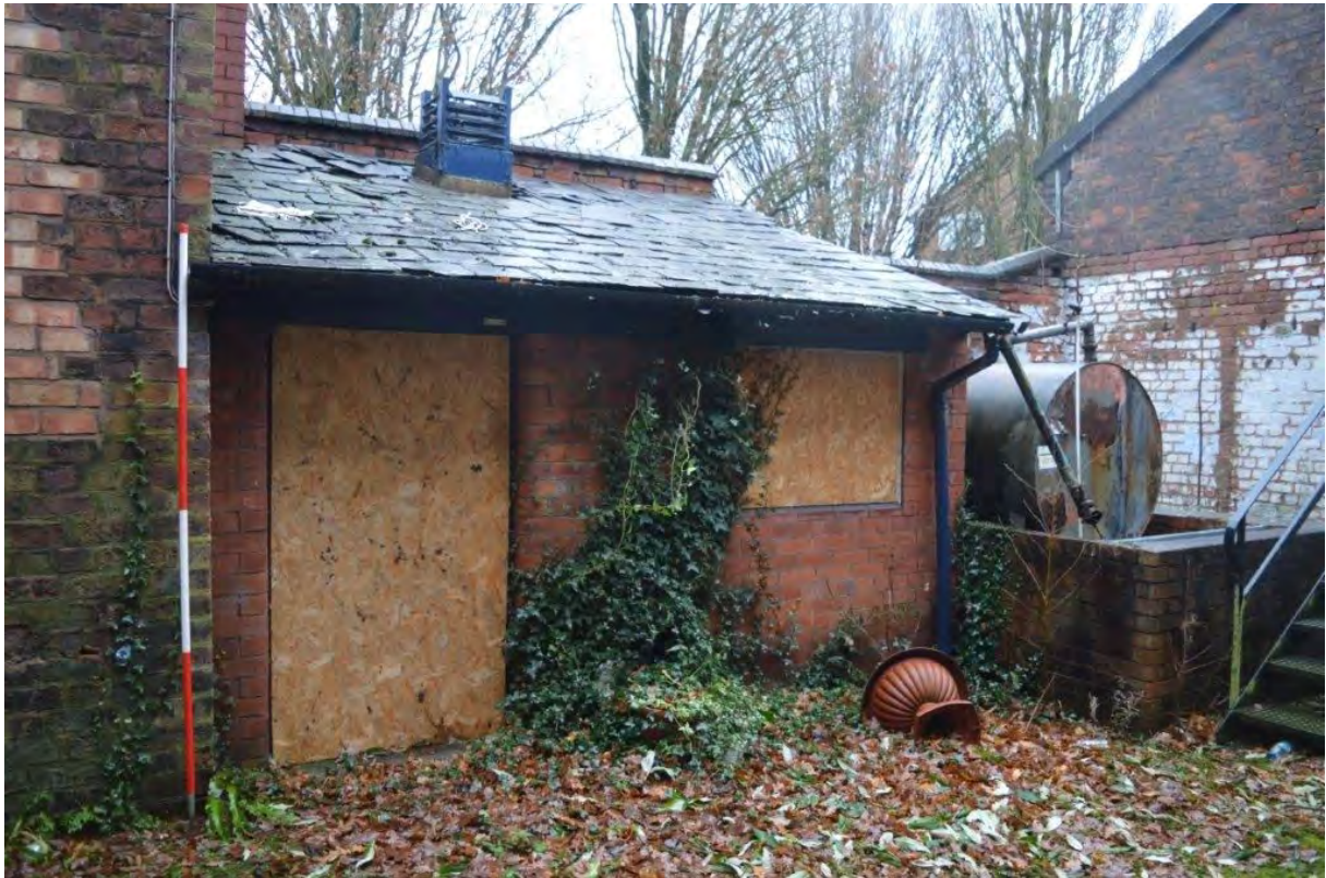
Plate 147. Building L, former boiler house, view west, scale 2m
