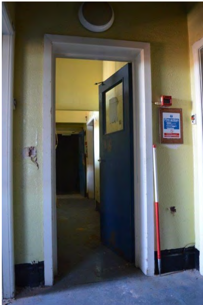
Plate 98. Inserted doorway between RF08 and RF02, view east, scale 1m
