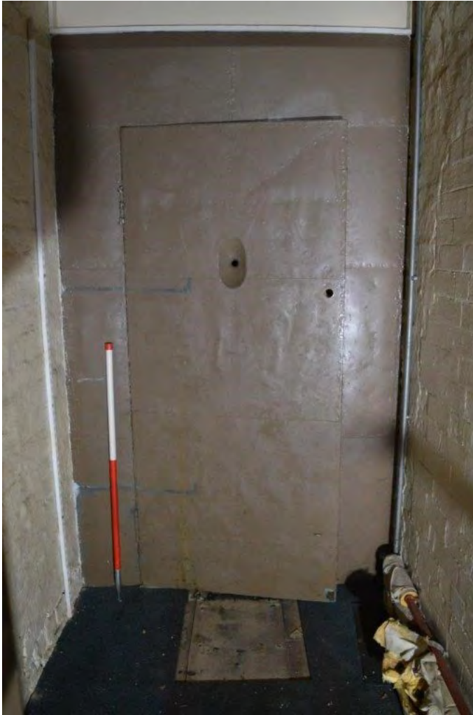
Plate 79. Metal plated rear of security door, scale 1m
