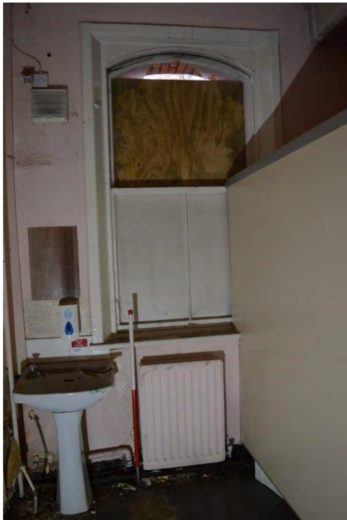
Plate 64. Single hung sash window in RG18a, view ESE, scale 1m
