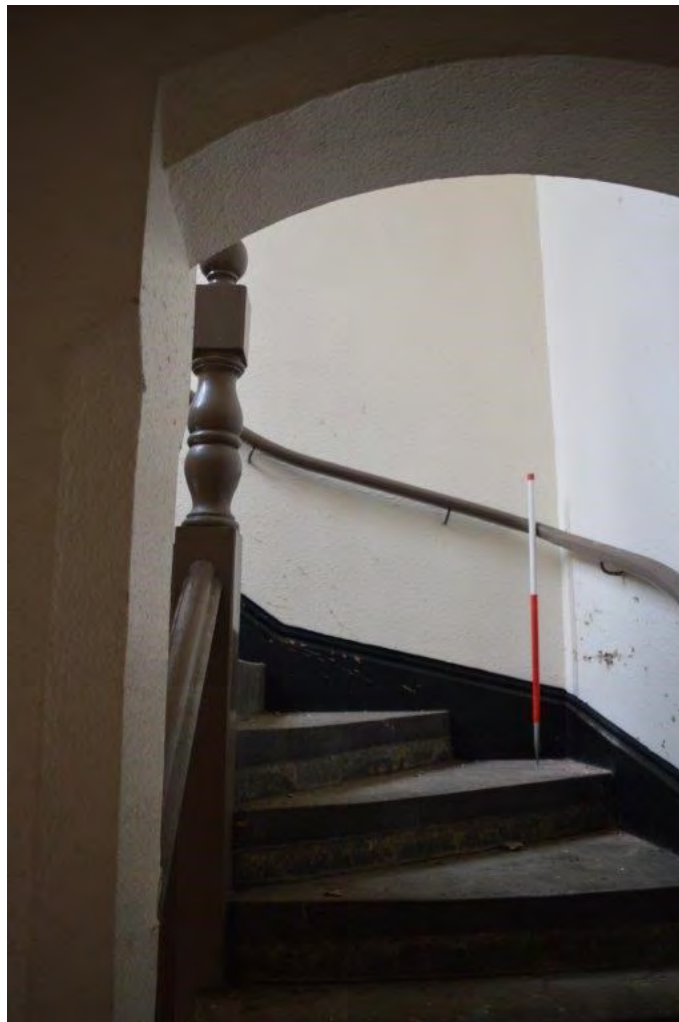
Plate 86. View south up courtroom stairs from first landing, scale 1m
