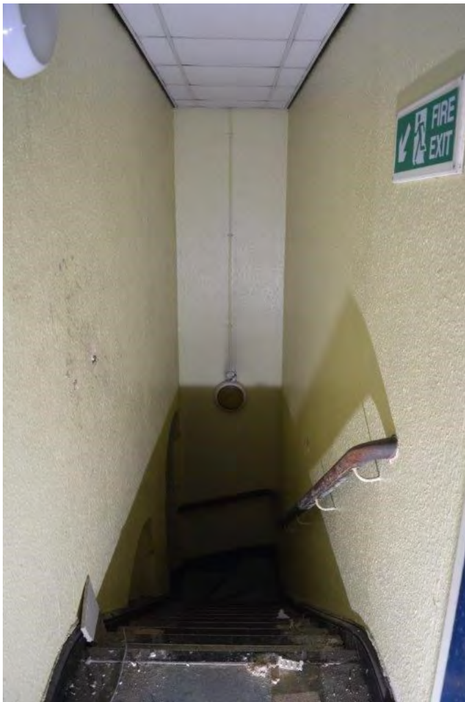
Plate 106. Stairwell RF13/RG11 facing east
