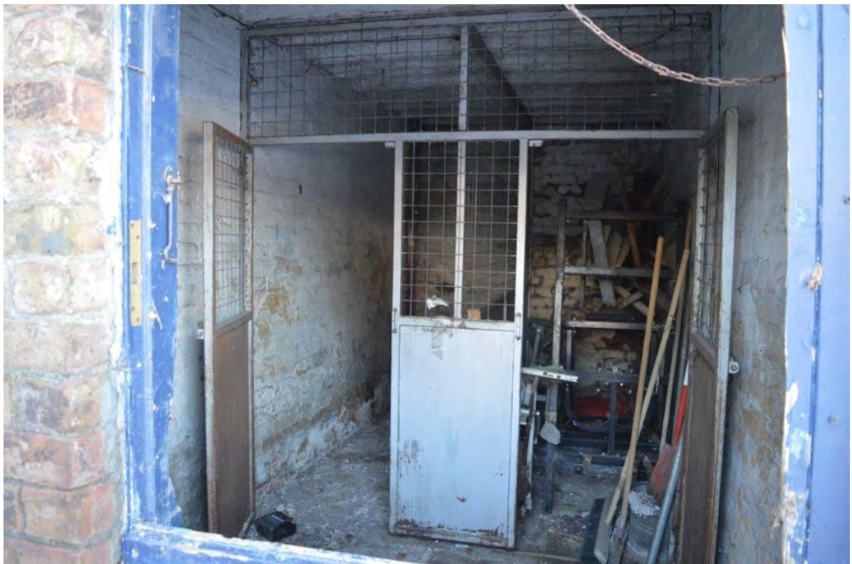
Plate 142. Northern section of Building J. view WSW
