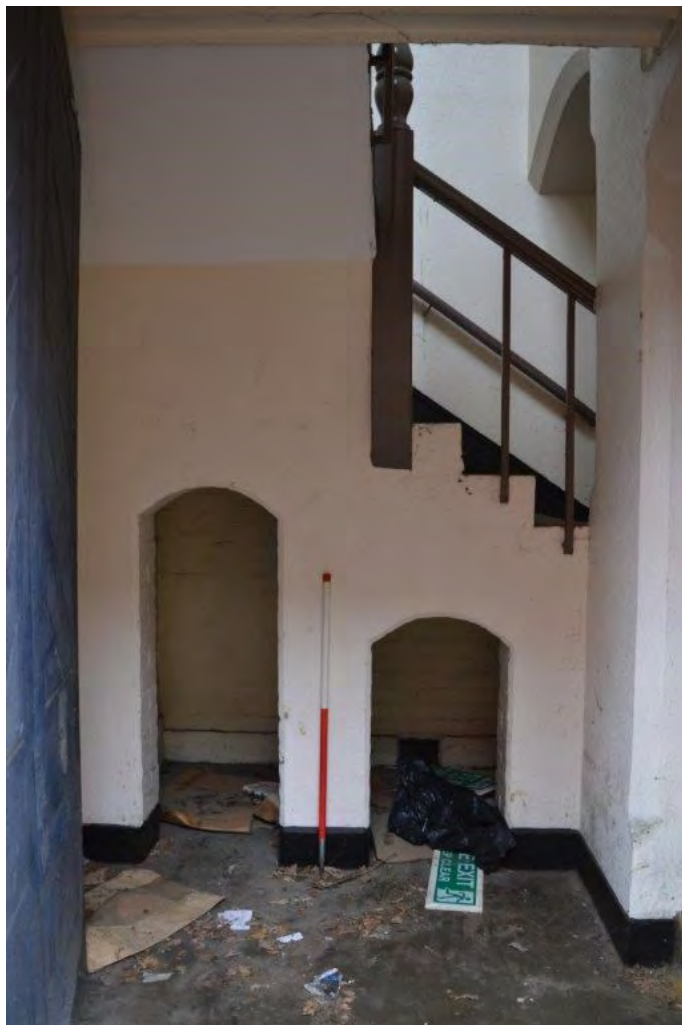
Plate 85. View west to base of formal stairs to courtroom, RG30, scale 1m
