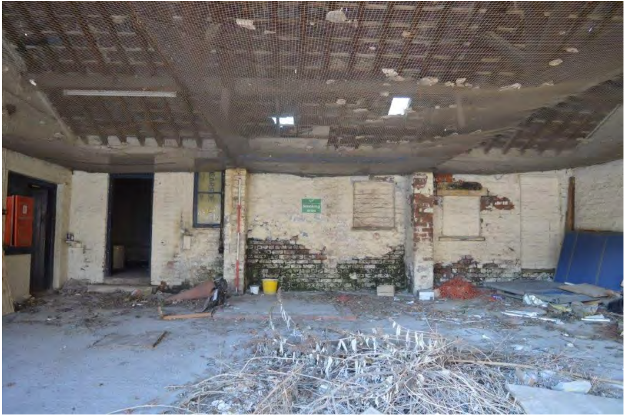
Plate 127. Interior of Building C, view east to Building F (doorway and window to left) and wall to adjacent property (right), scale 2m
