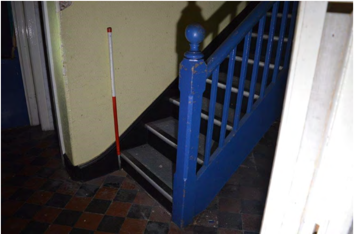
Plate 42. Base of stairwell RG06, view south-west
