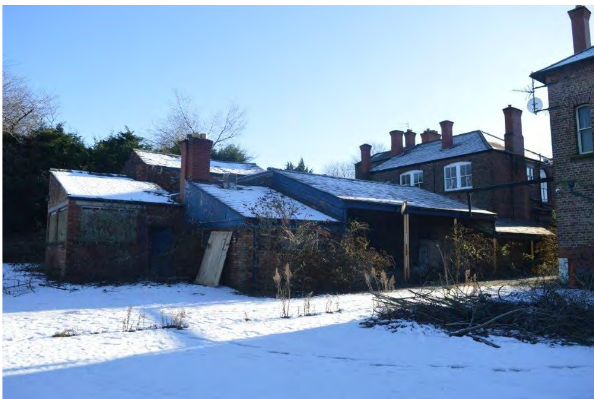
Plate 124. Buildings B-G view south-east
