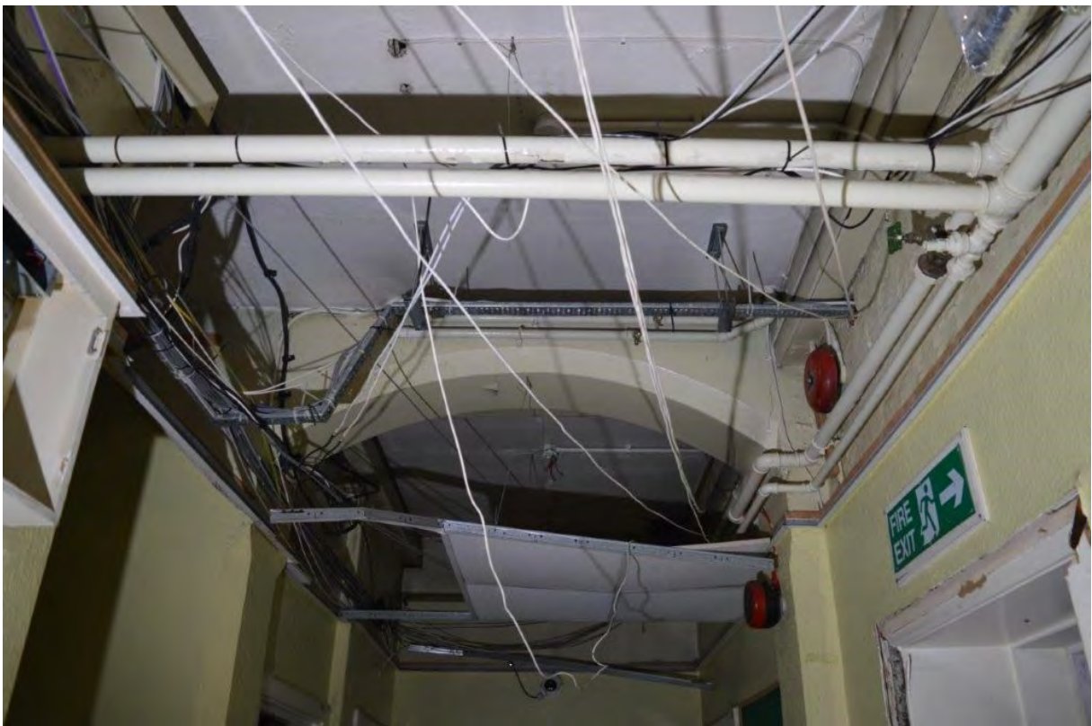
Plate 26. Arch over central section of RG01 adjacent to stairwell RG11, view south
