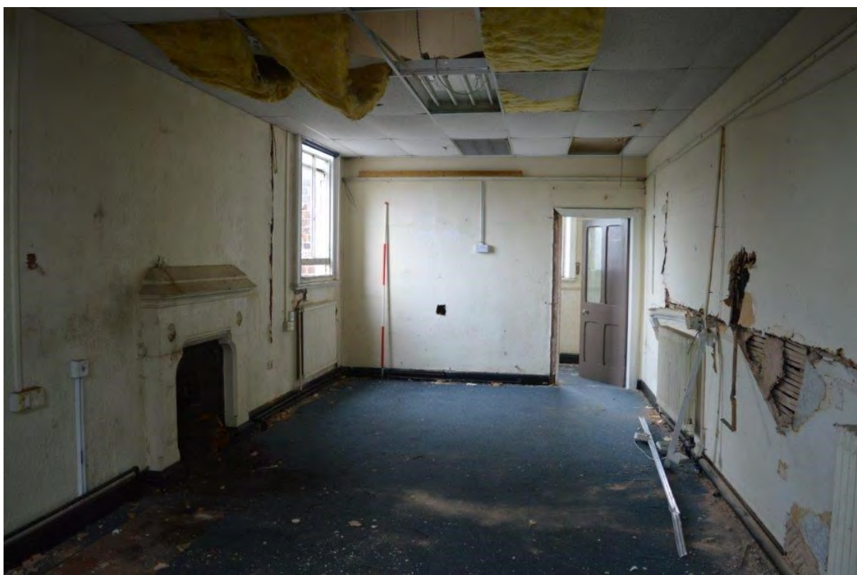
Plate 118. View ENE in former magistrate's retiring room, RF19, scale 2m
