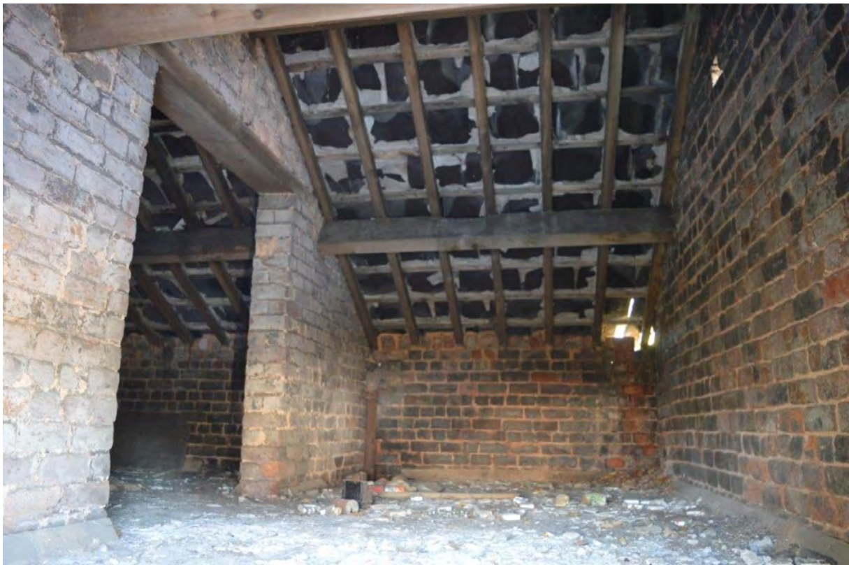
Plate 144. Upper floor of stables, Building J, probable former hay loft
