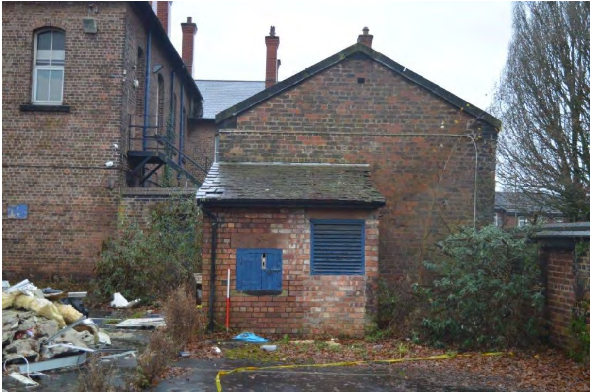
Plate 145. Building K, view south, scale 1m
