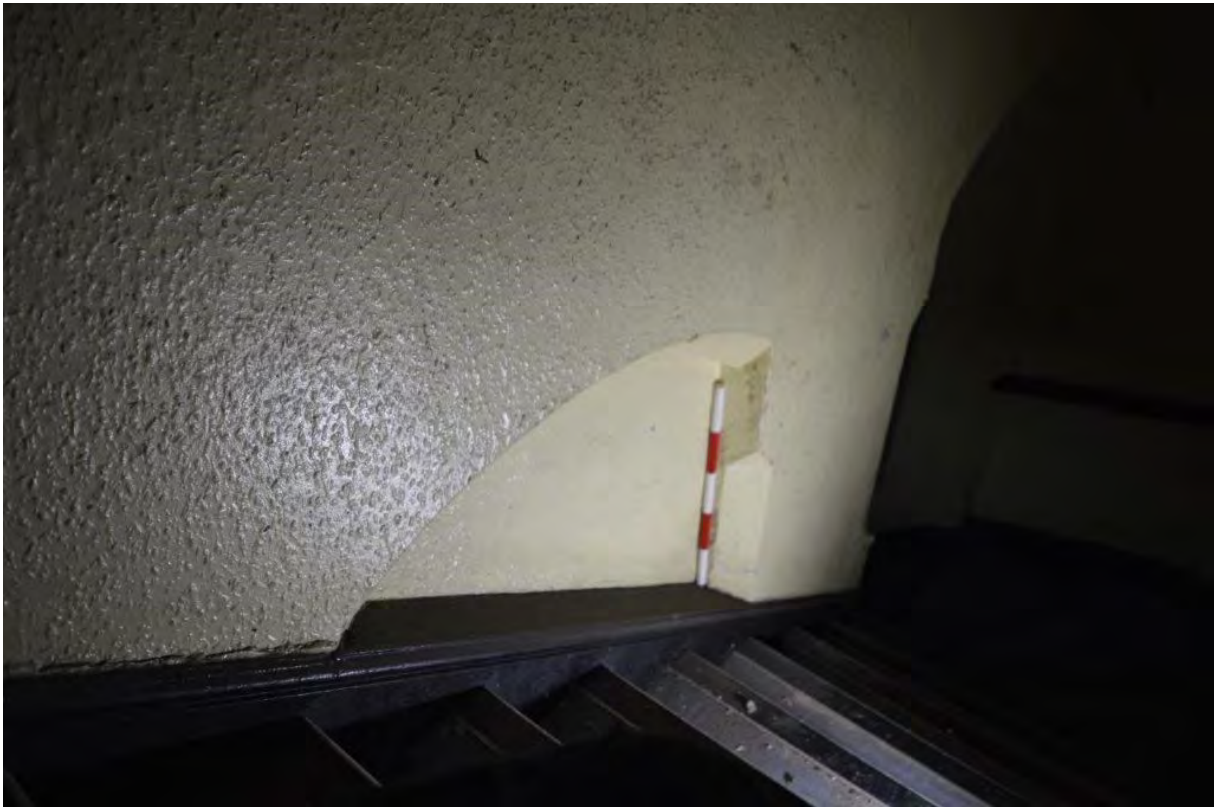
Plate 107. Top of blind arch partially obscured by staircase RF13, view north-east, scale 0.5m
