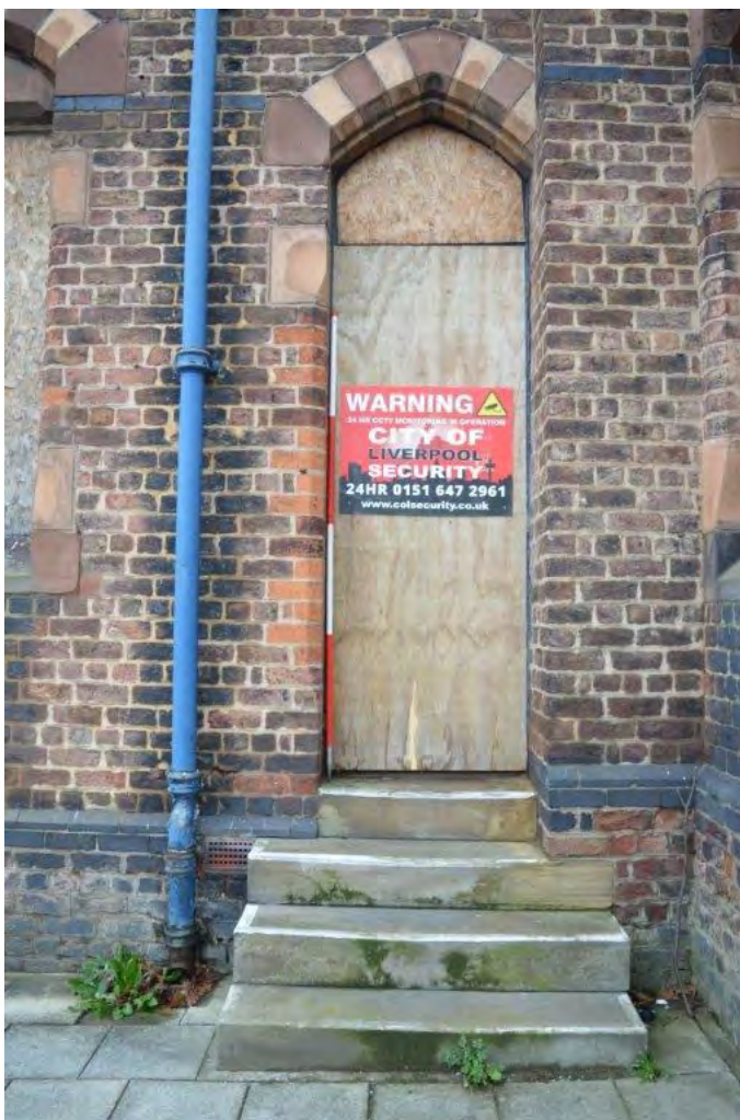
Plate 10. Narrow doorway in front elevation of building, view north, scale 2m
