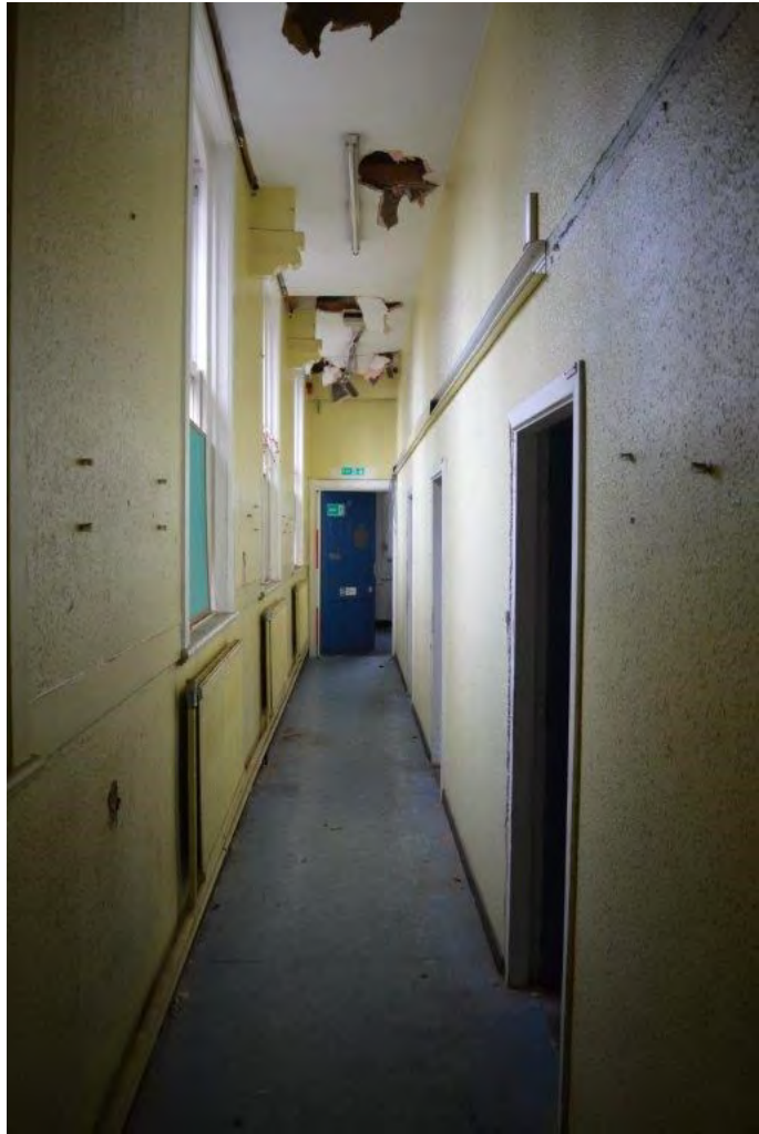
Plate 109. Corridor to west side of courtroom wing (part of RF02), view north
