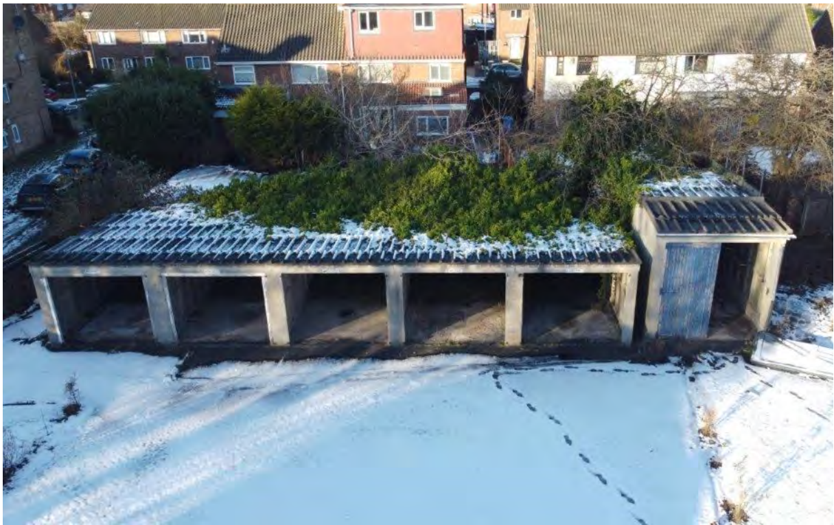
Plate 139. Low level aerial view of Buildings H (garages) and I (maintenance shed), view NNW
