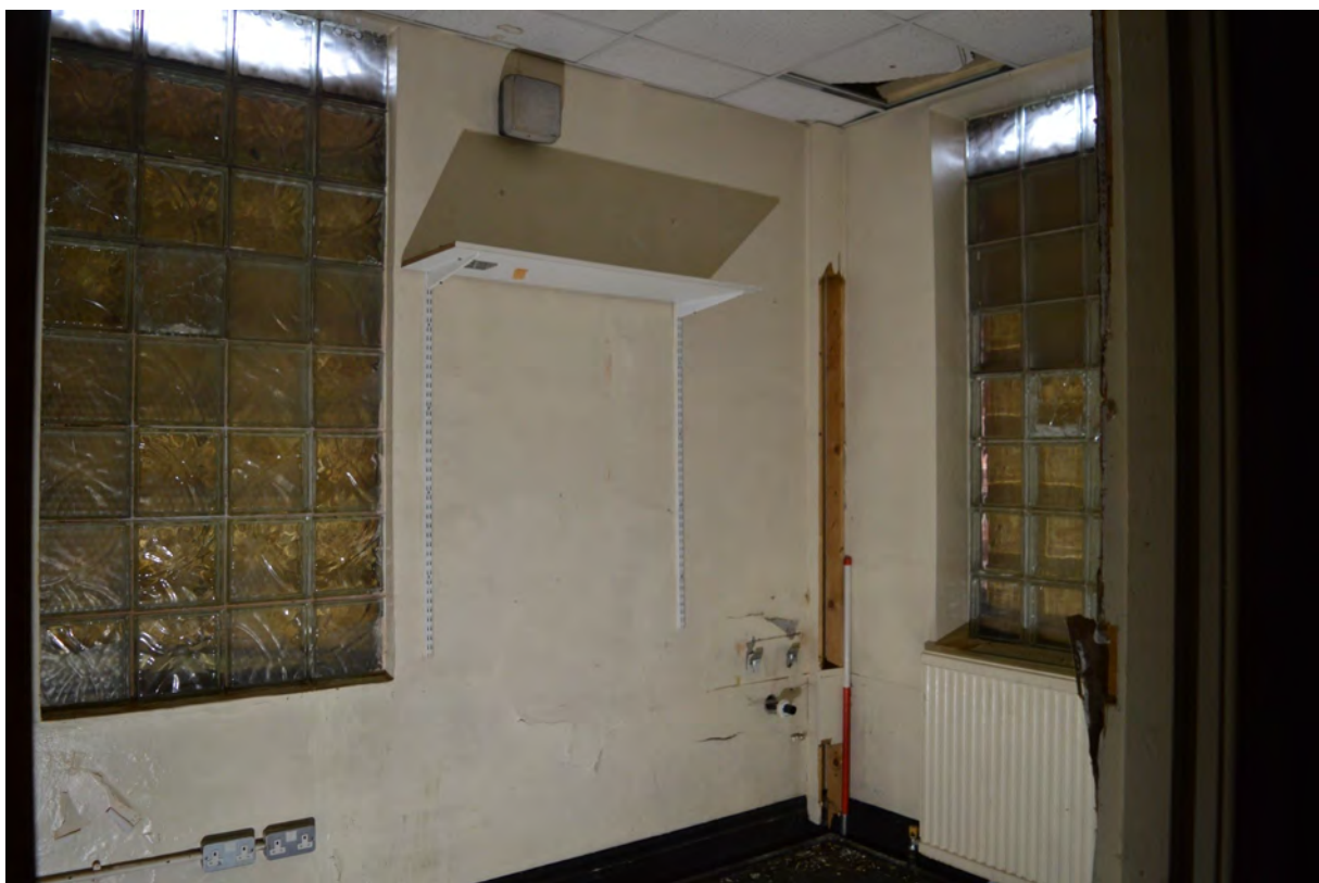
Plate 72. View north-east in former kitchen RG22, scale 1m
