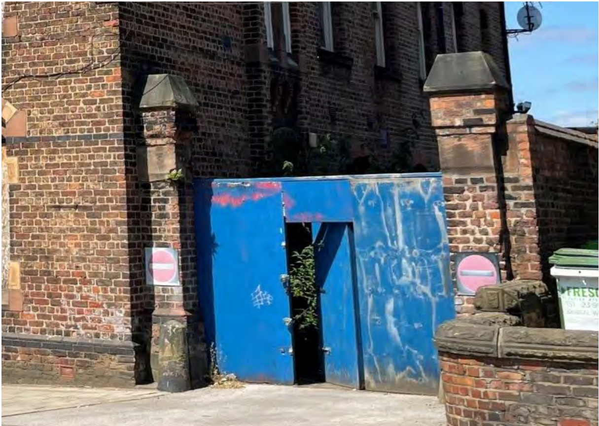
Plate 5. Gate piers at Derby Street., view north-west
