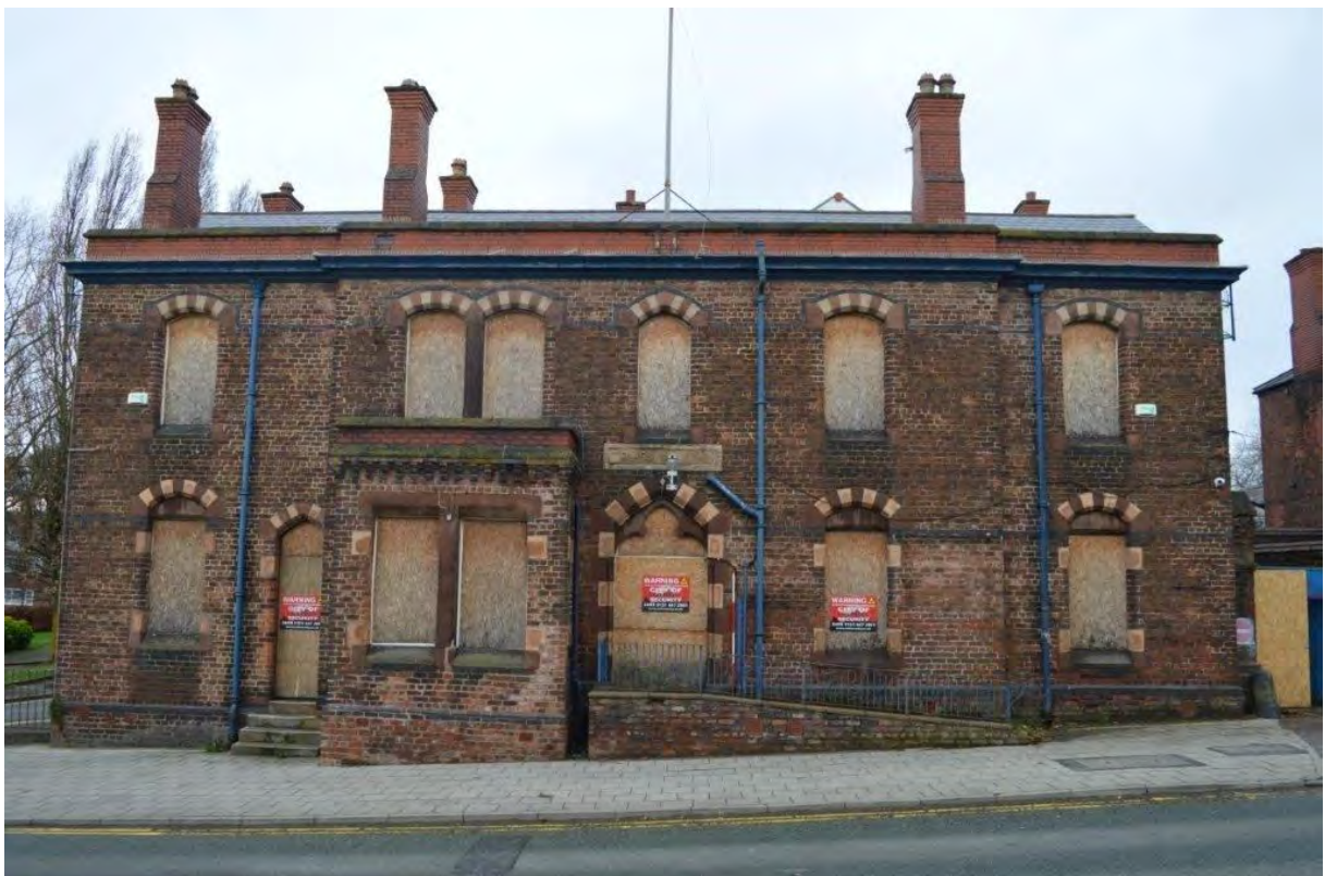
Plate 8. South facing elevation of police station, view north, scale 2m
