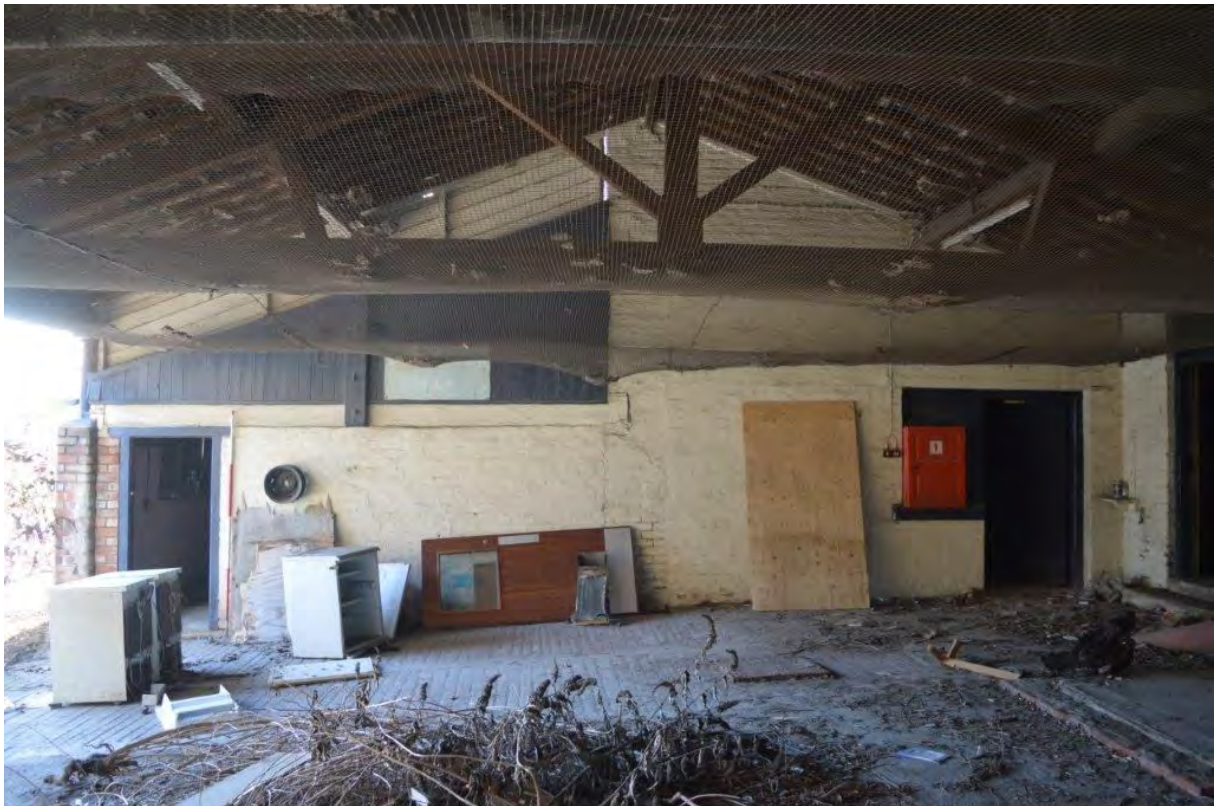
Plate 126. Interior of Building C, view north
