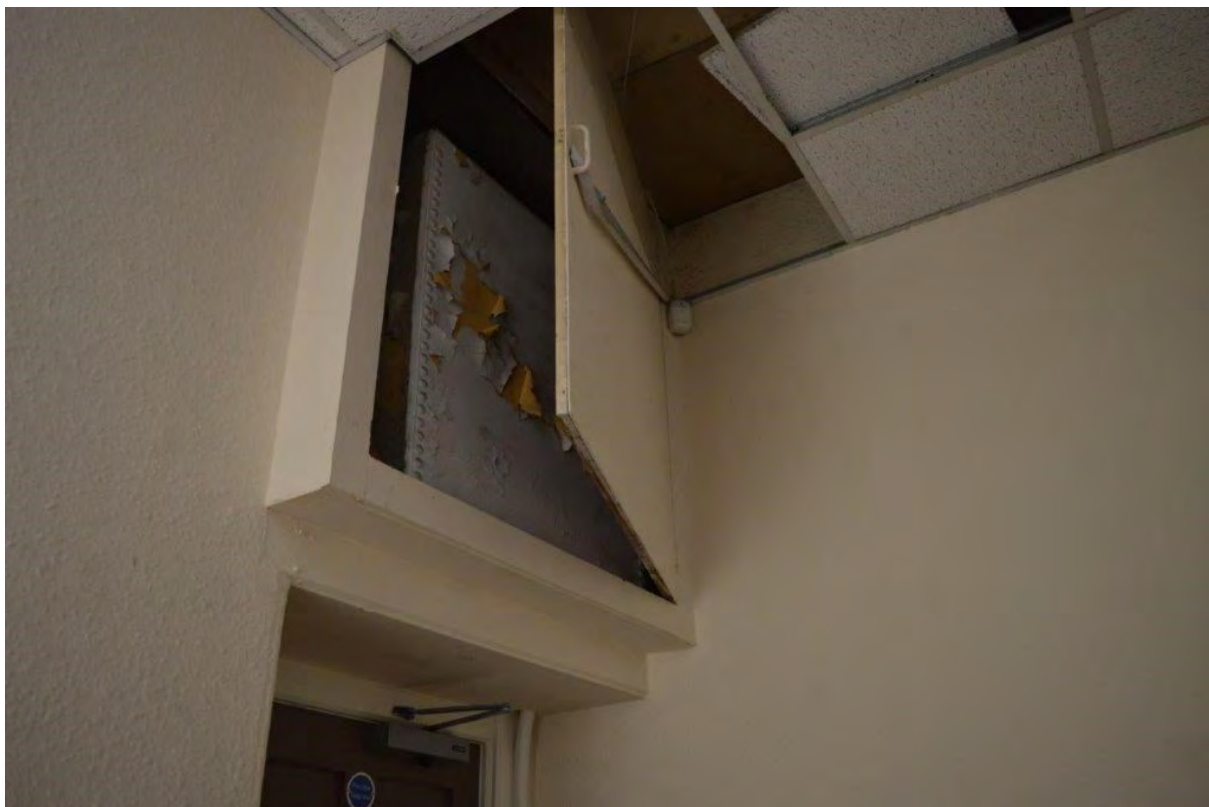
Plate 91. Cupboard to header tank above door to RF03, view north-west
