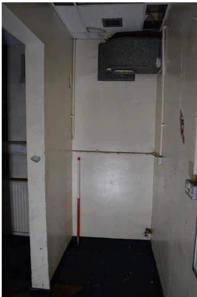
Plate 69. View east in alcove toward blocked door, scale 1m
