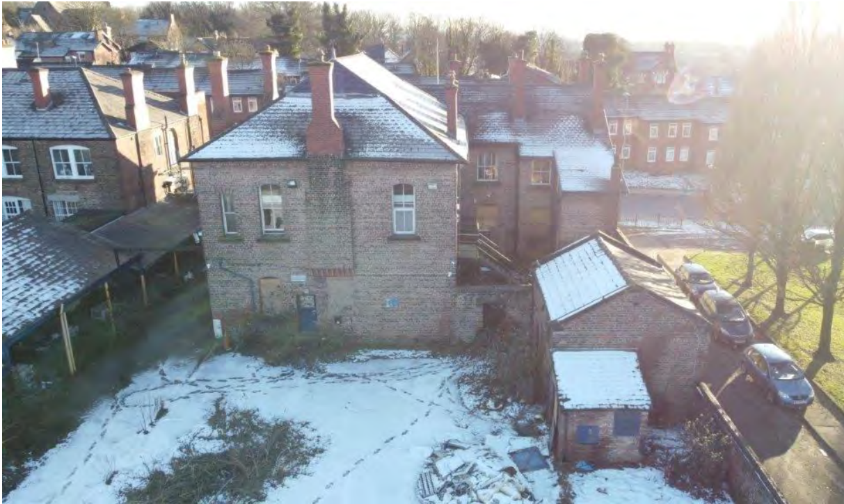
Plate 3. Low level aerial view of rear of building, view south
