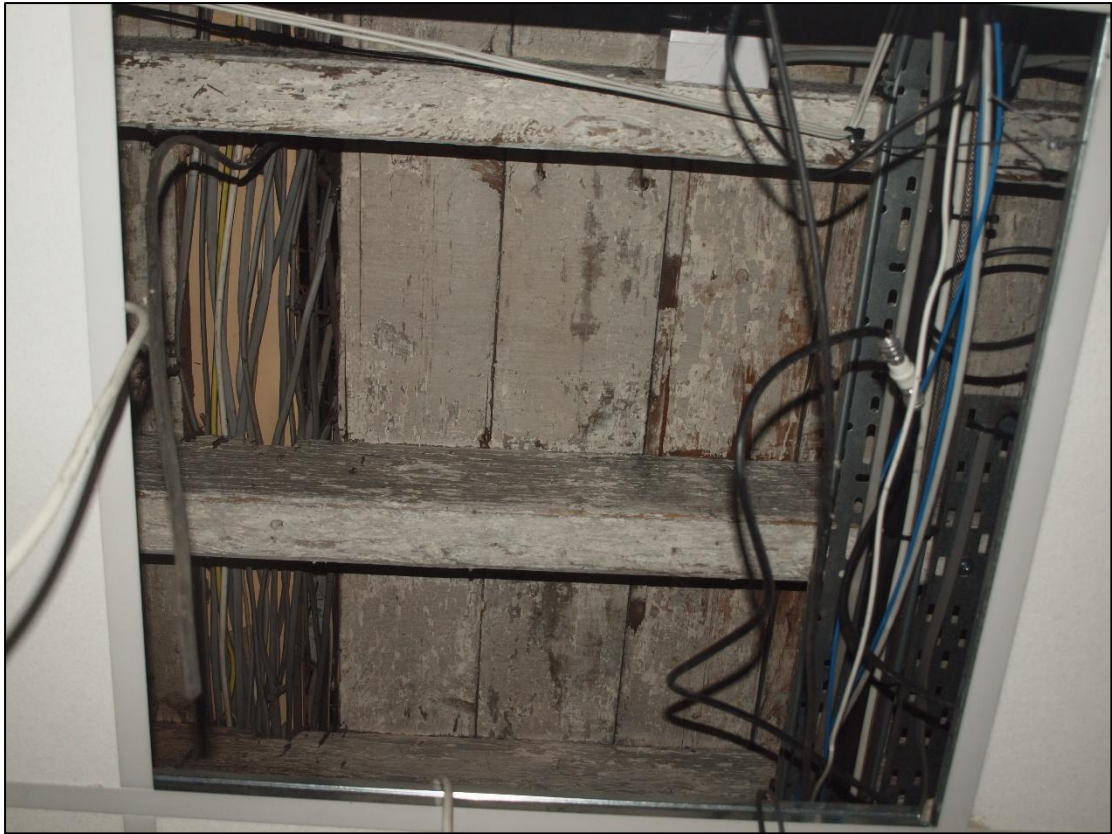
Plate 35: Timber beams and boards of first floor
