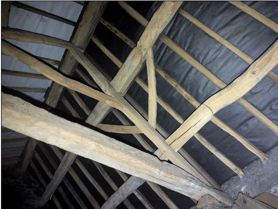
Plate 37: Detail of above showing wind braces
