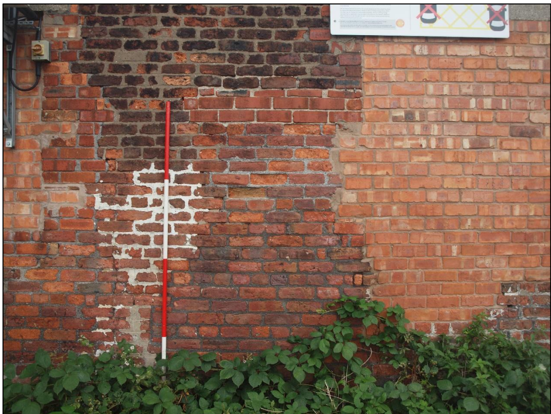
Plate 18: Blocked doorway south of blocked window
