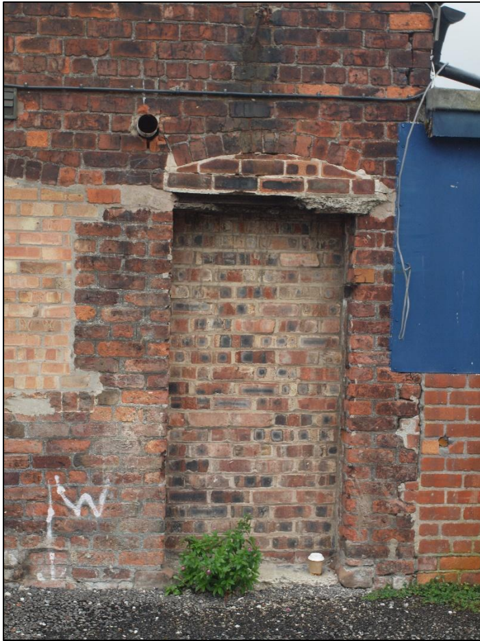
Plate 11: Detail of blocked doorway
