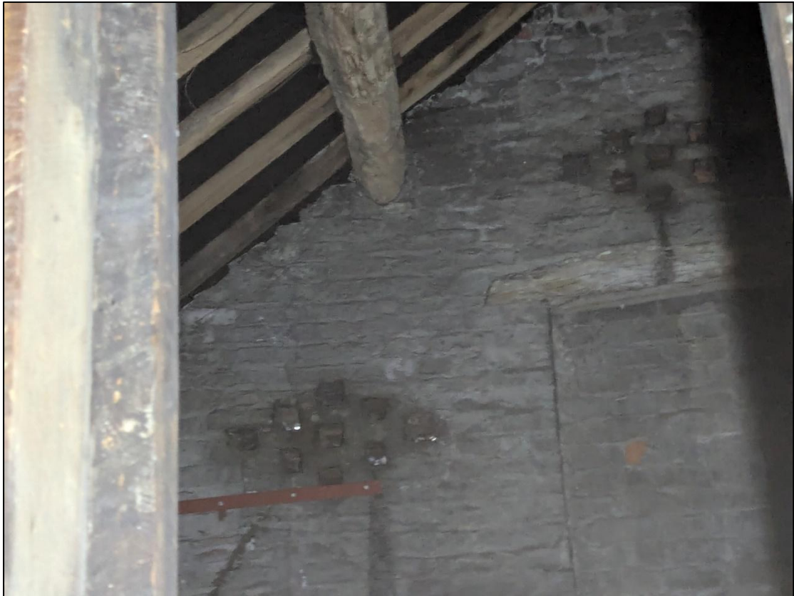
Plate 41: Northern gable showing blocked pitching window and ventilation slots
