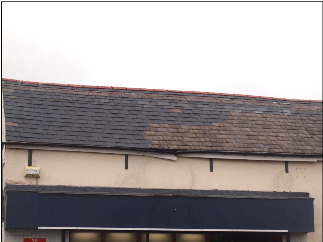
Plate 4: East elevation showing ghost of blocked pitching eye and roof
