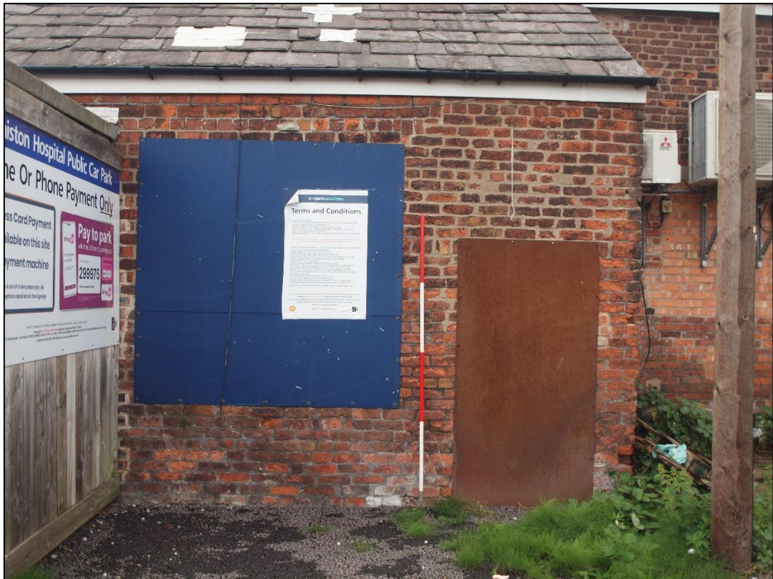
Plate 15: West elevation of lean-to showing blocked doorway
