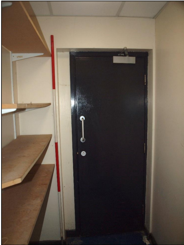
Plate 33: Doorway to modern lean-to WC
