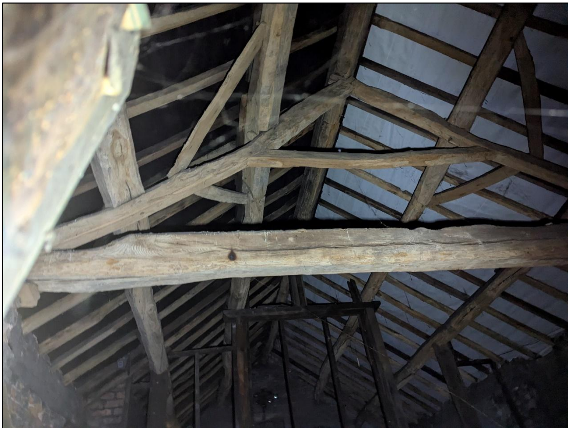
Plate 36: First floor showing truss with timber partition beyond
