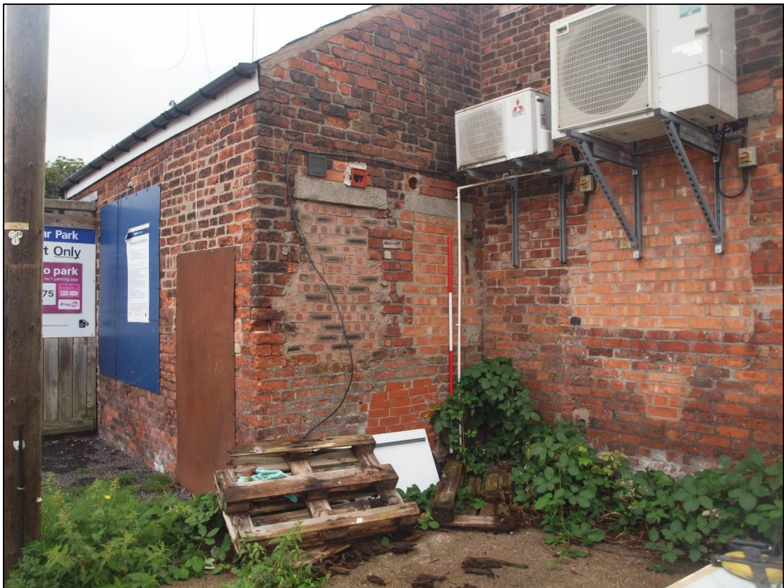
Plate 24: South elevation of lean-to
