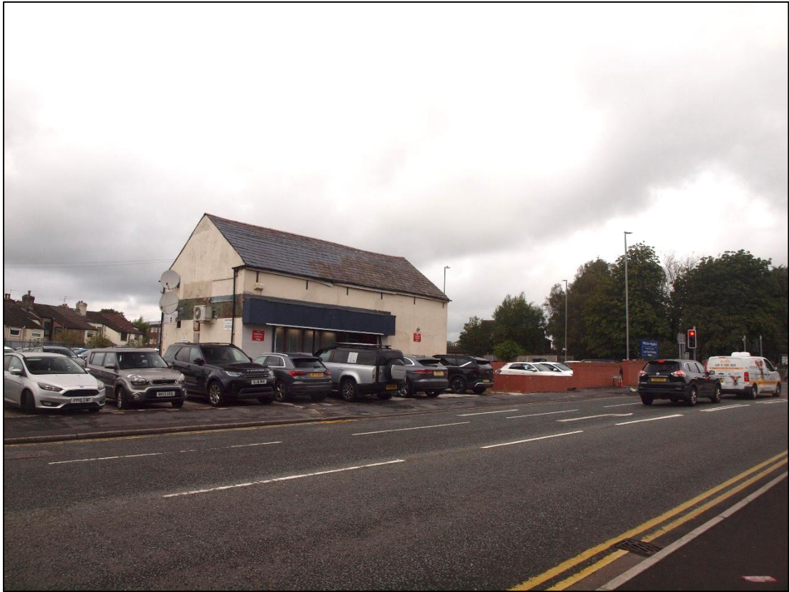
Plate 1: General shot of building
