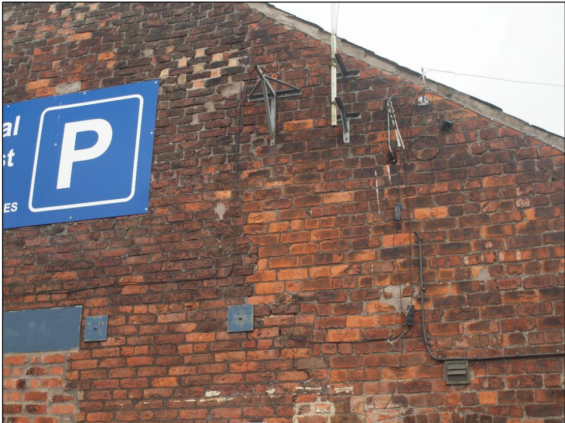
Plate 12: Change of brickwork showing lean-to extension joint
