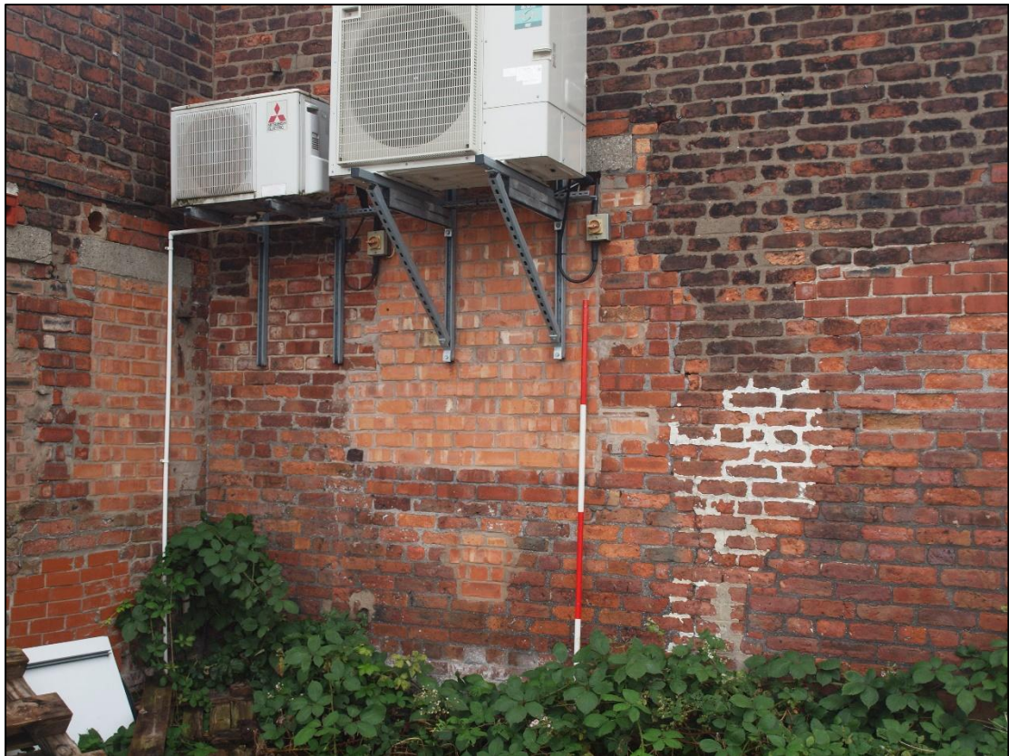
Plate 17: Blocked window with concrete lintel to north end
