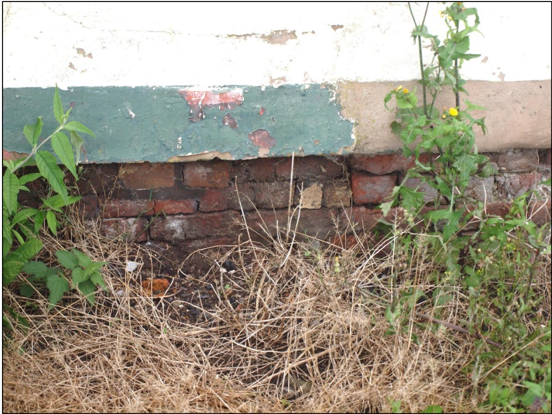
Plate 23: Brickwork visible below render
