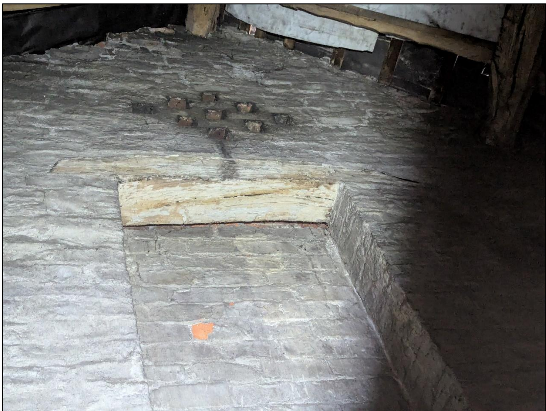
Plate 42: Detail of blocked pitching window and ventilation holes above
