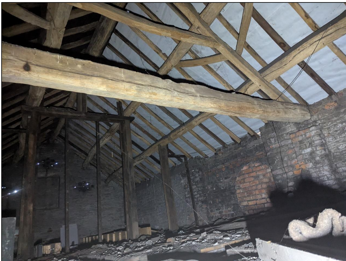
Plate 38: Blocked pitching eye and timber partition
