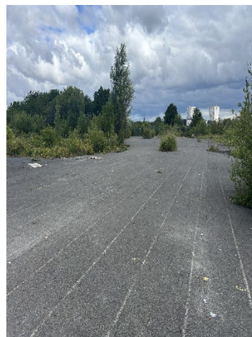
Figure 6 – Hardstanding underlying most of the southern site section.
