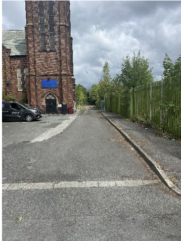
Figure 1 – Site entrance and existing St. Dominic's Church from Southdean road facing north.
