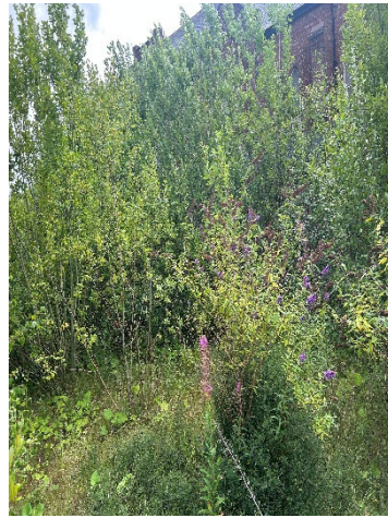
Figure 4 – Area of the former club with dense vegetation underlain by hardstanding.
