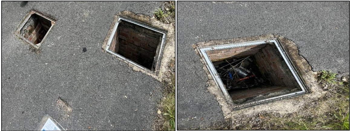
Figure 6: Photograph showing the uncovered manholes in the southern site section
