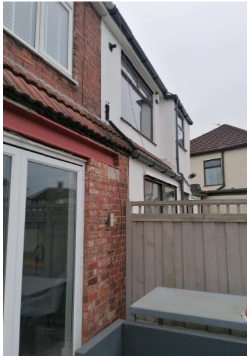
Boundary with No. 15 Windsor Road
