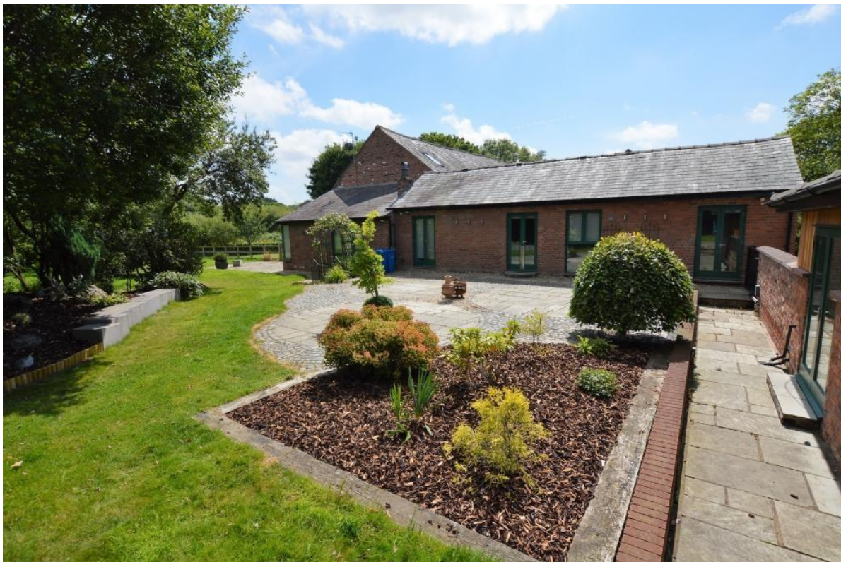
Fig.1 North facing elevation of Shippon 1 viewed from patio area
