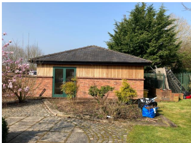
Fig.13 Gable end of Garage/Utility Room to patio
