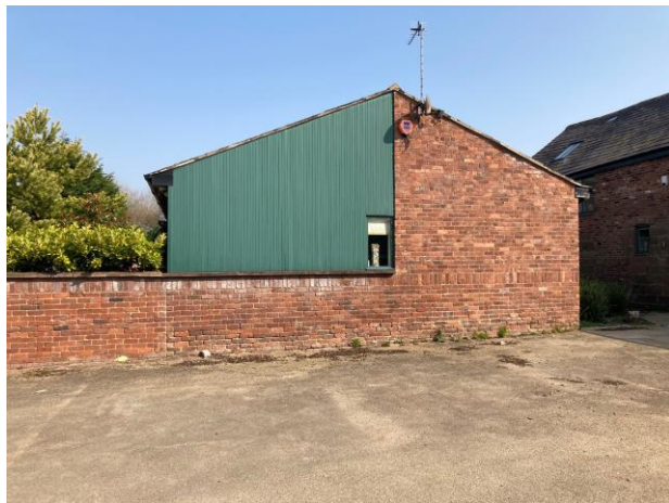
Fig.11 Brick & Timber South gable end to Shippon 1
