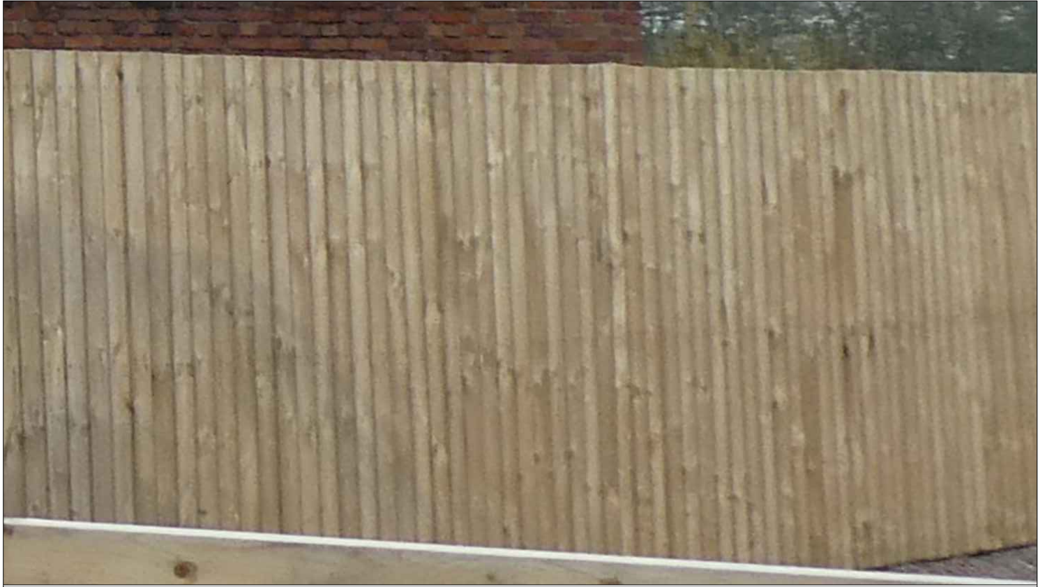
PHOTOGRAPHS OF EXISTING 2.0m HIGH TIMBER FENCE TO FORM NEW CENTRE BOUNDARY WALL BETWEEN (NTS)
