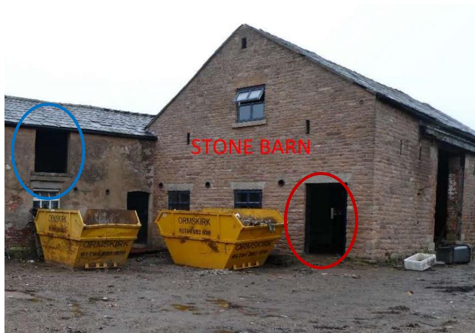
Figure 5.4 – Visual Aid – Emergence location of Brown Long-eared bat on first survey from open door on southern elevation of Stone Barn A (red circle) and barn owl from hay loft on eastern elevation of Stone Barn B (blue circle)
