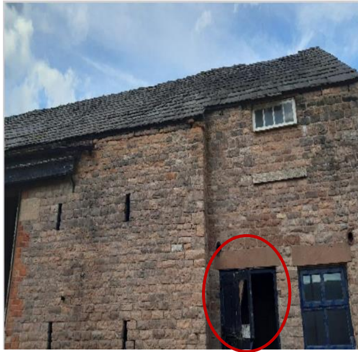
Figure 5.3 – Visual Aid – Emergence location of three Common Pipistrelle on both surveys from open door on eastern elevation of Stone Barn A
