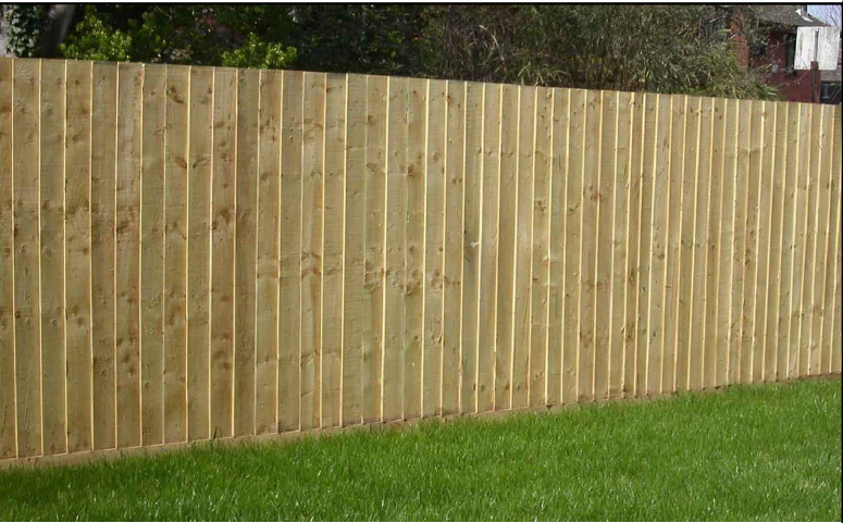
Close Boarded Timber Fence
