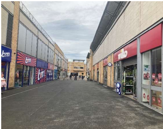
Photograph 13: Pedestrian Conditions within Huyton town centre
