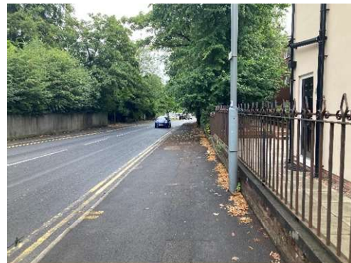
Photograph 6: Pedestrian footway conditions headed eastbound along Huyton Lane
