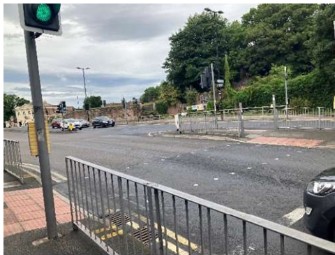
Photograph 9: Pedestrian Signalised Crossing at Huyton Lane viewing westbound
