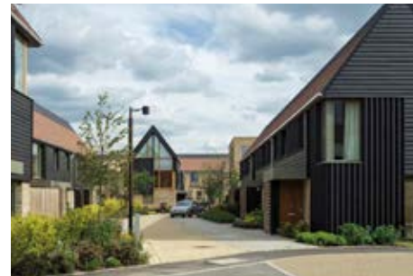
① Timber to First Floor Accommodation
