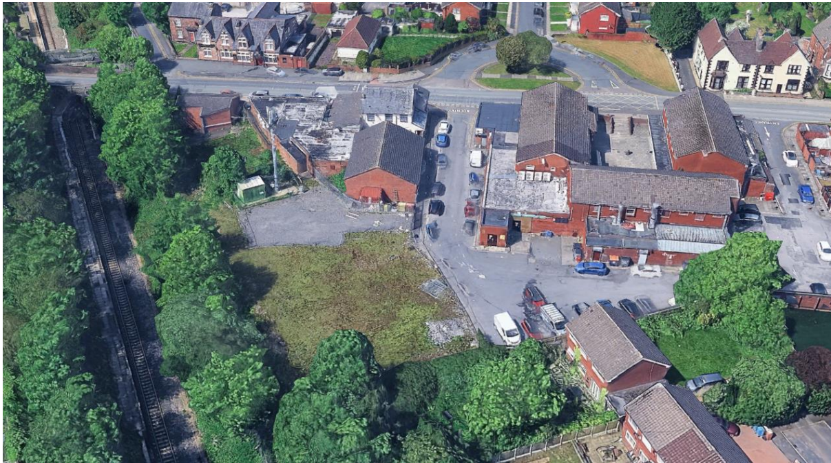
Aerial Image of the site (Source: Google Earth)
