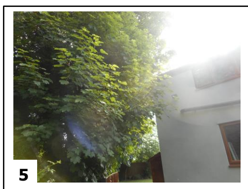
Photo 5: A view of the sycamores overhanging the gable and rear of the Coach House.
