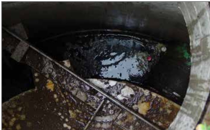
Fig. 8 View of outer annulus of floatables and oil collection zone.
