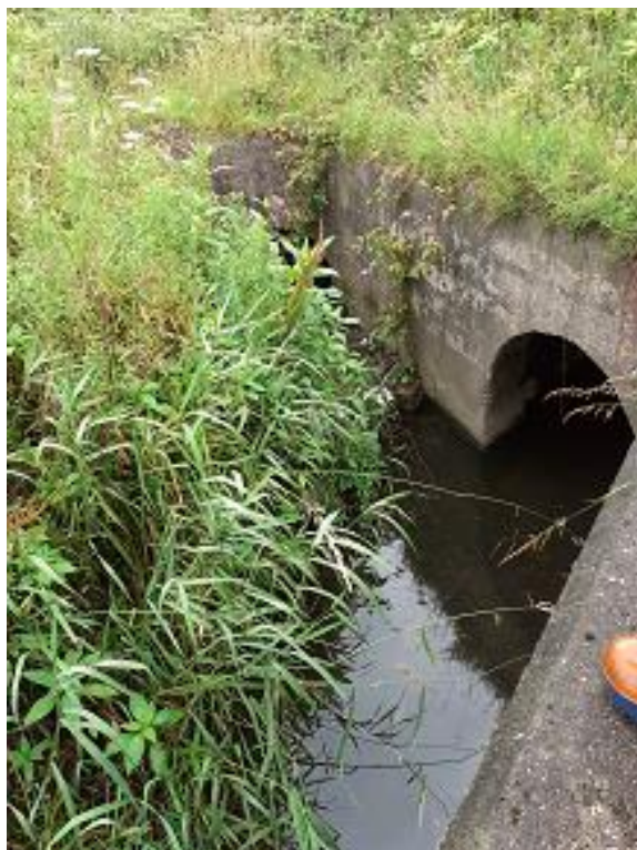
Photograph 3. Slow-flowing culverted stream (TN2) – Kirkby Brook which runs through the proposed Headbolt Lane station site.
