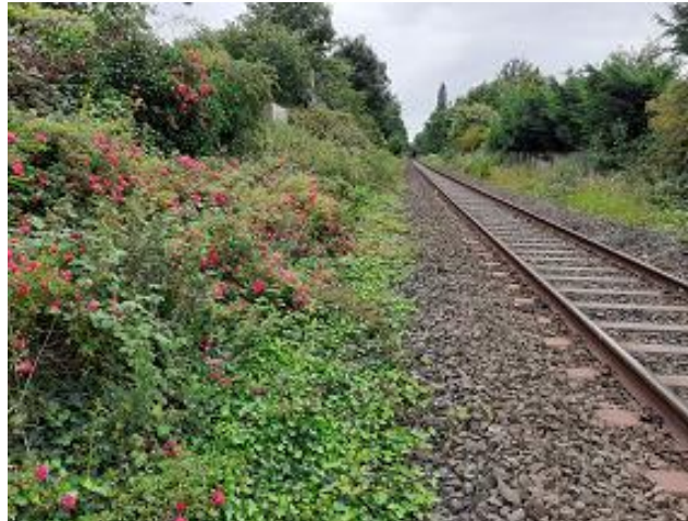
Photograph 12. Embankment vegetation (TN15), large numbers of garden escape shrubs are present between Kirkby Station and the Mill Brook crossing (bridge 56).
