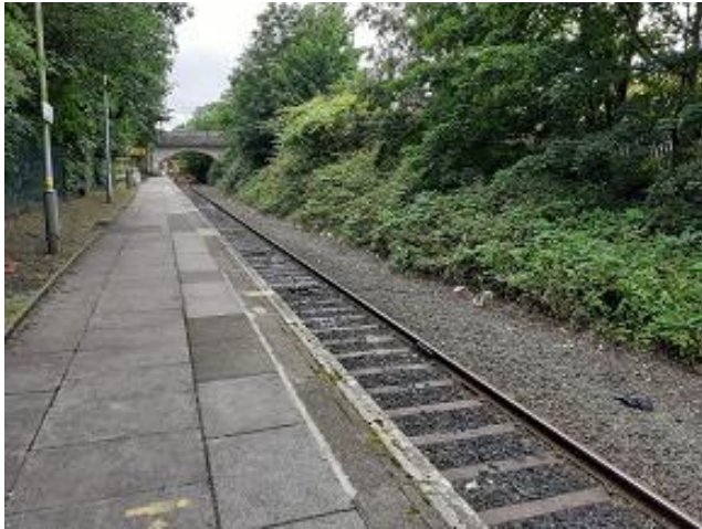
Photograph 11. Northern platform of Kirkby (TN15), with bankside vegetation opposite including Japanese knotweed at base of bare ground for substation (TN13).
