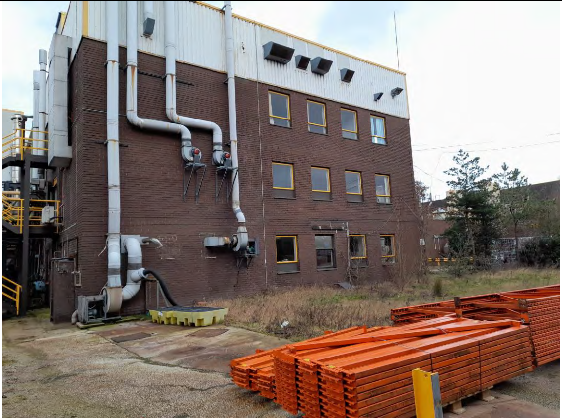
A15.1 View of the TDC building from the south
