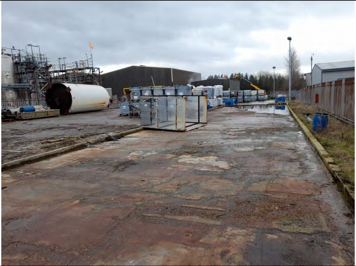
A19.1 View of the bunded storage area along the western side of the site
