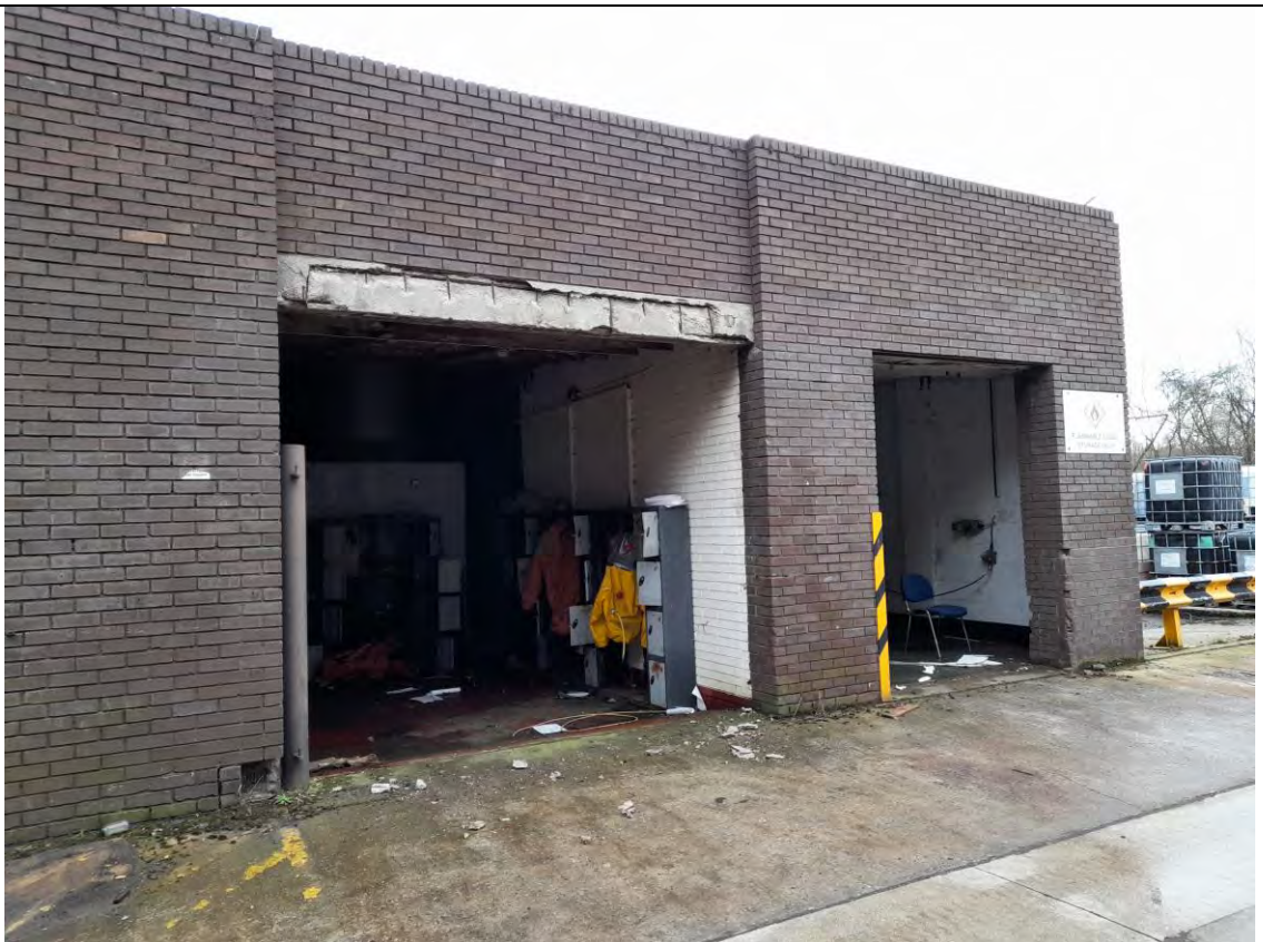
A14.1. View of the dryer house from the north west
