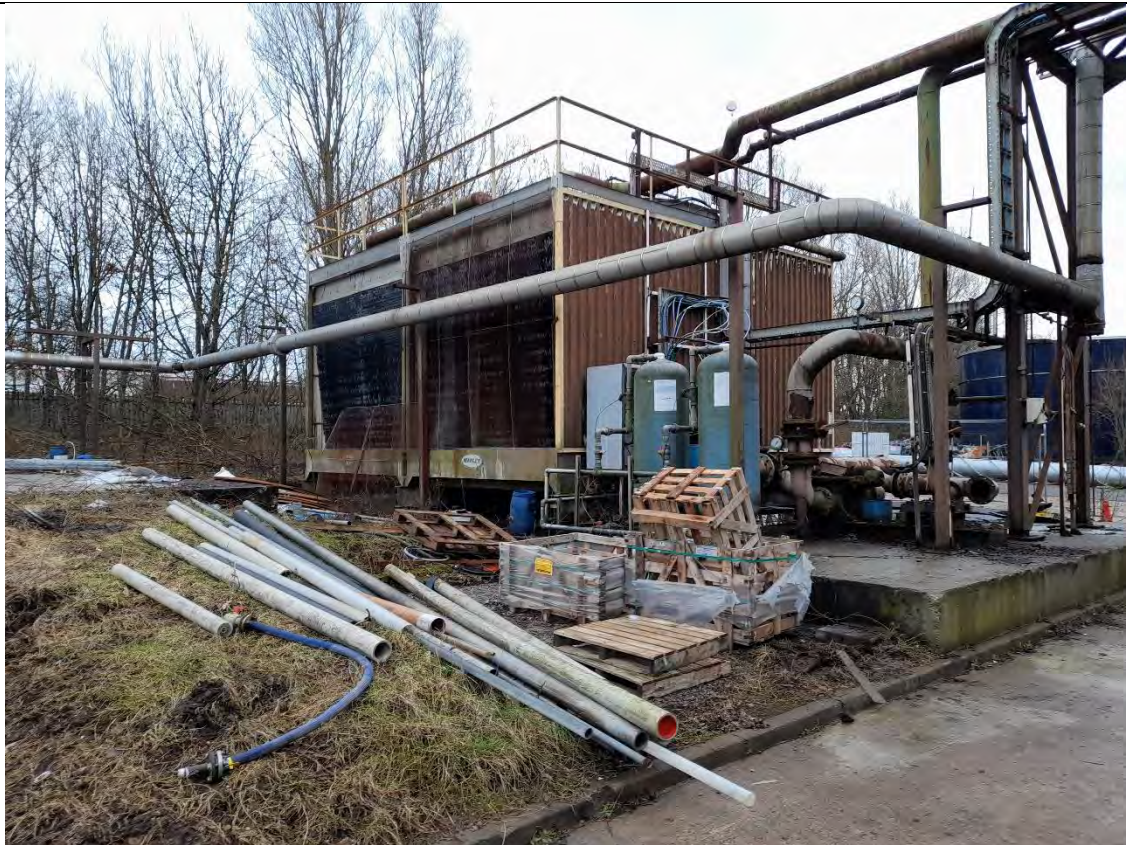
A3.1. View of the cooling tower along the northern boundary of the site
