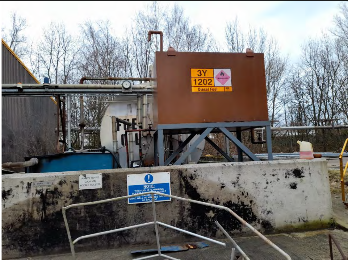
A6.1. View of the fuel tanks along the northern boundary of the site
