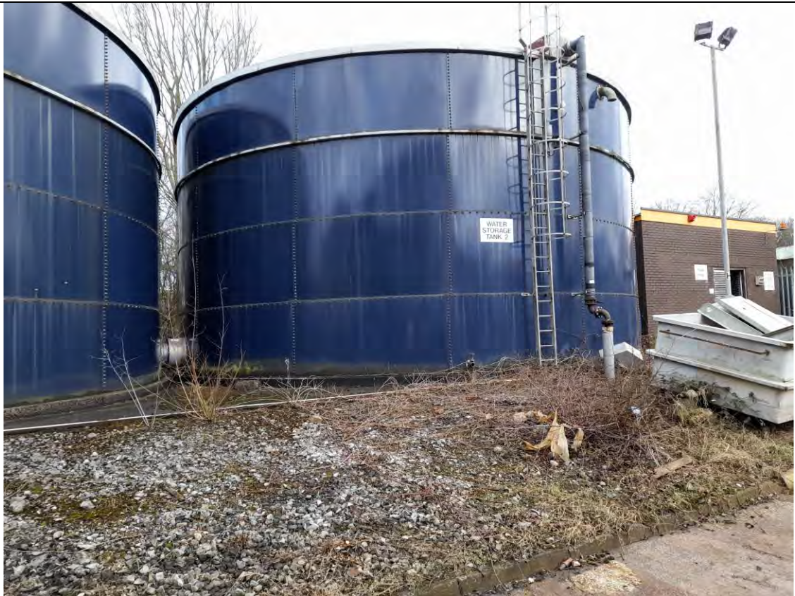
A2.1. View of water tanks from the south west
