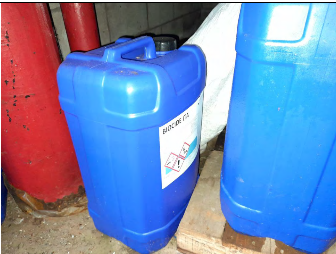
A1.4. Chemicals within the pump house
