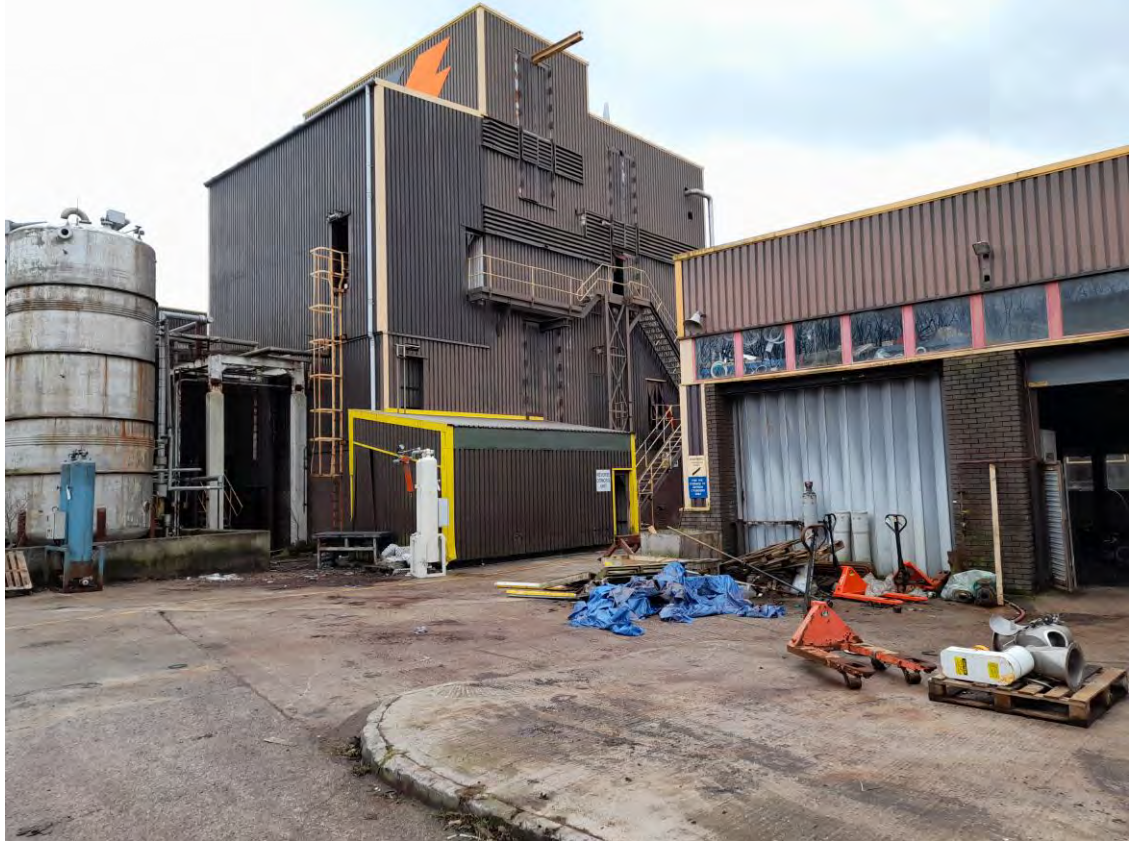
A17.1 View of the Diol Plant from the North west
