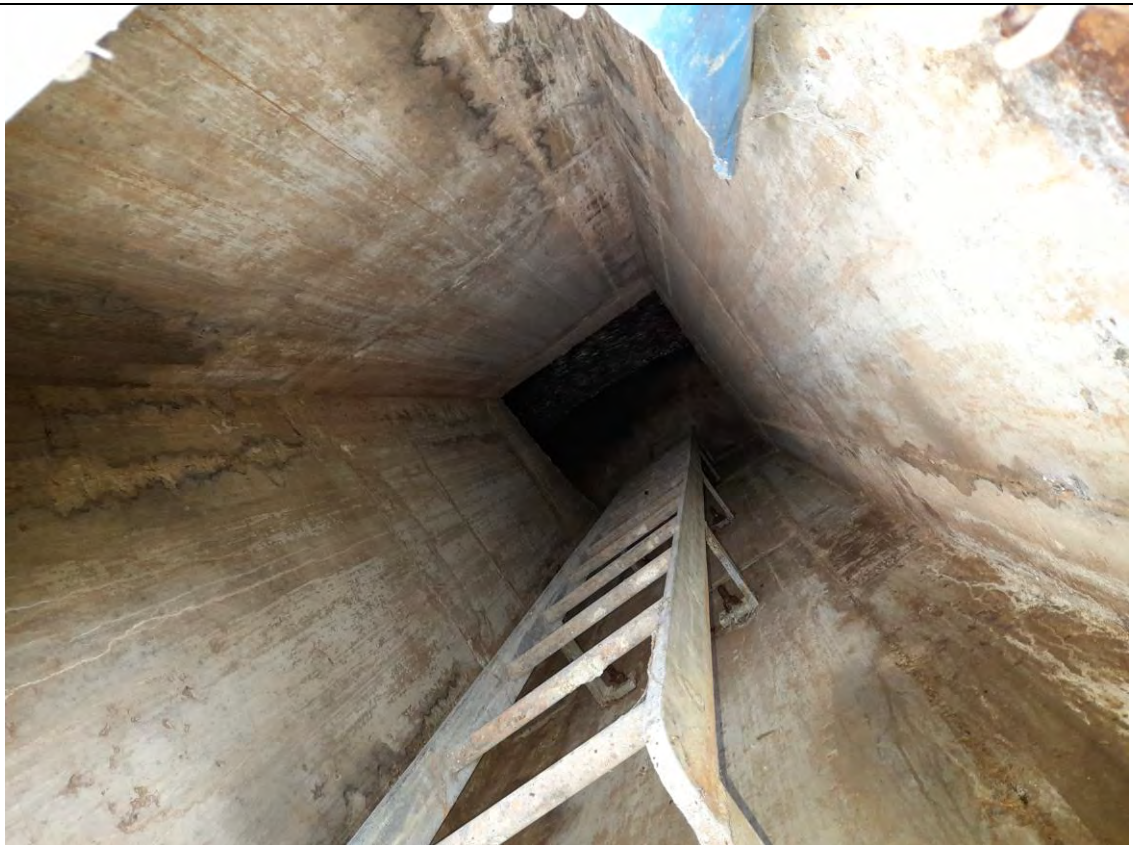
View within the culvert
