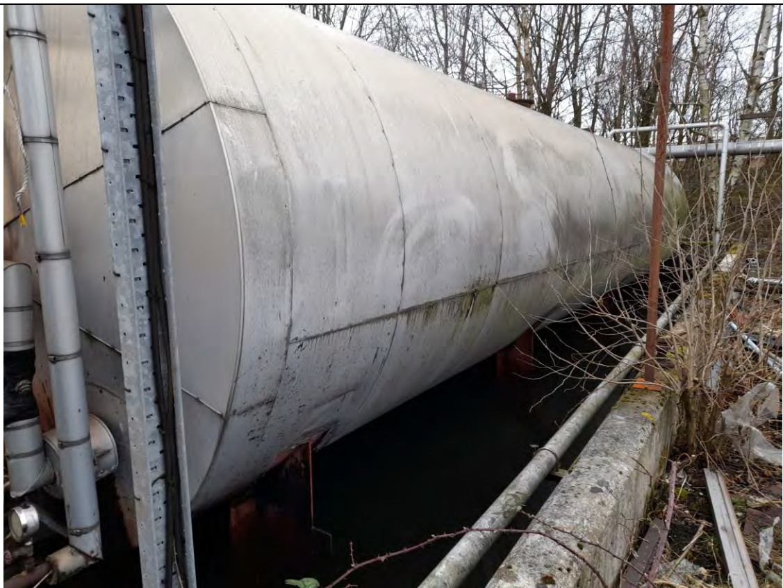
A6.2. View of the fuel tanks along the northern boundary of the site
