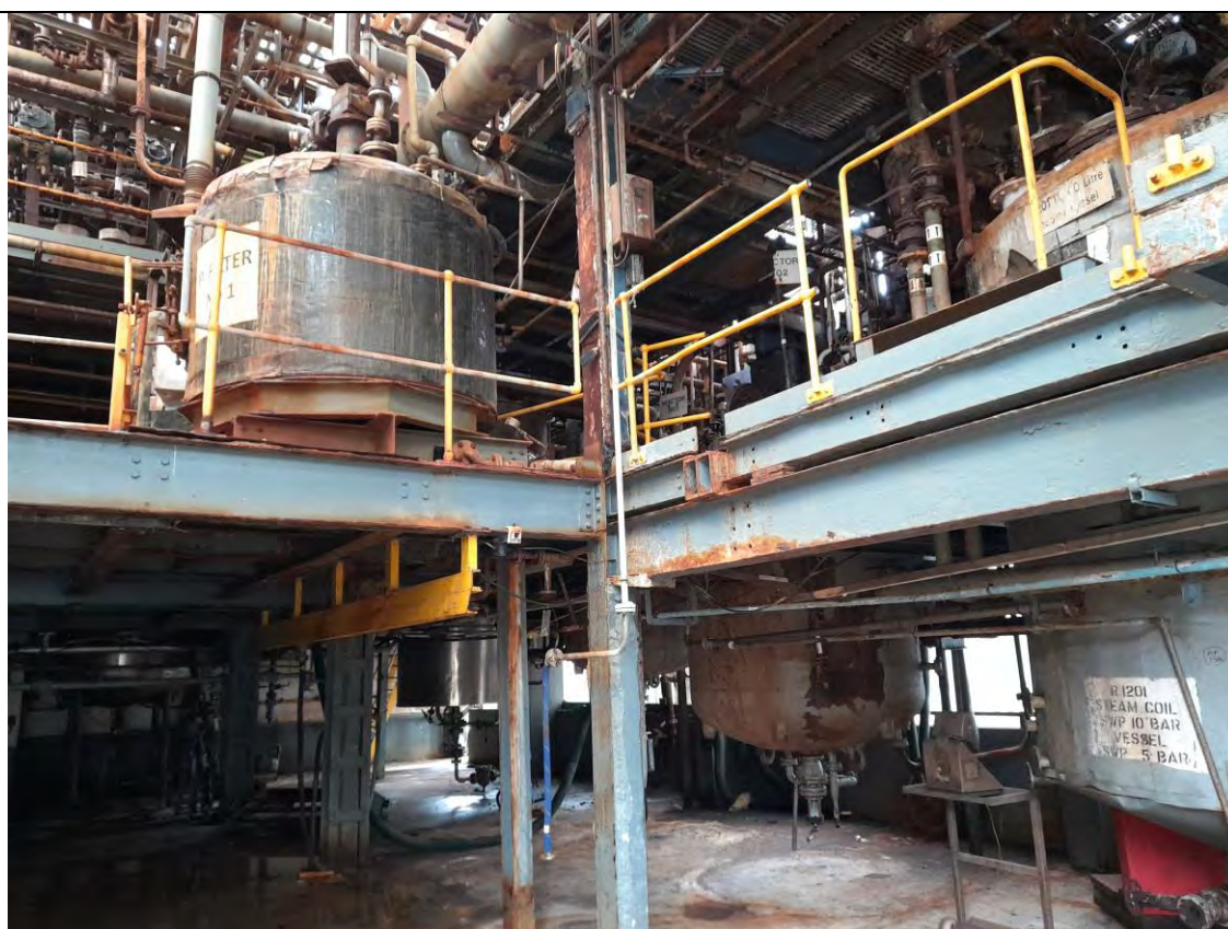
A15.4. View of inside the TDC building
