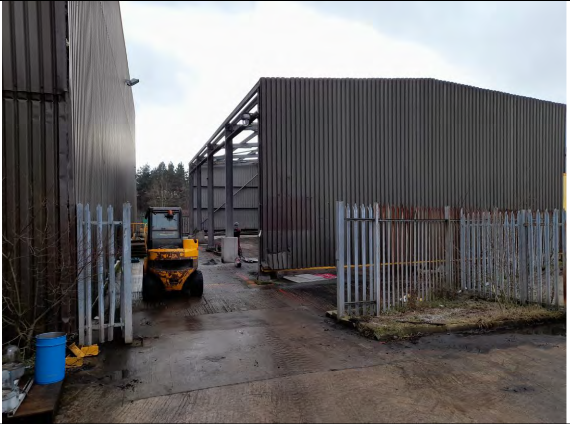
A11.1 View of the flammable store from the north
