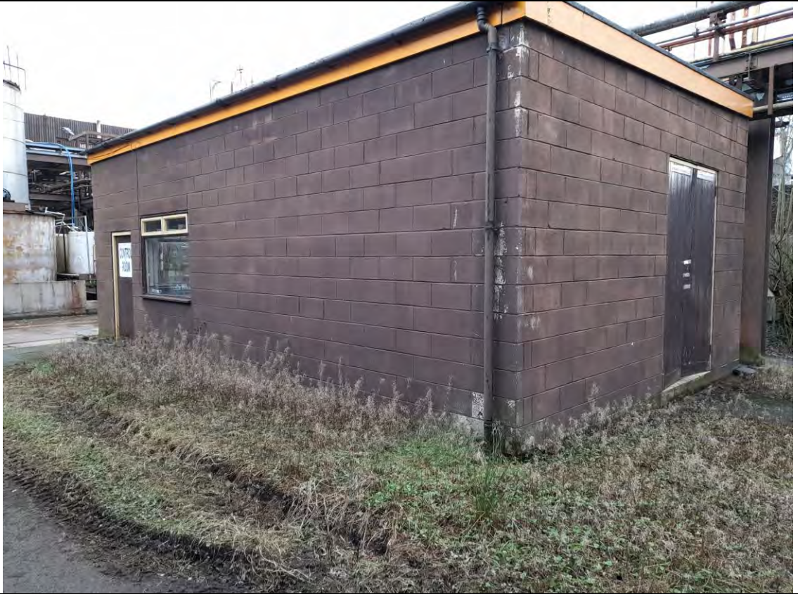
A13.1 View of the switch room from the north west
