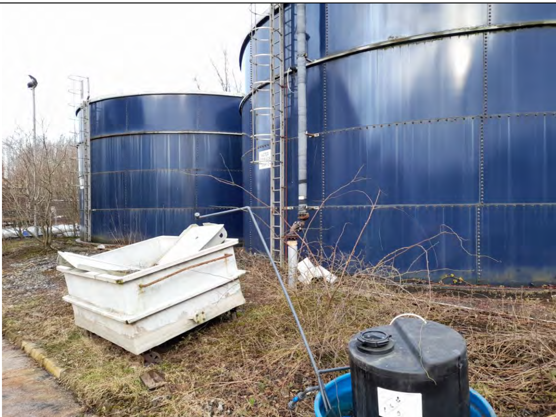
A2.2. View of water tanks from the south east
