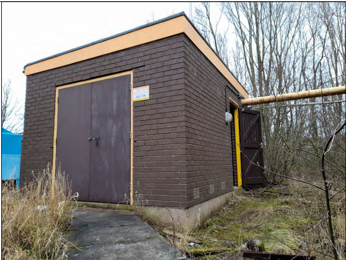
A8.1. View of the Valve house
