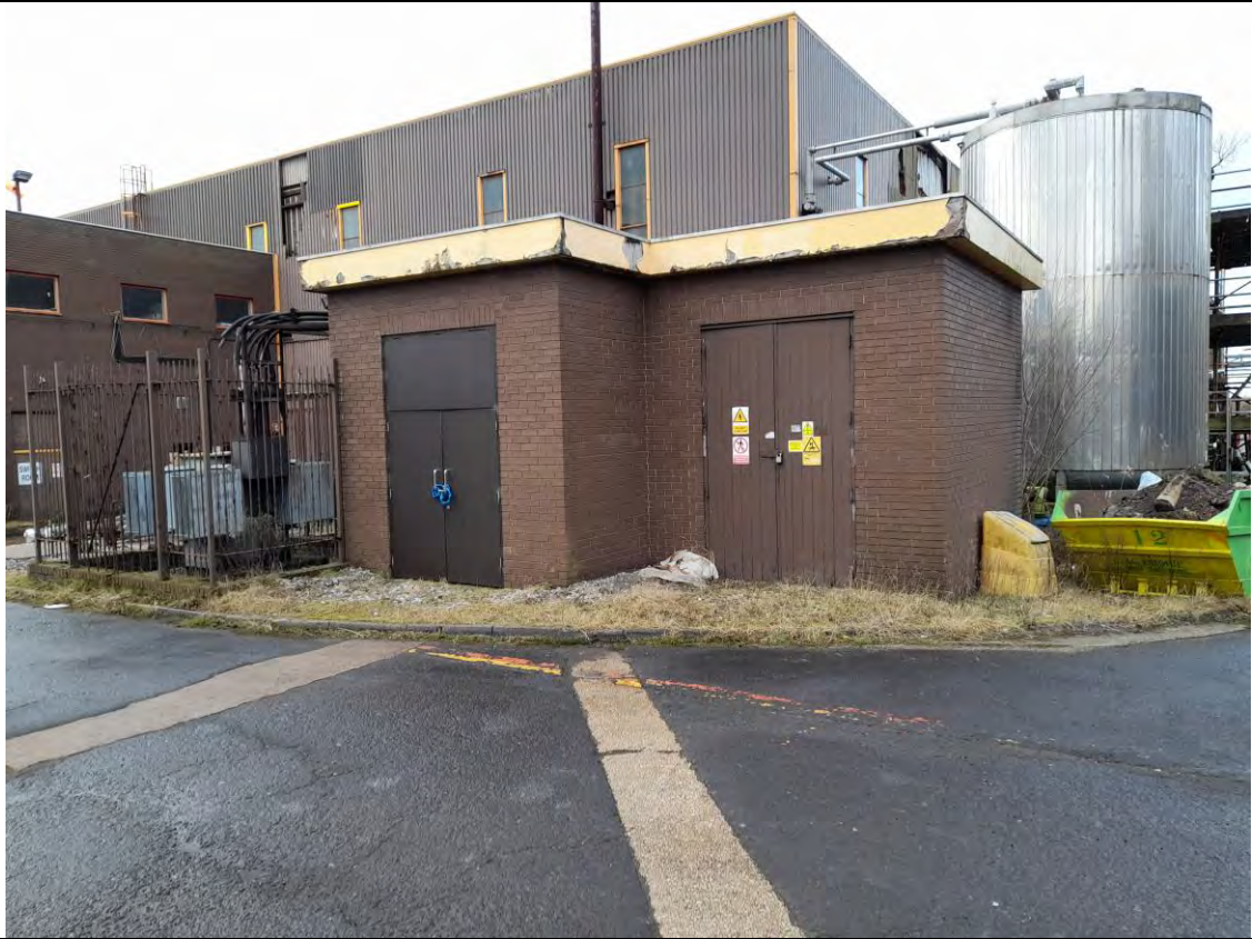
A20.1. View of the Electricity substation structure from the North east
