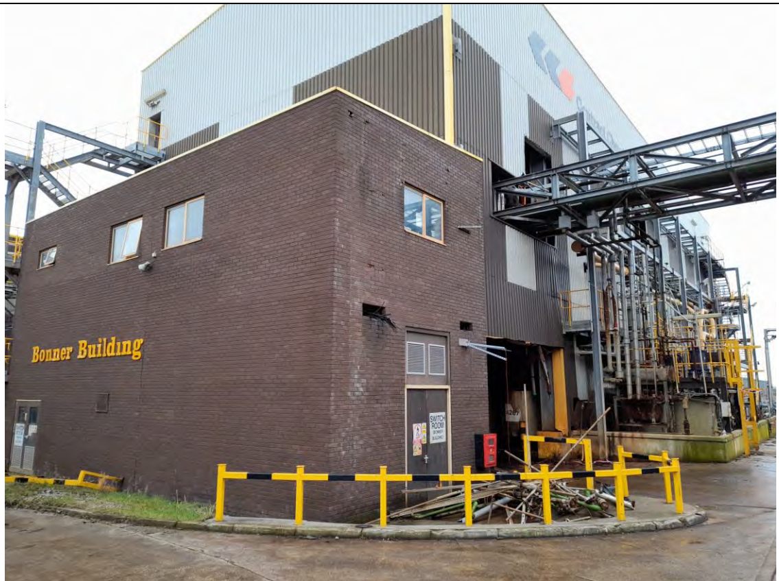
A16.1 View of the Bonner Building from the north east
