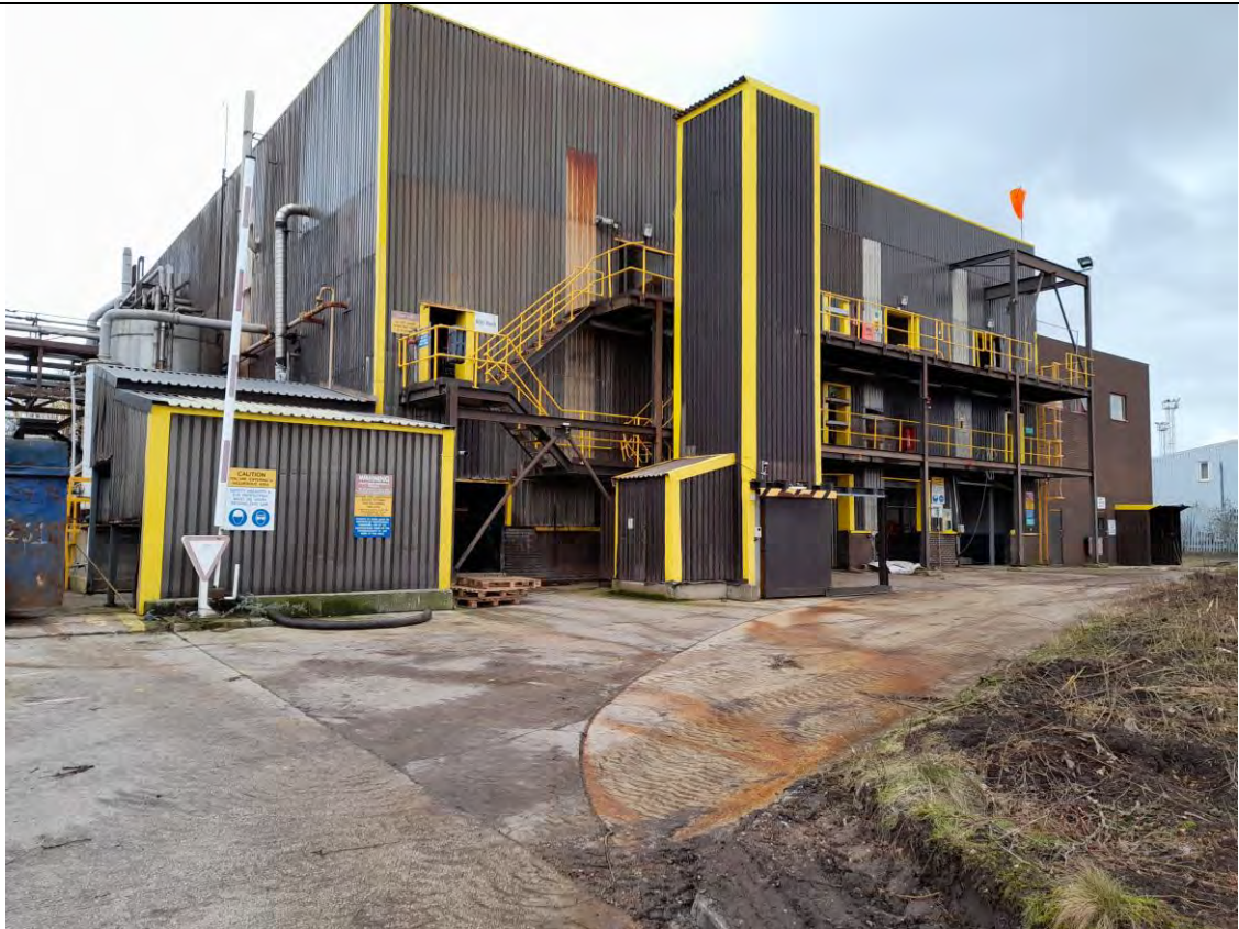
A5.1. View of the Surfactant building from the south
