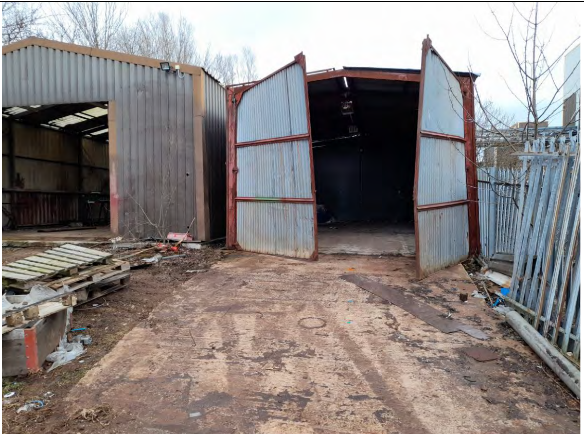
A9.2. View of the workshop sheds
