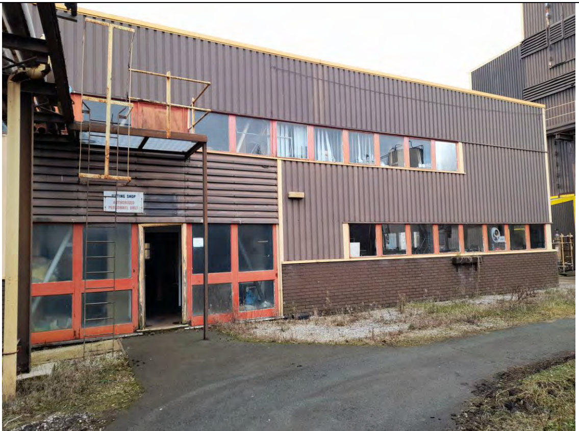
A12.1. View of fitters shop from the south
