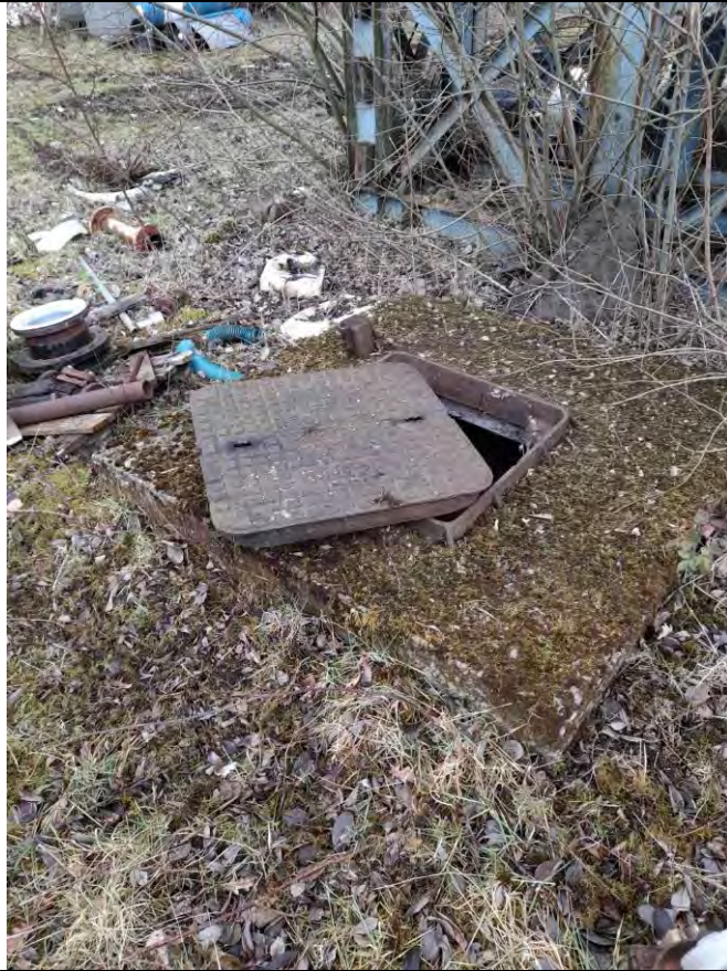
View of the drain above the culverted Knowsley Brook, picture taken from the north western corner of site
