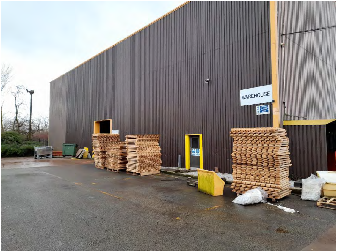
A18.1 View of the warehouse entrance from the north east
