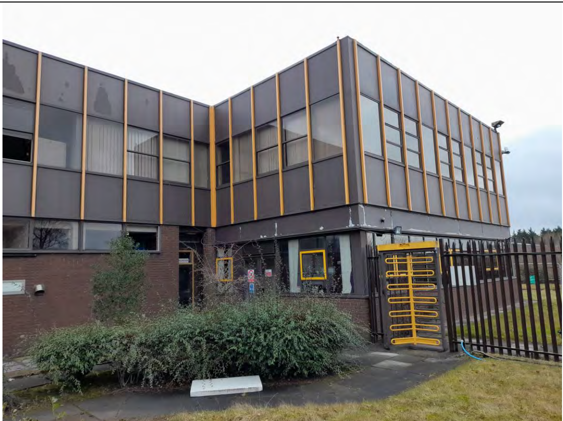
A4.2. View of the office building from the site entrance
