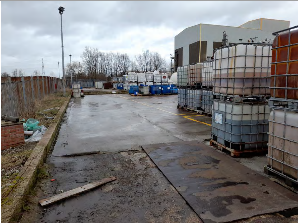
A19.3 View from the south of the storage area
