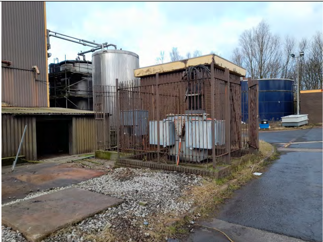
A20.2. View of the Electricity substation structure from the South east
