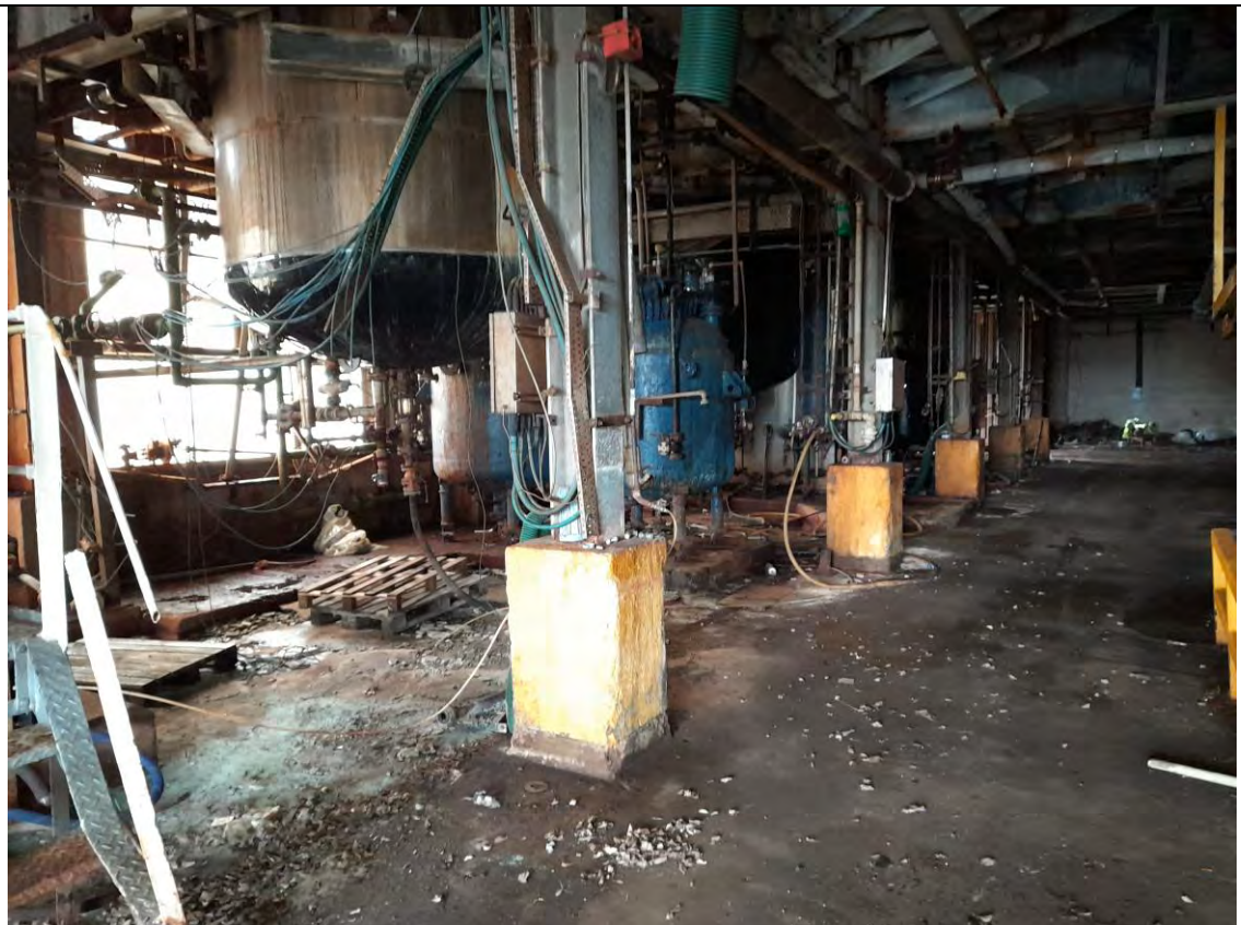
A16.2. View inside of the Bonner building
