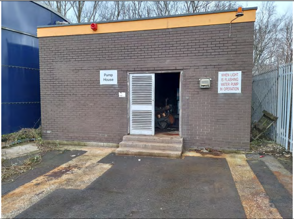
A1.1. View of Pump House building
