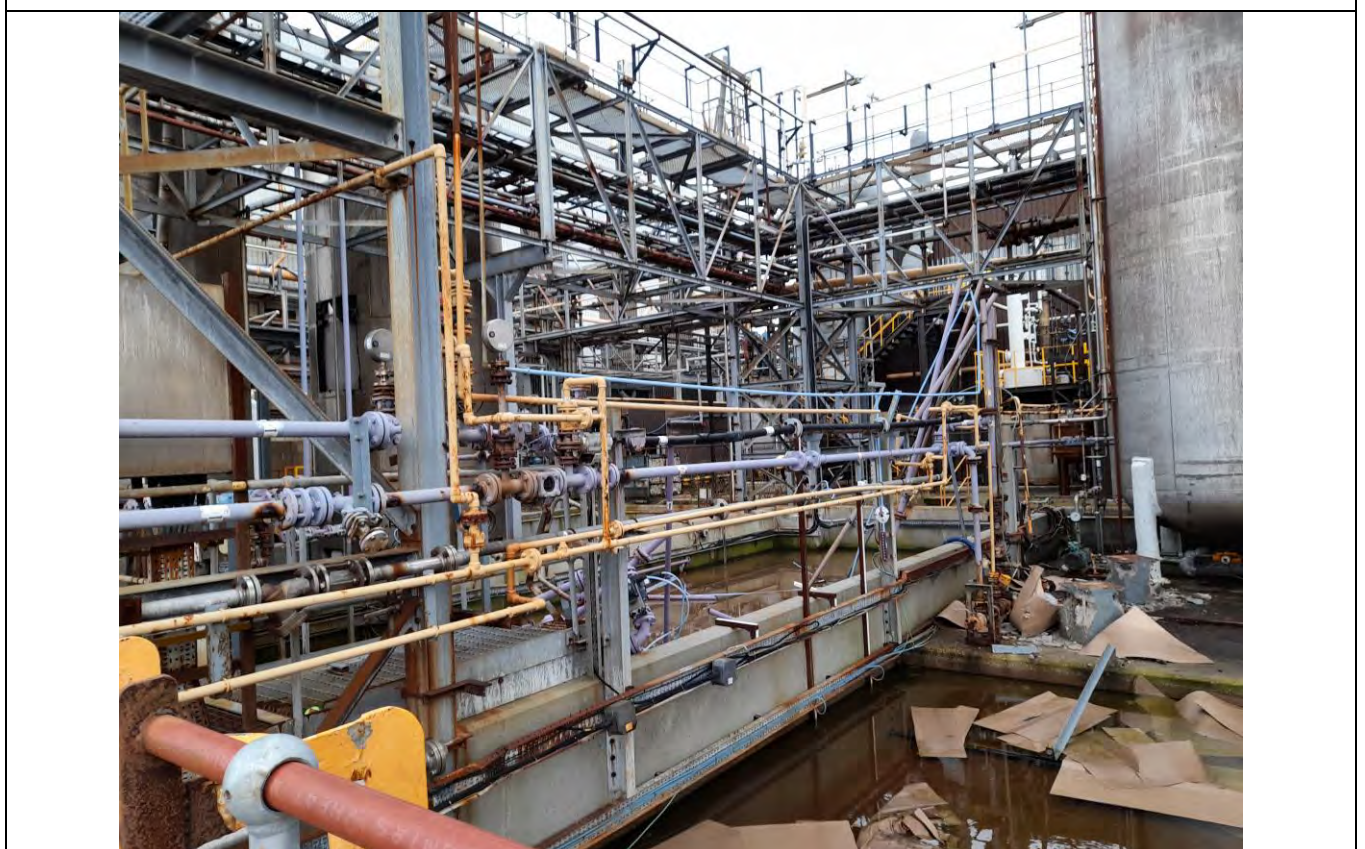
A16.4. View of the bunded tank farm area to the south of the Bonner building
