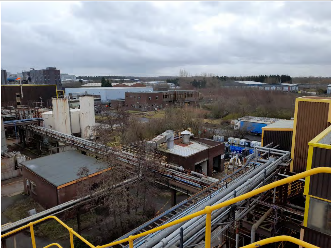
View from the Bonner Building towards the south east, office block visible in the distance
