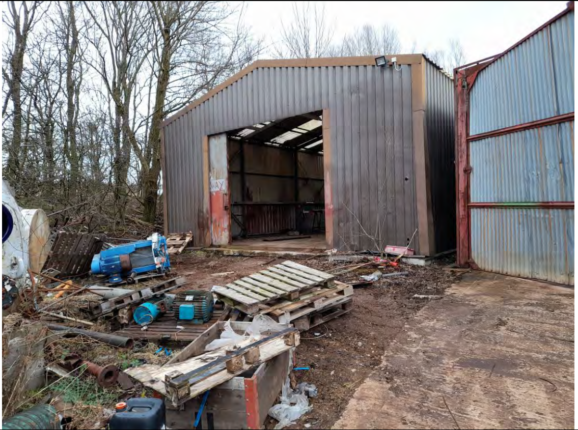
A9.1 View of the workshop sheds
