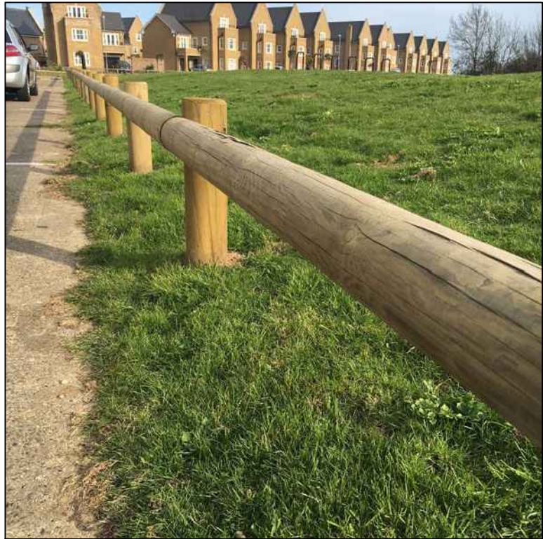
Timber Knee rail to define LAP Boundary 600mm above ground.
