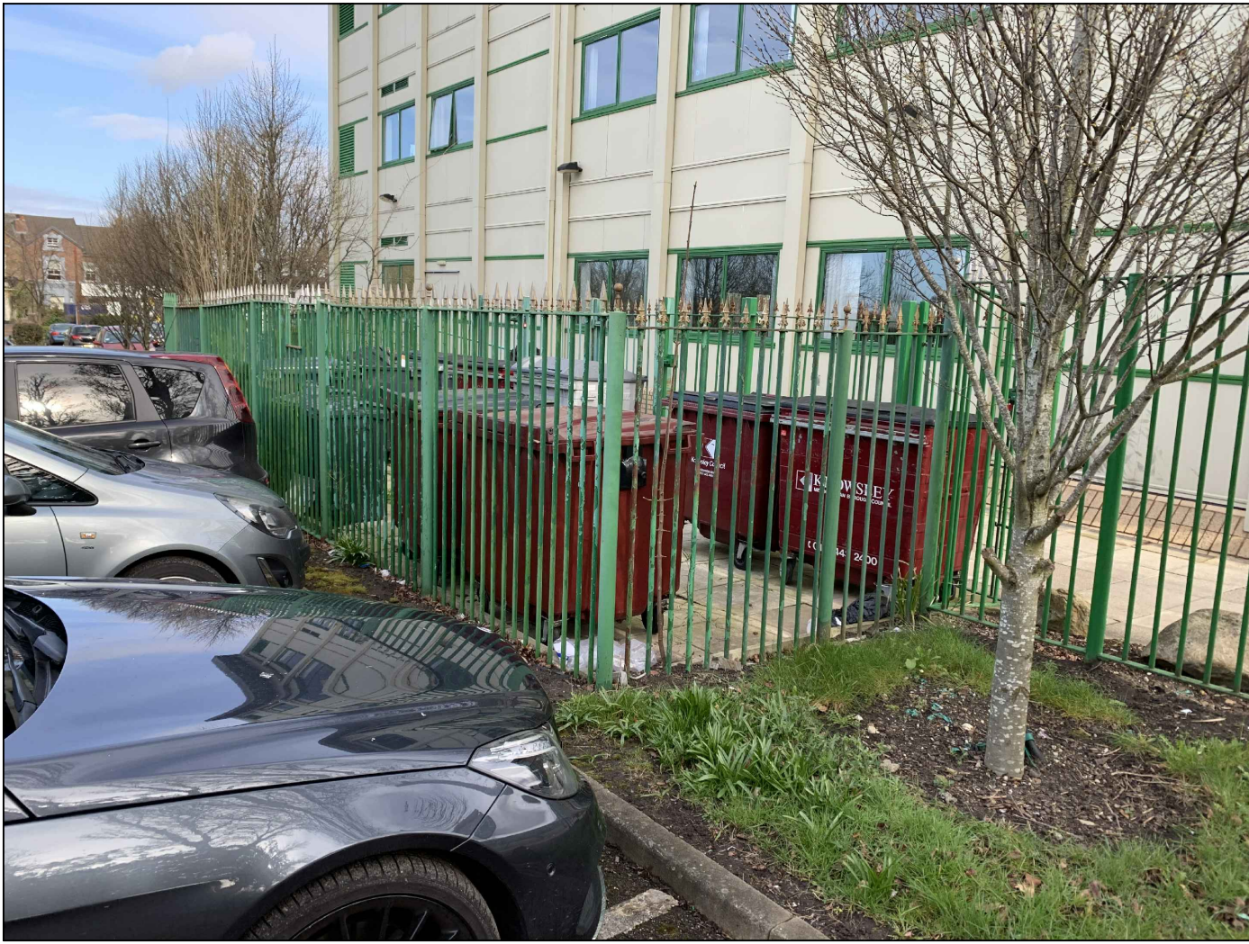
EXISTING SIDE A ELEVATION BIN STORE AREA
