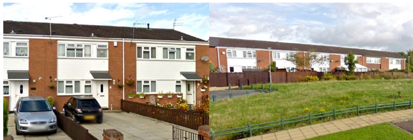
Front driveways and rear private gardens to houses
