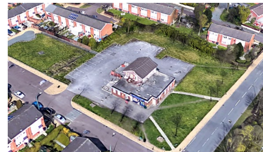
Aerial Photo overlooking the existing shop
