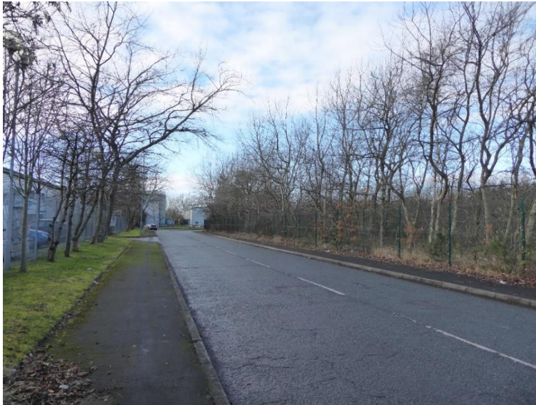
Fig. 10. View west from Villiers Road
