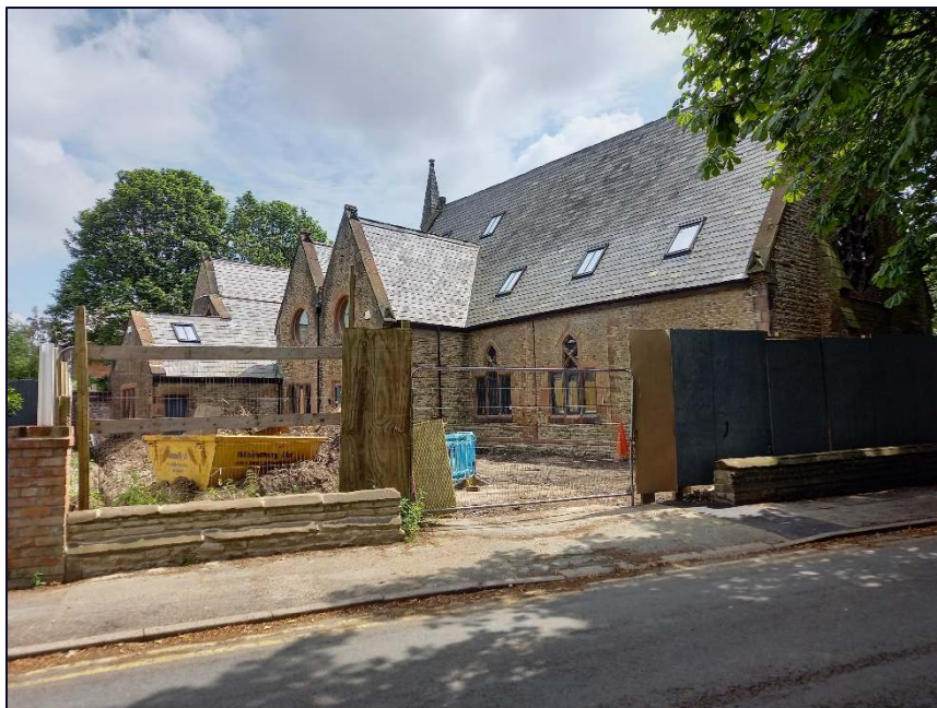
Plate 2: View looking east showing the Grade II listed Park Hall, a former church and school, which is currently under redevelopment (as of July 2021)
