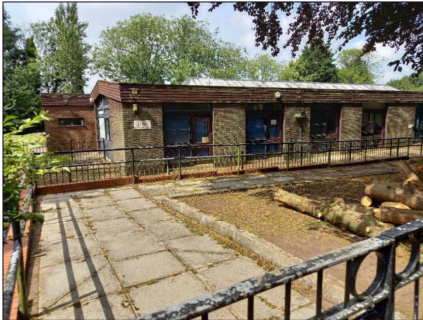
Plate 7: Prospect House, west side of Huyton Church Road
