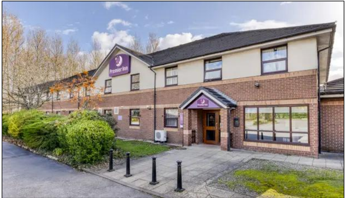
Figure 1 Premier Inn Liverpool (Tarbock) Hotel (Source. Premier Inn)
