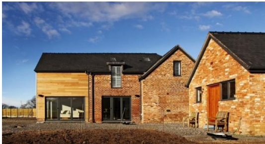
Example of Timber extension to brick building with Aluminium windows.
